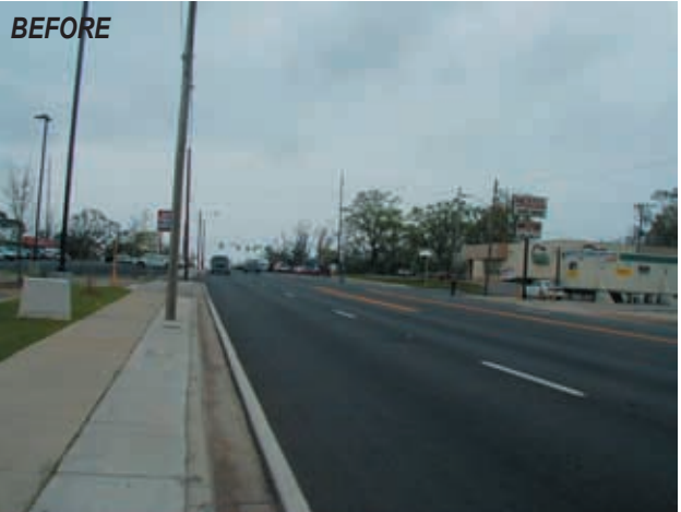
Existing Conditions: Pace Boulevard
