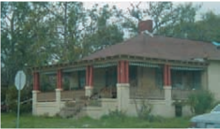
Vernacular residential architecture: Chase Street
