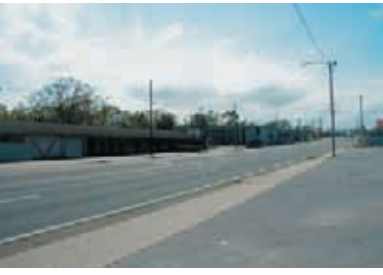
Vacant Commercial Structure: Cervantes Street
