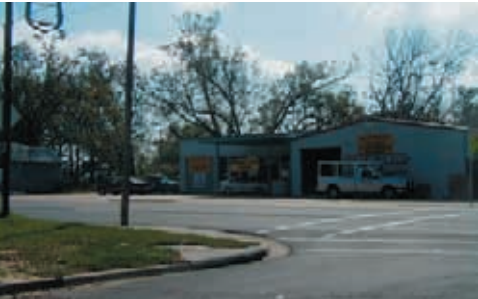
Commercial Establishment: Pace Boulevard
