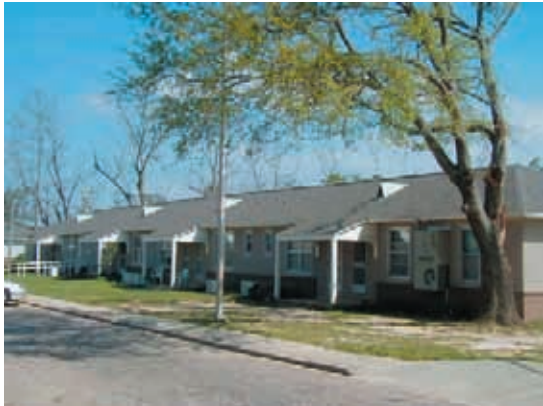
Existing Conditions: Multi-Family Housing, Westside Area
