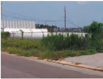
Existing Conditions: ACW Site
