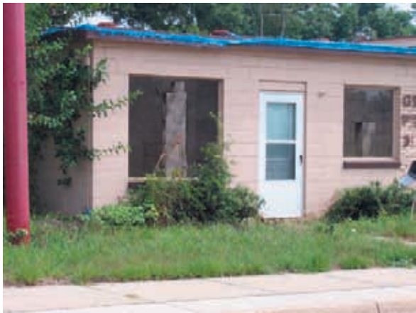
Vacant housing units, Westside Neighborhoods
