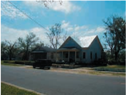
House under repair: A Street
