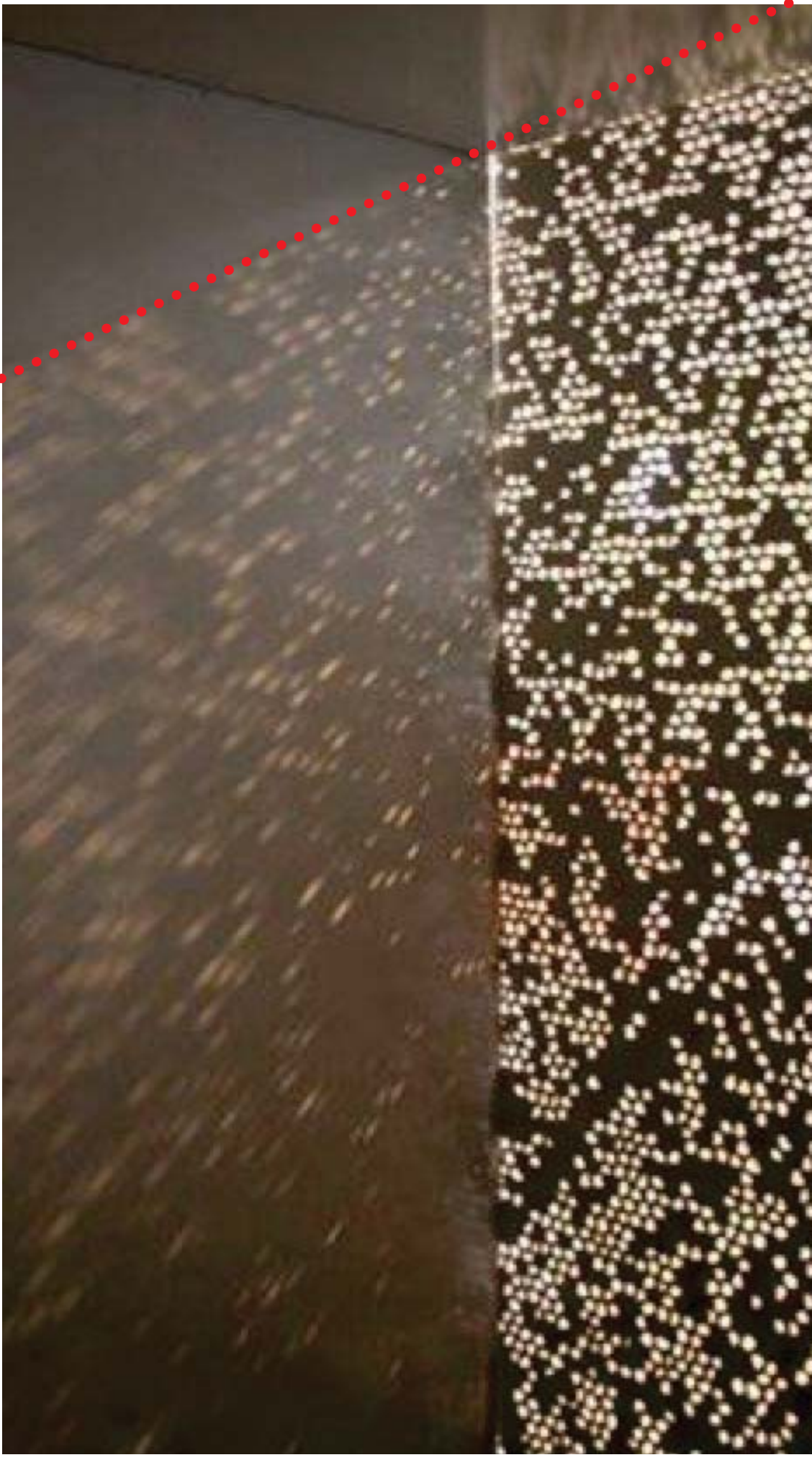
EXAMPLES OF BACKLIT PERFORATED METAL SCREENS
