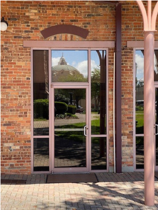
Existing door shown above is to be matched with the new exit door in style, type, material, and color. The hardware is shown above right and the manufacturer is shown to the right.
