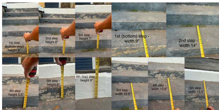
Varying heights and widths of existing concrete steps
