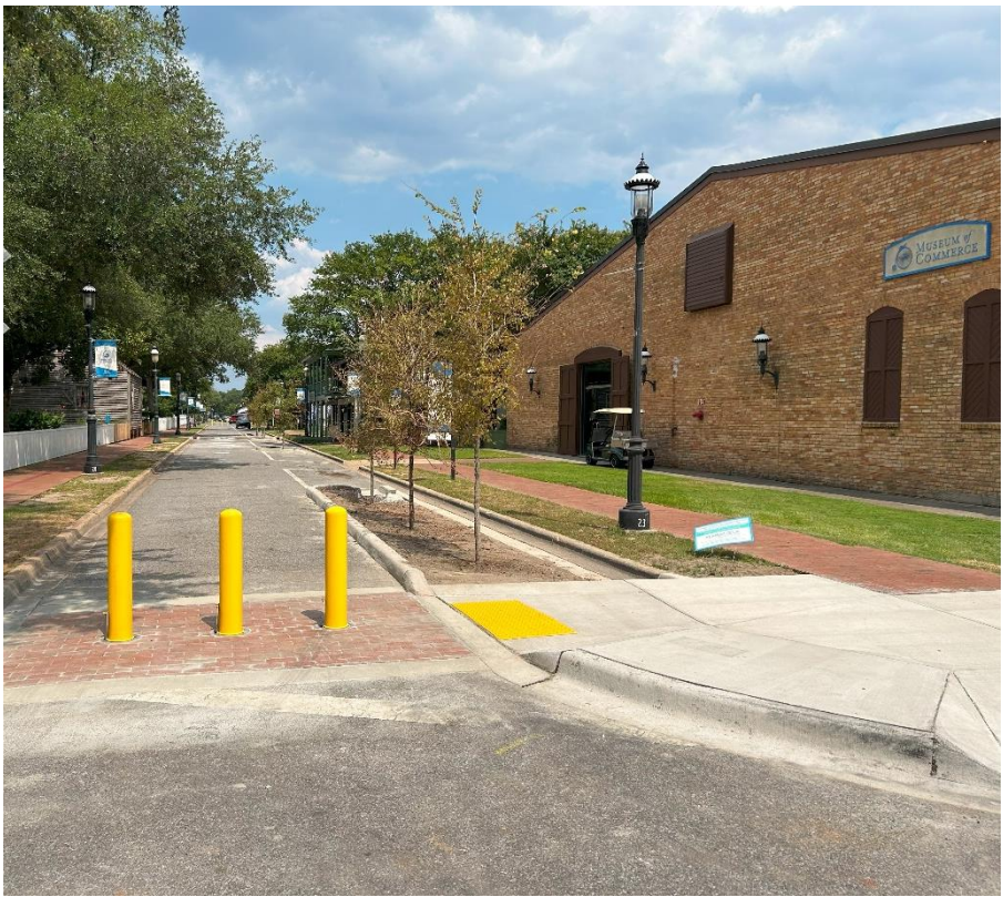
Front of Museum of Commerce with new street improvements
