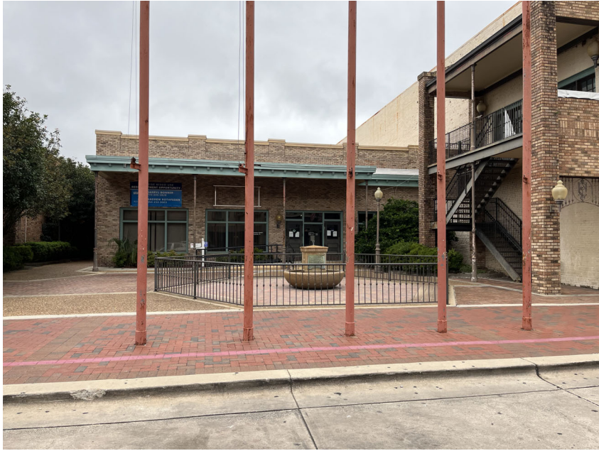
POST OFFICE - FRONT ELEVATION (PALAFOX STREET)
