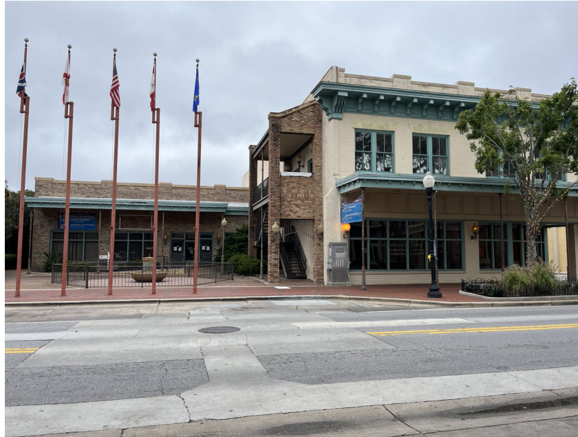
POST OFFICE - FRONT ELEVATION (PALAFOX STREET)
