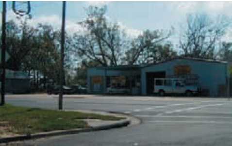
Commercial Establishment: Pace Boulevard
