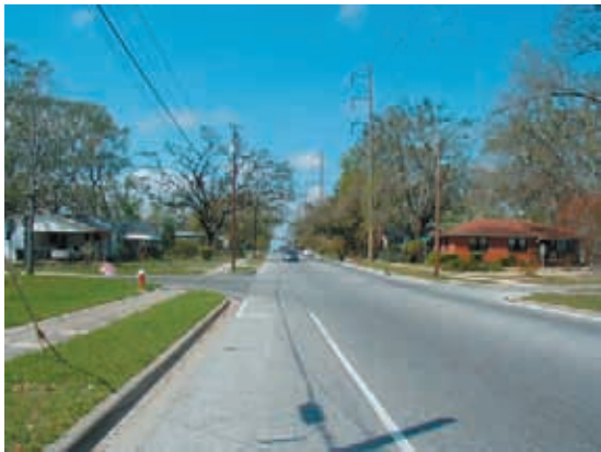
Existing Conditions: Residential Streets
