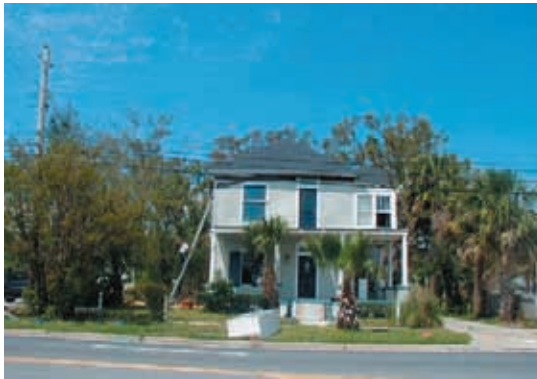
Existing Conditions: Garden Street
