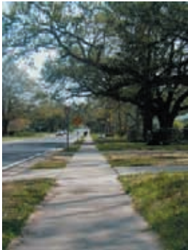
Maintained sidewalks on A Street North
