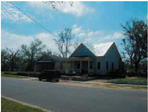
House under repair: A Street
