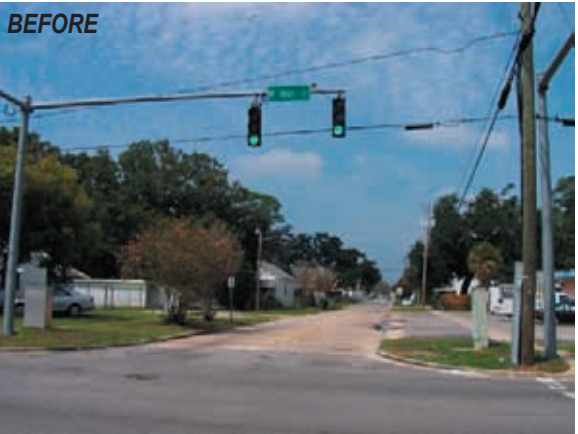
Existing Conditions: Main Street and “E” Street looking north on “E” Street
