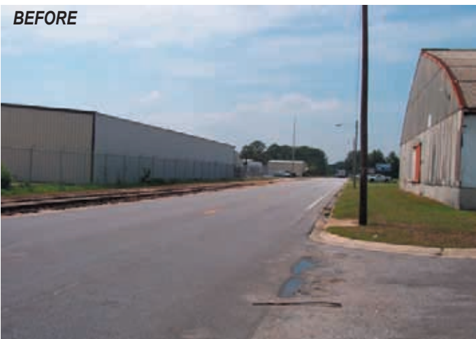
Existing Conditions: Main Street looking east
