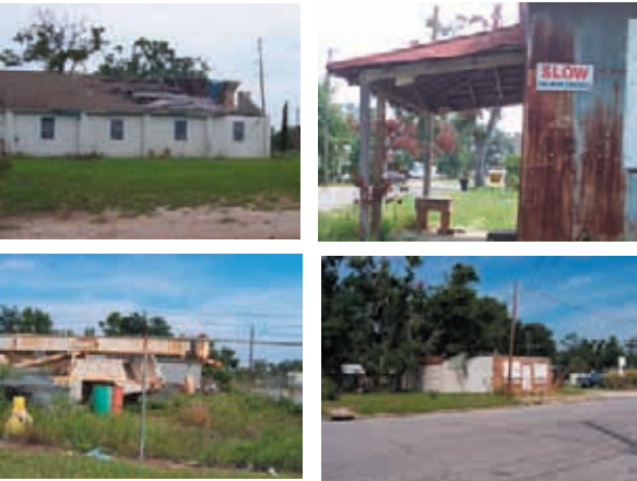
Deteriorating Site Conditions, Westside Neighborhoods Commercial Properties
