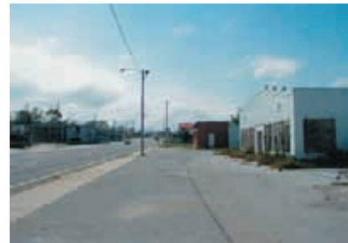
Vacant Commercial Structures: Cervantes Street
