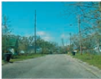
Lack of Sidewalks: M Street
