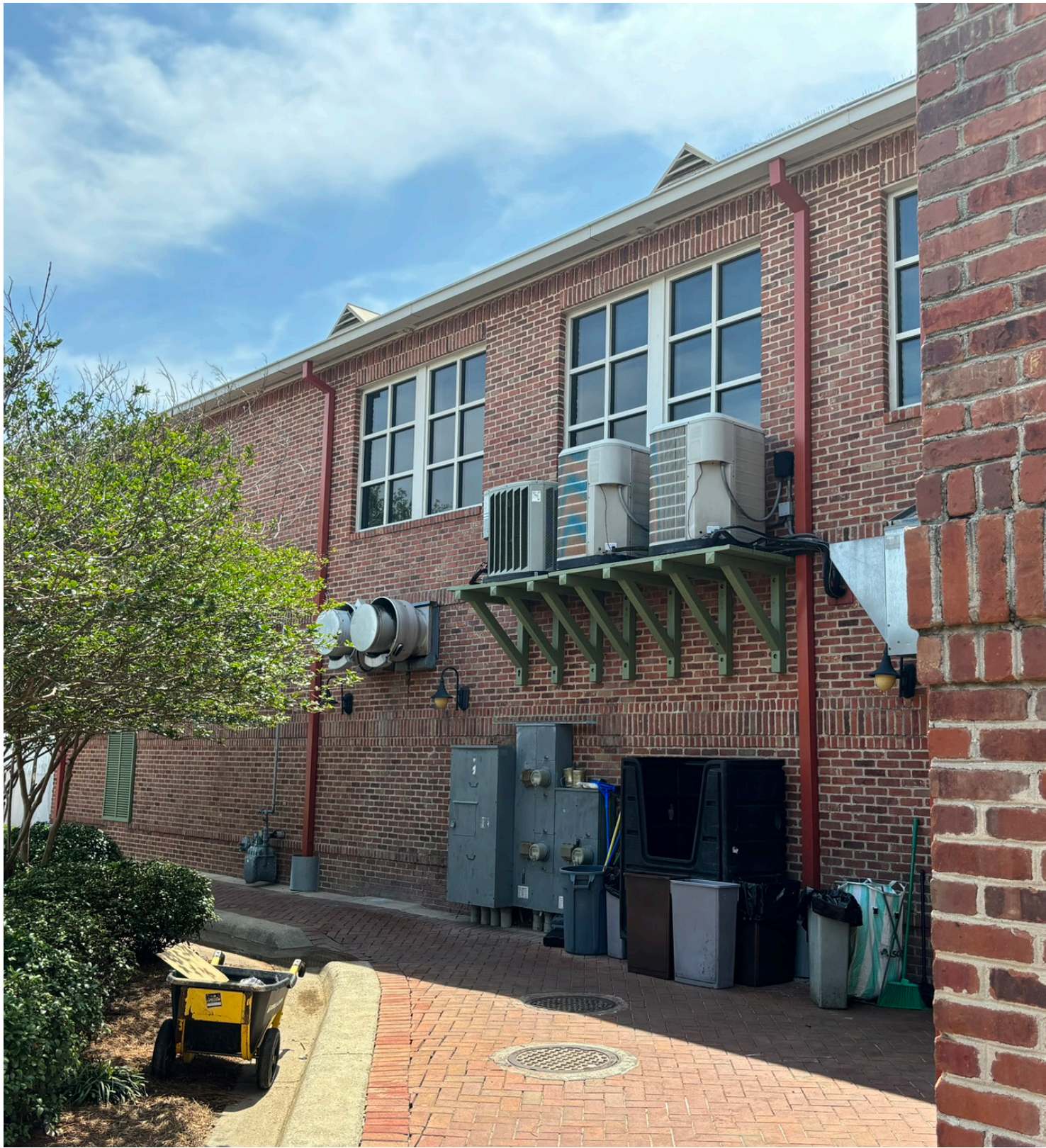
Current mechanical equipment conditions
