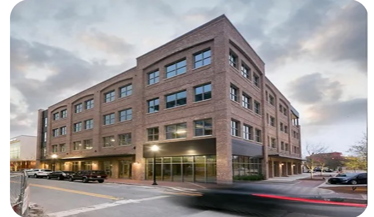
Urban Core Office Building Development Manager Completed: 2017
