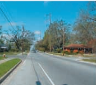
On- street Parking E Street
