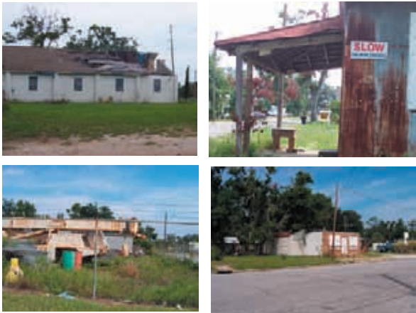
Deteriorating Site Conditions, Westside Neighborhoods Commercial Properties
