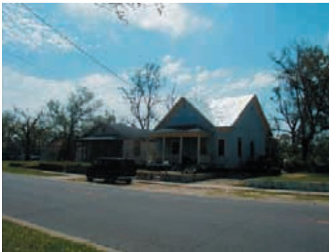
House under repair: A Street
