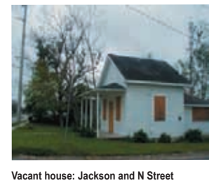
Vacant house: Jackson and N Street
