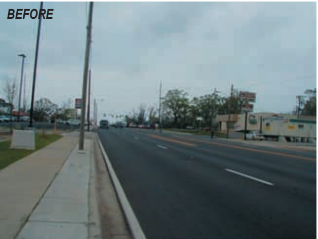
Existing Conditions: Pace Boulevard
