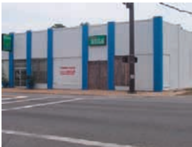
Vacant and Boarded Structure along Pace Boulevard
