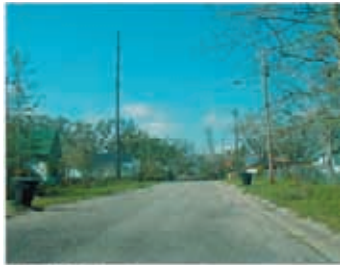
Lack of Sidewalks: M Street
