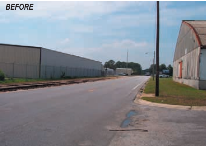
Existing Conditions: Main Street looking east
