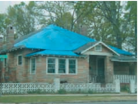
Stone clad house: Chase Street
