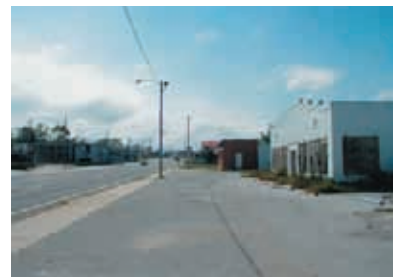
Vacant Commercial Structures: Cervantes Street
