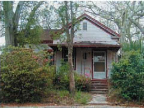
Residential House: J Street
