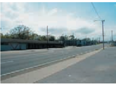
Vacant Commercial Structure: Cervantes Street
