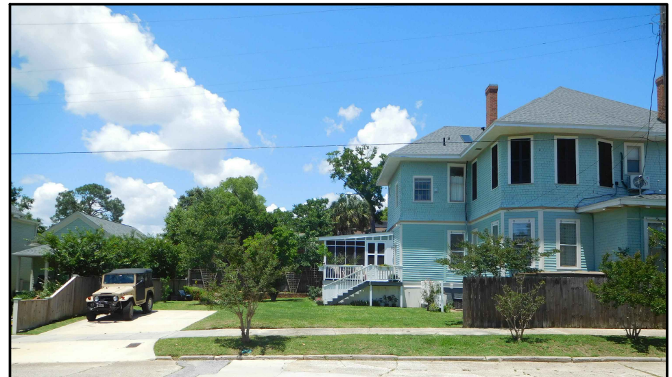
3 EXISTING CONDITIONS PHOTO 3-A1 Photo of side elevation taken from side street (Strong St.). Porch, deck and steps leading up to it will be demolished to make way for new structure.
