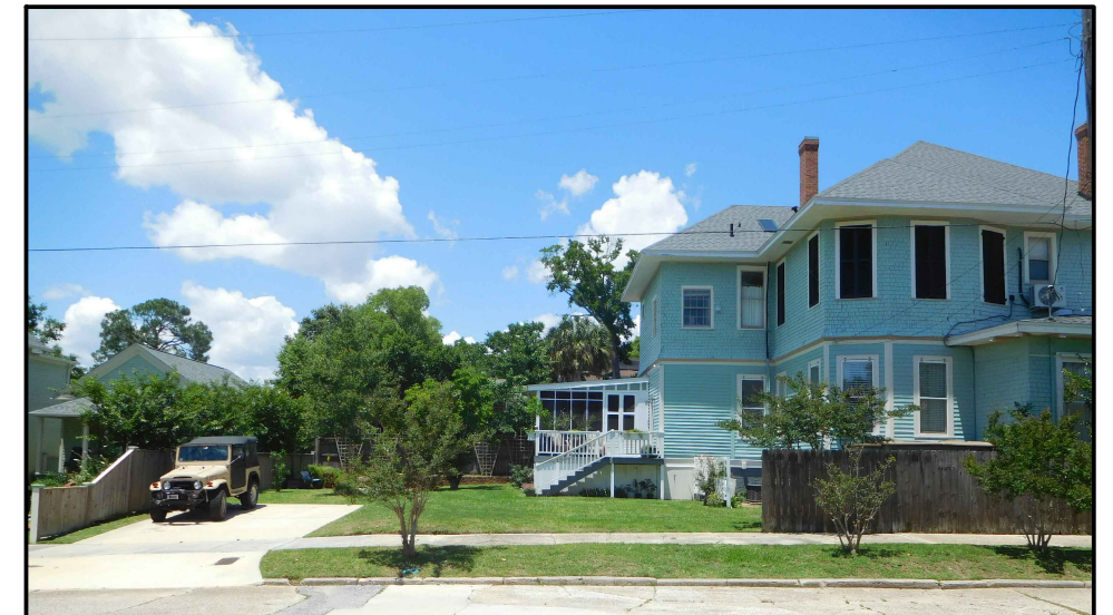
3 A1 EXISTING CONDITIONS PHOTO 3-A1 Photo of side elevation taken from side street (Strong St.). Porch, deck and steps leading up to it will be demolished to make way for new structure.
