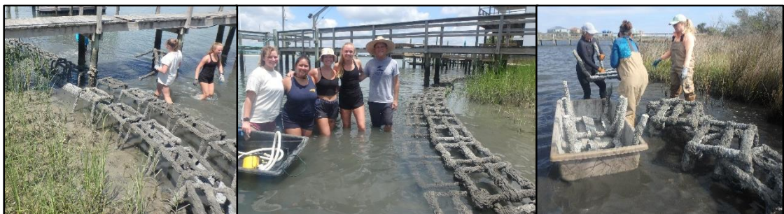
Figure 4. Volunteers constructing Table reefs – Topsail Beach, NC.
