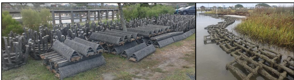
Figure 5. Staged materials and newly installed reef – Surf City, NC . Page 39 of 241
