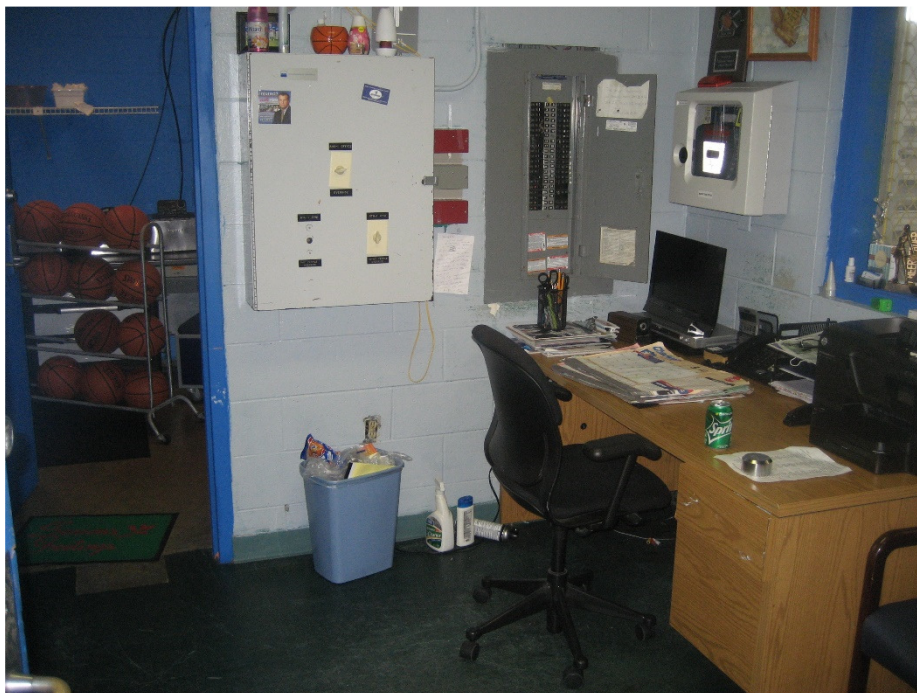
Interior View of Office in Subject Building
