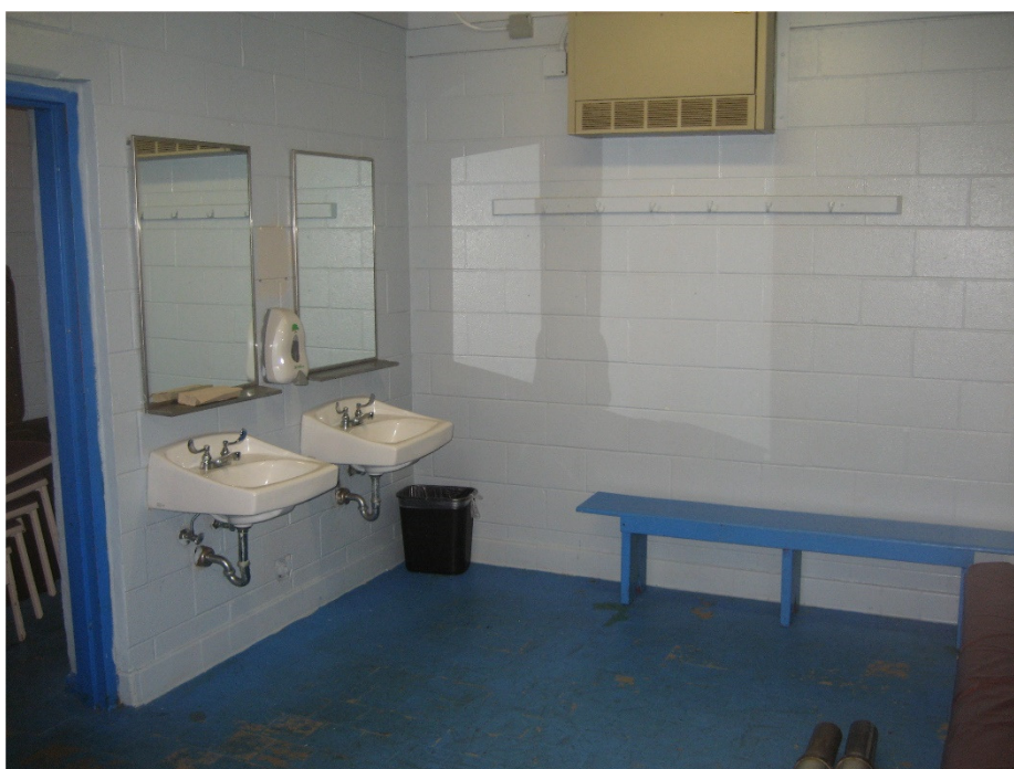
View of Typical Restroom in Subject Building
