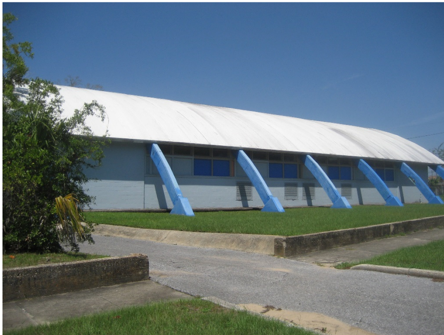
Side View of Subject Building
