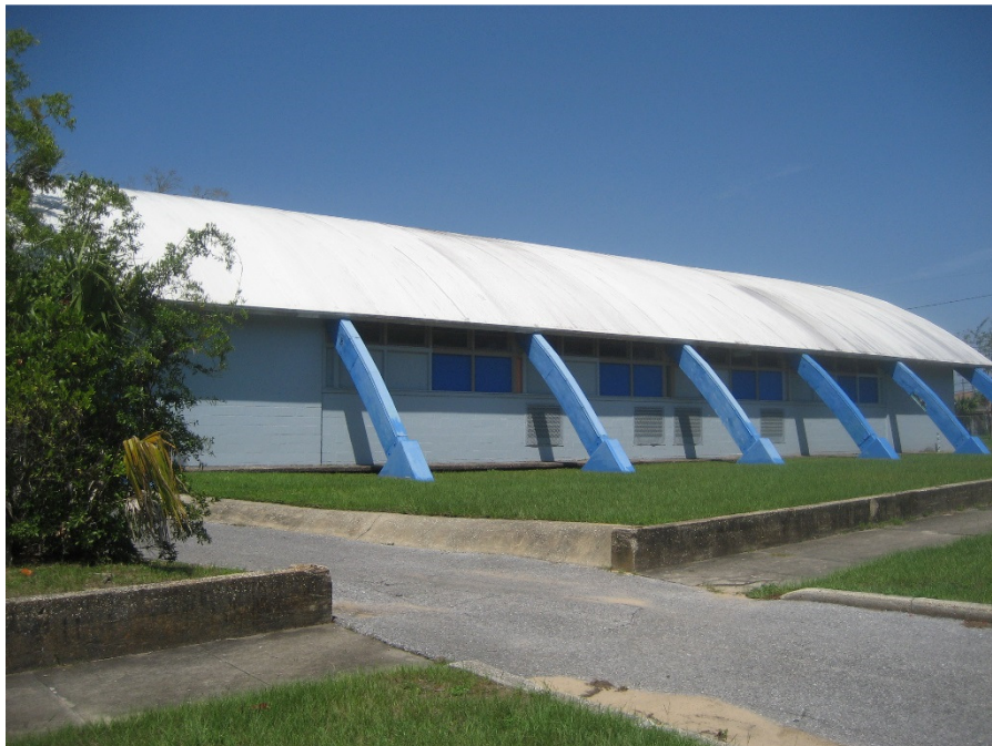
Side View of Subject Building
