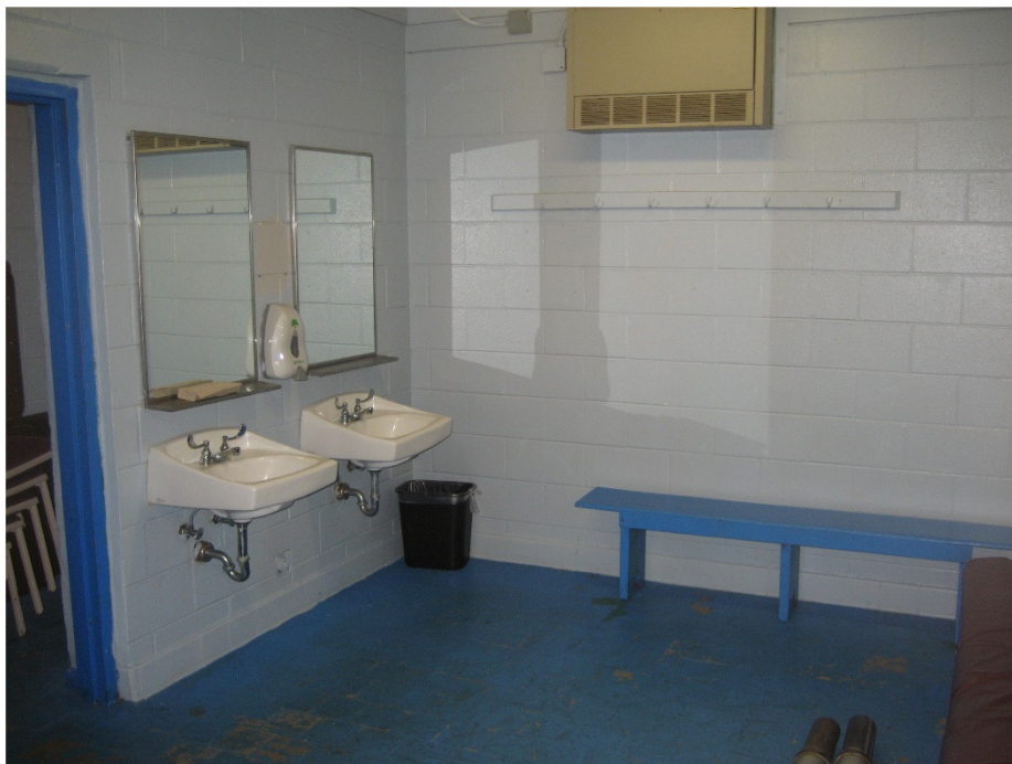
View of Typical Restroom in Subject Building
