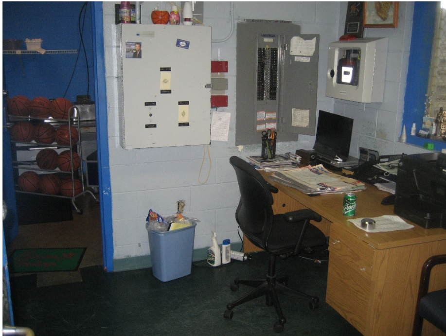
Interior View of Office in Subject Building
