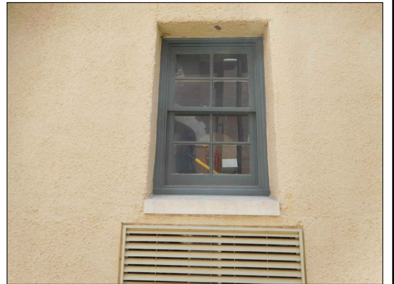
Close up view of Location B window at West Elevation (existing).
