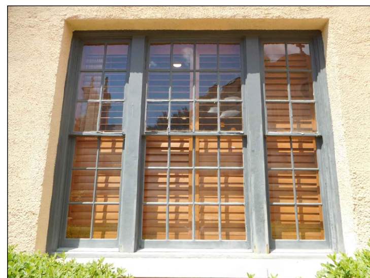
Close up view of typical Location C window at East Elevation (existing).
