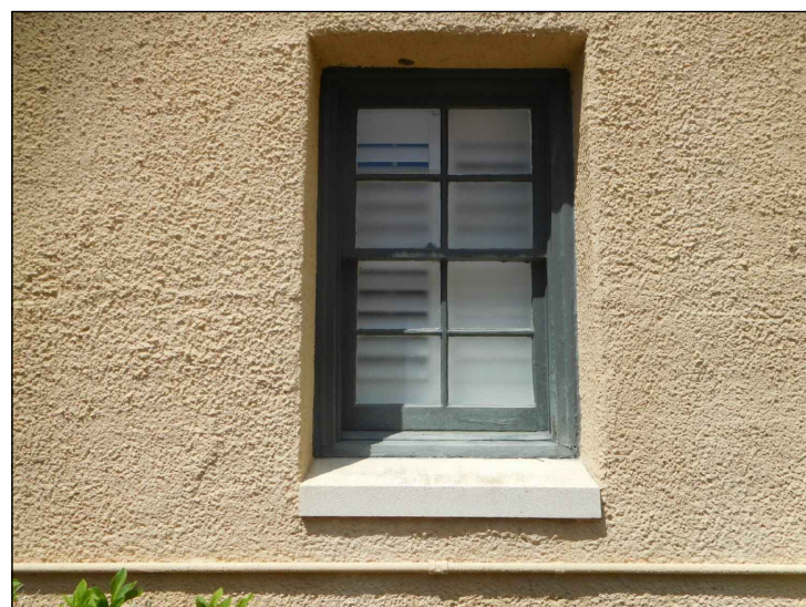
Close up view of Location B window at East Elevation (existing).
