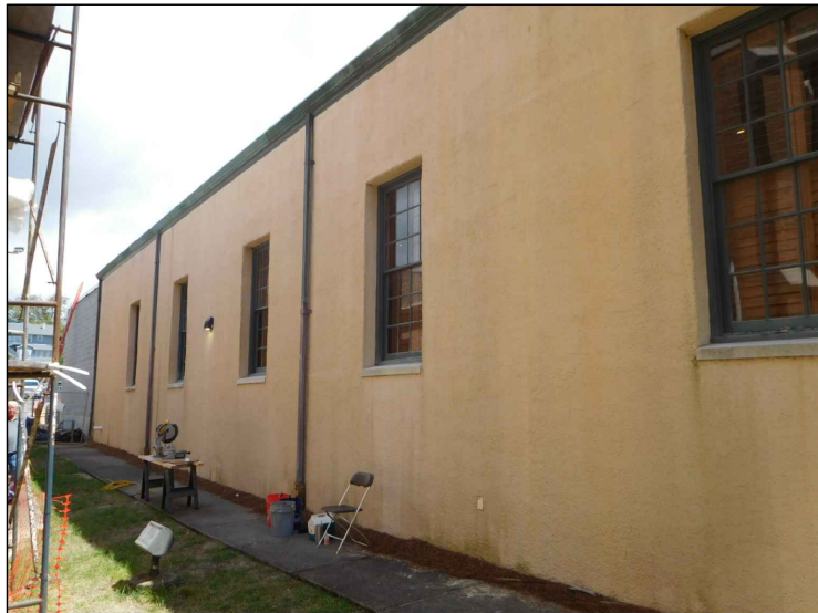
West Elevation Showing the five Location A windows as they currently exist.
