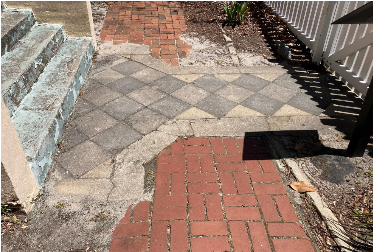
Photo 9: Front of the Lear House. The black and white pavers with a concrete edging will remain and the two different brick types will be replaced.
