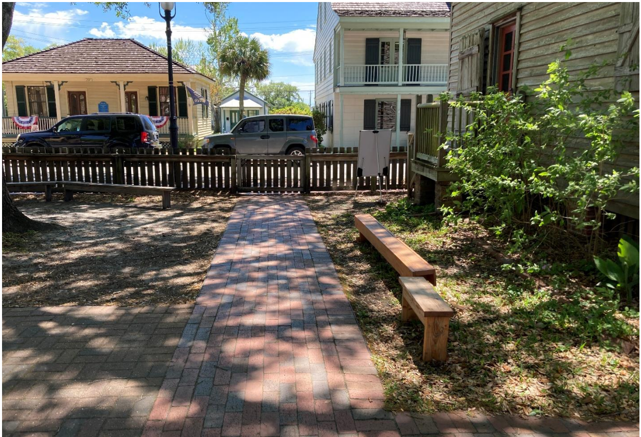
Photo 2: Existing entrance looking south. Note two different brick types: wire cut clay brick (Glen Gery, Full Range 2-1) and concrete paver.
