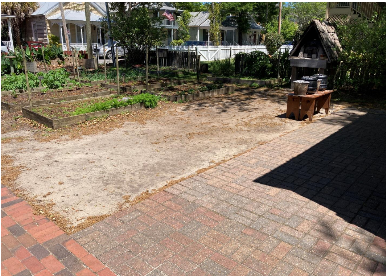
Photo 6: North side of Kitchen House where school tours are held. Constant traffic has killed the grass. Note the two different brick types: wire cut clay brick (Glen Gery, Full Range 2-1) and concrete paver.
