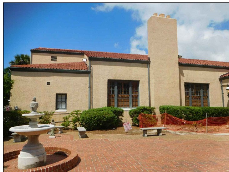
East Elevation Showing the two Location C windows and the one Location B window as they currently exist.
