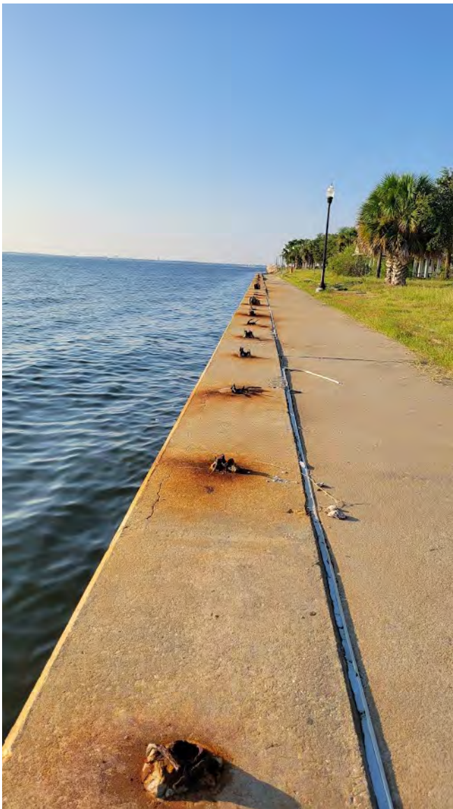
Photo 7: Damaged handrail
