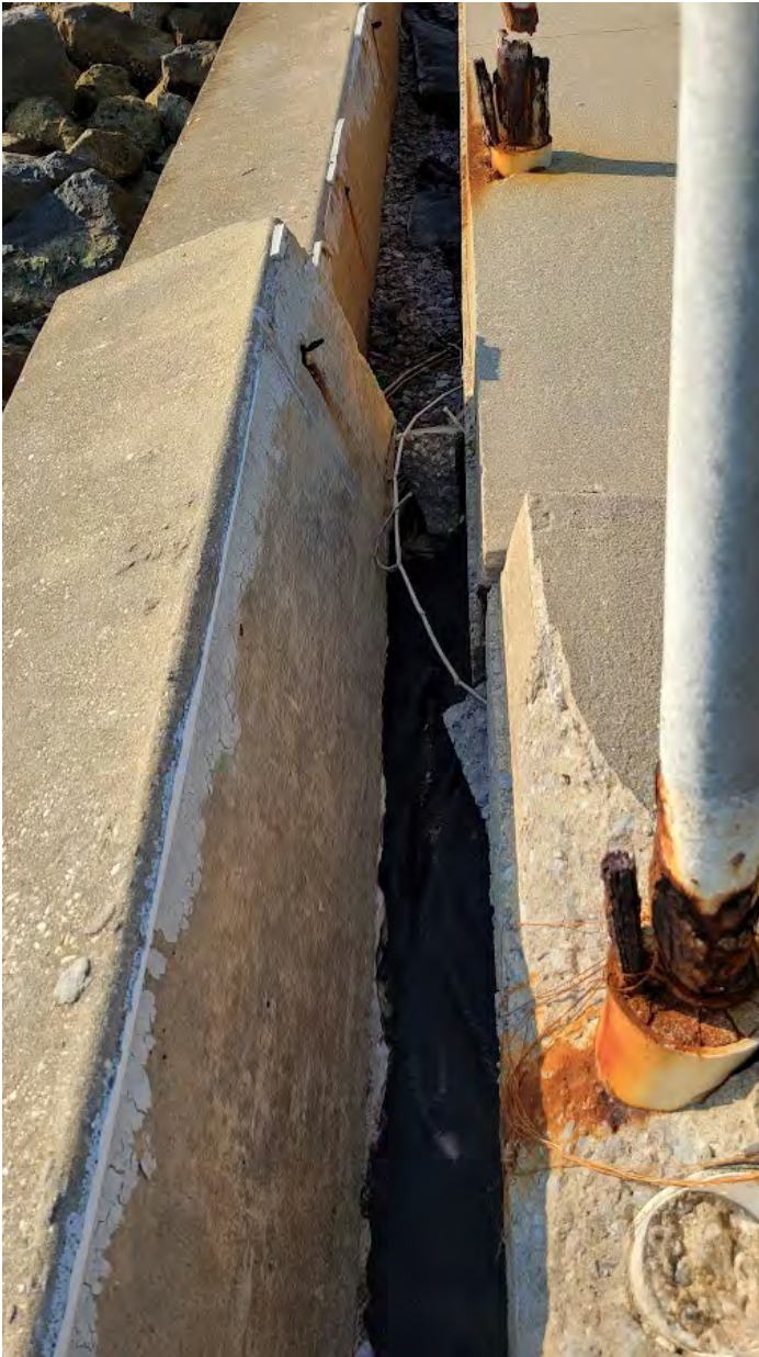
Photos 10 & 11: Undermined ground-supported beam at revetment; damaged sidewalk/handrail
