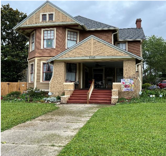
SOUTH SIDE OF HOUSE
