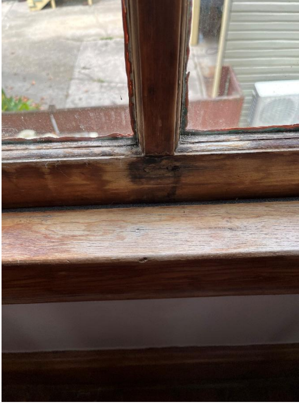
WATER INTRUSION CAUSING DAMAGE TO WINDOW TRIM AND BASE BOARDS
