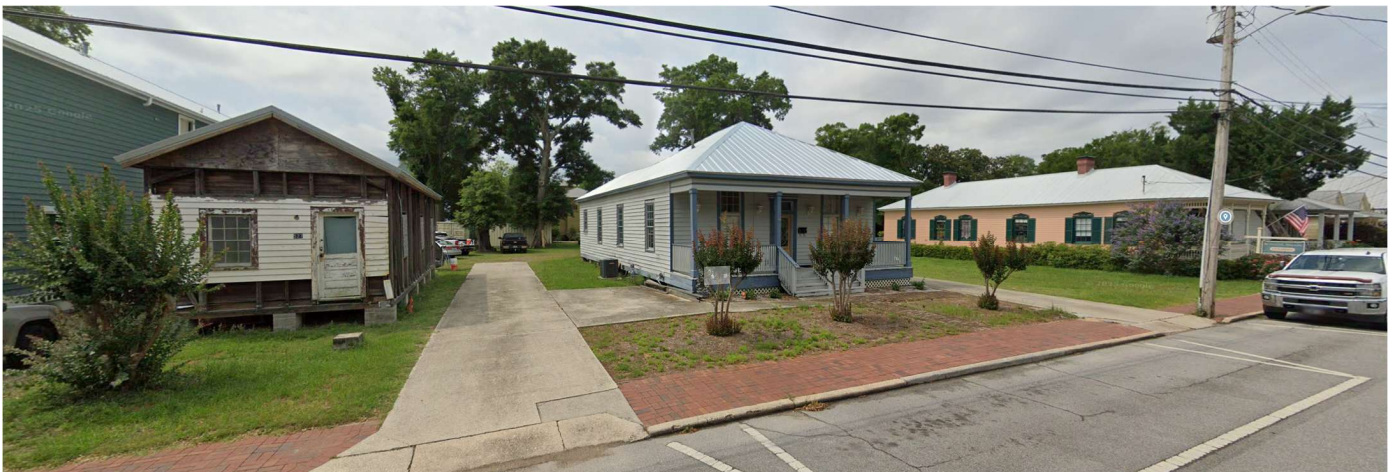
View from E Government St looking East
