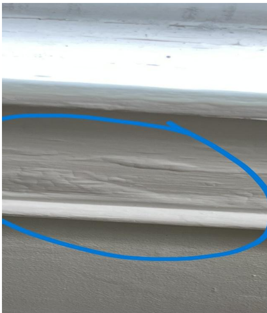
WATER INTRUSION CAUSING DAMAGE TO WINDOW TRIM AND BASE BOARDS
