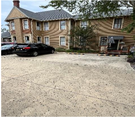
EAST SIDE OF HOUSE
