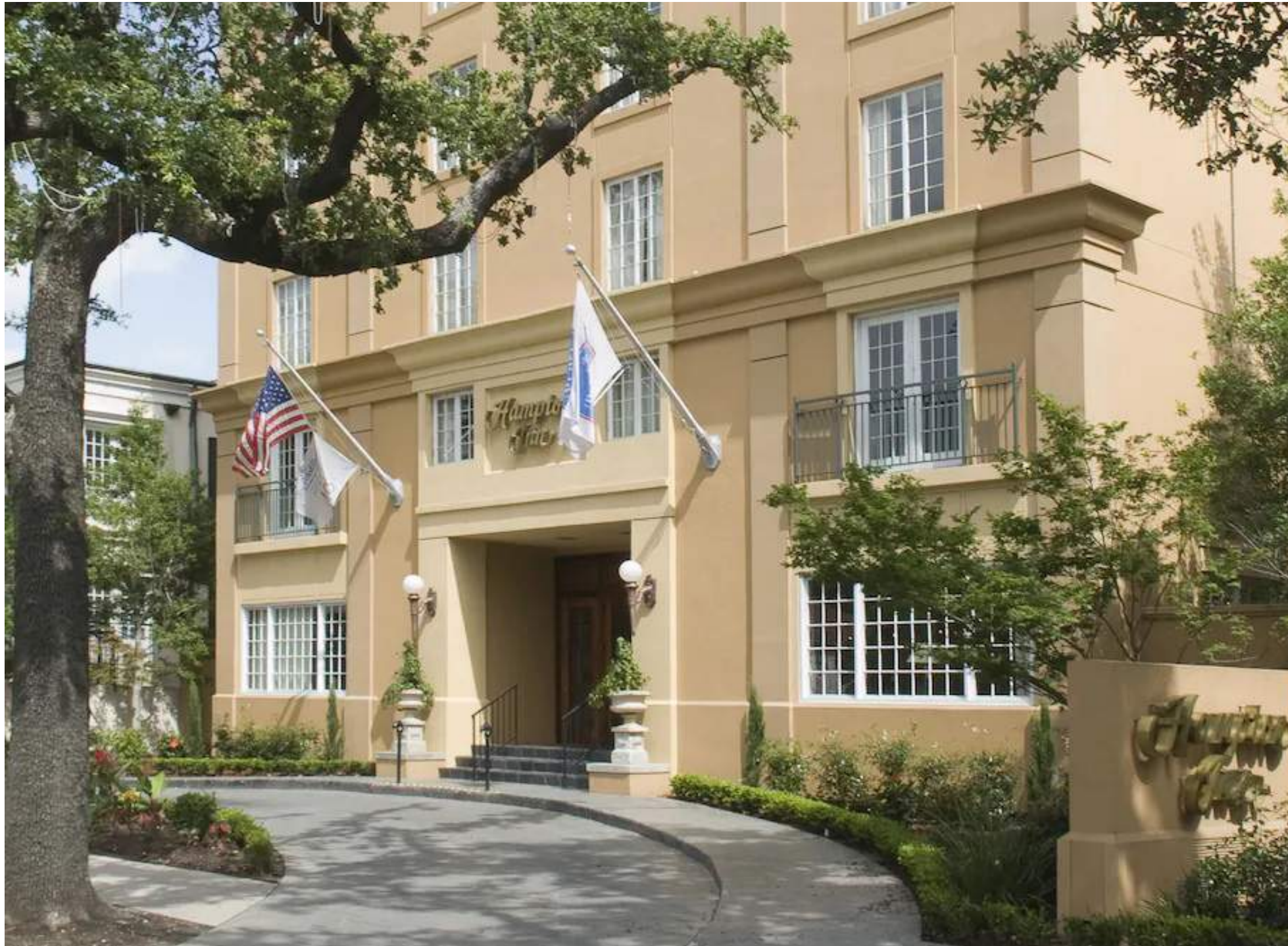
AC Hotel Pensacola
