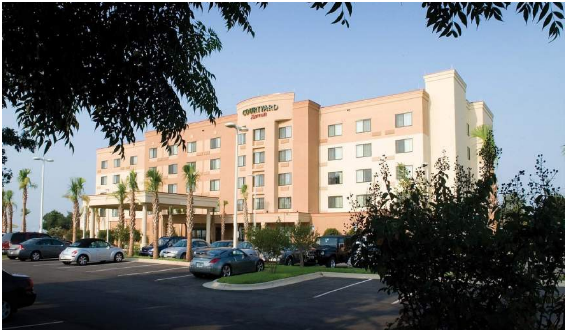
Courtyard by Marriott - Downtown - Pensacola, FL
