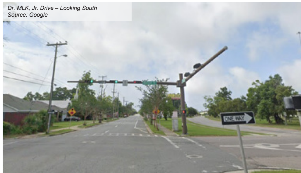
Figure 19 Eastside – Arterial Road
