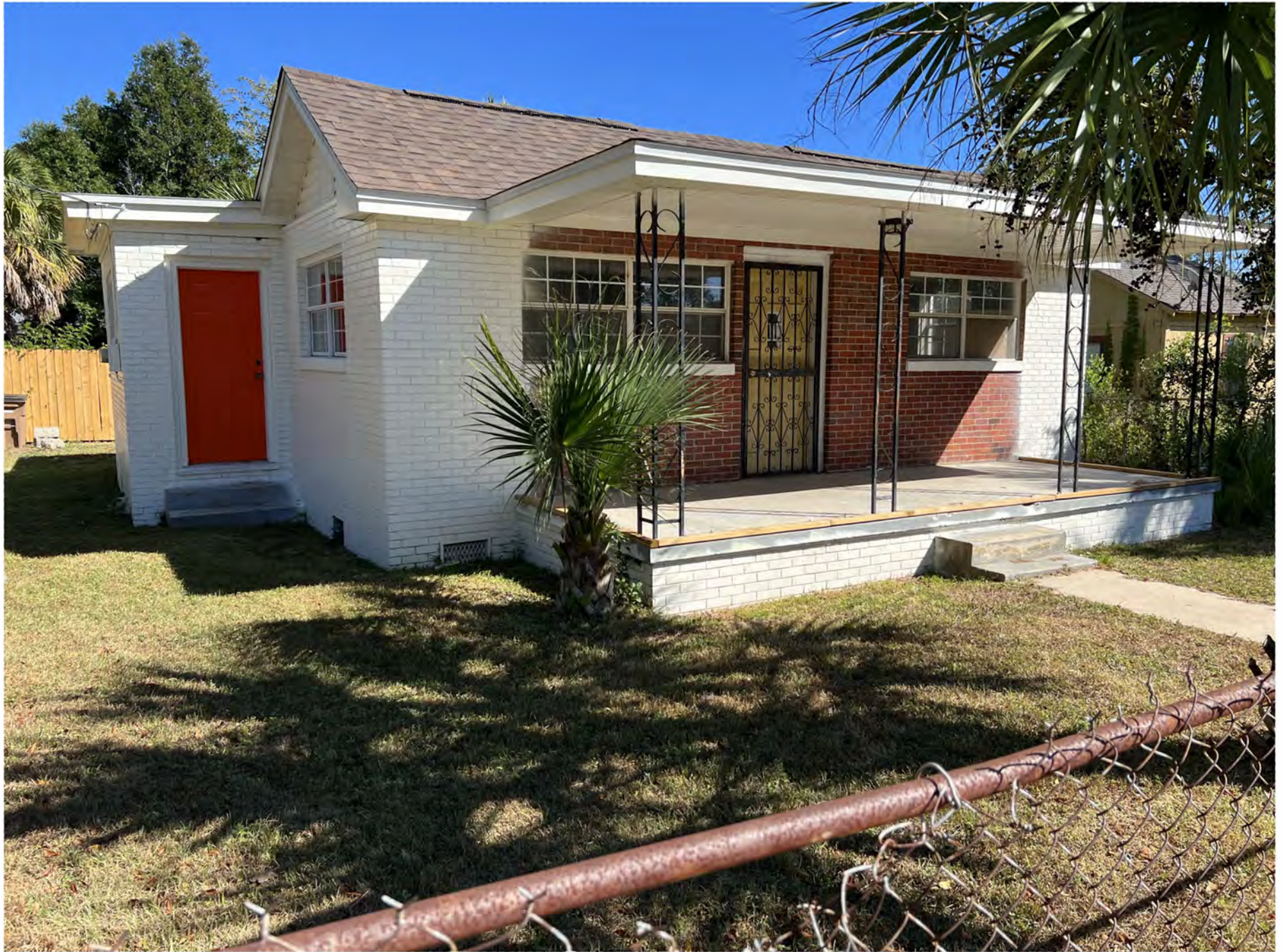
View of 2504 N Davis Hwy., taken from N. Davis Hwy. facing southwest.
