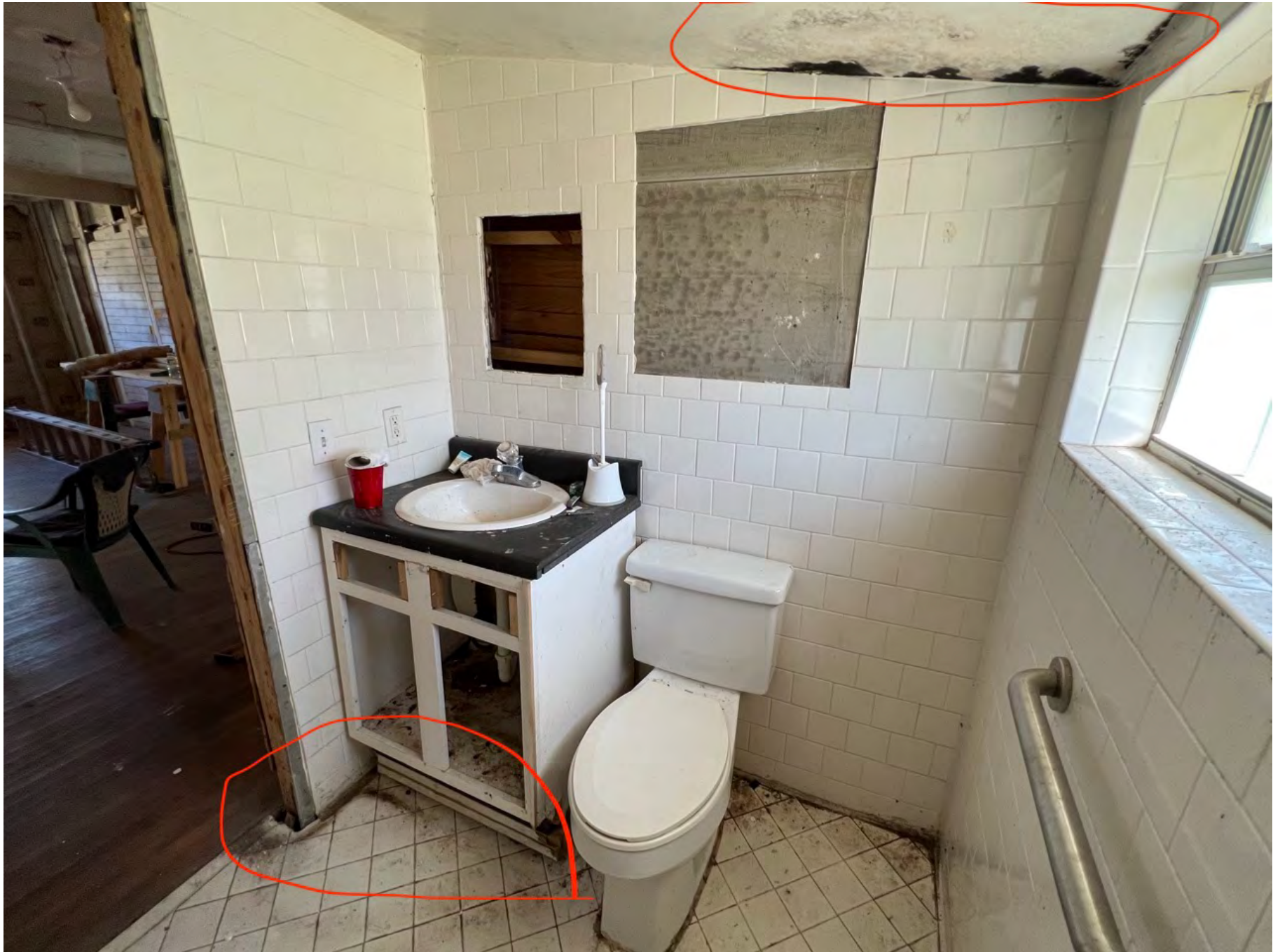
2504 N Davis existing bath
