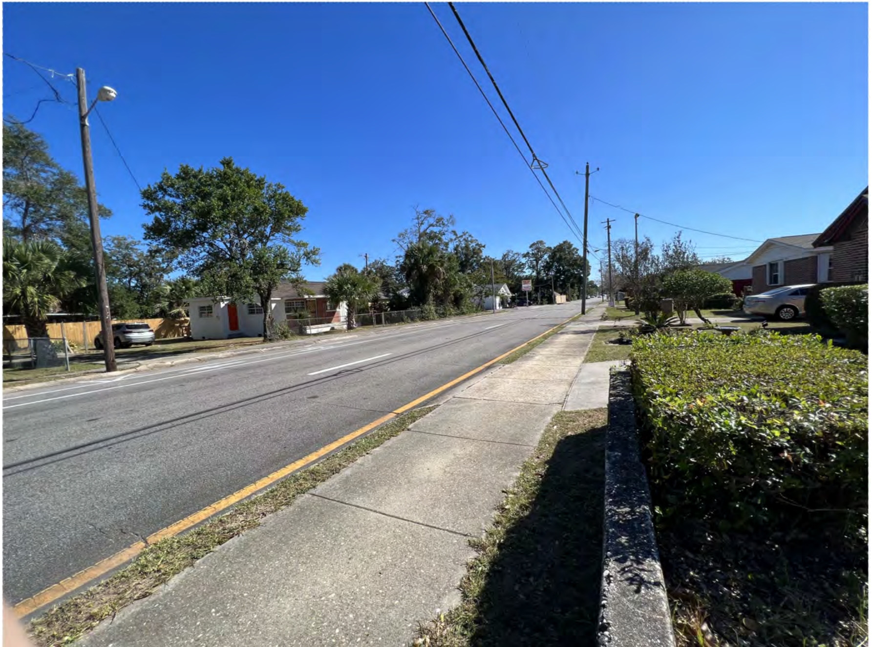
View 2504 N Davis taken from N. Davis Hwy. facing southwest.
