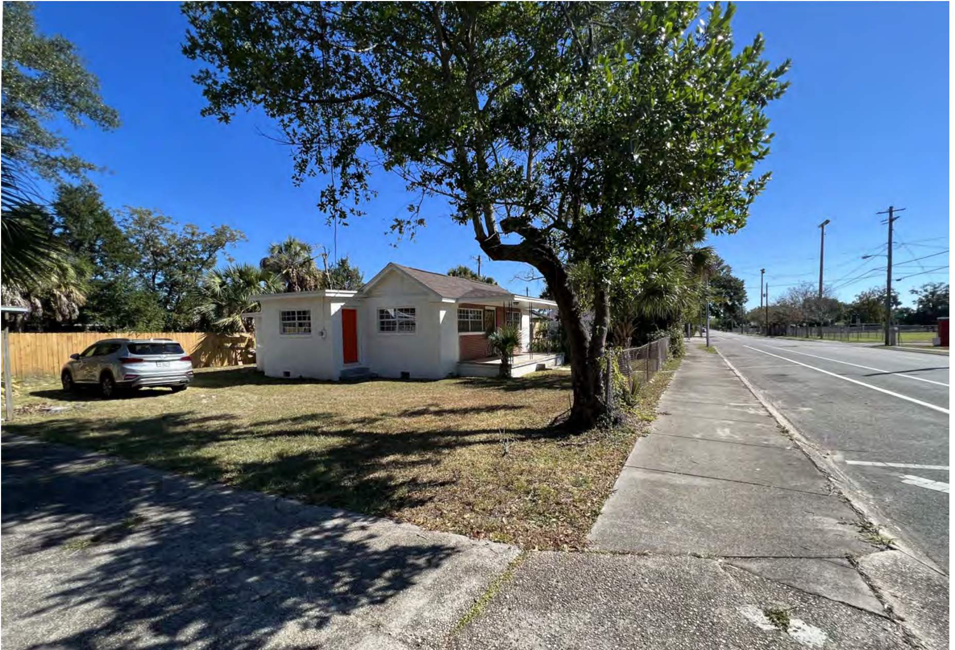
View of 2504 N Davis Hwy., taken from N. Davis Hwy. facing southwest.
