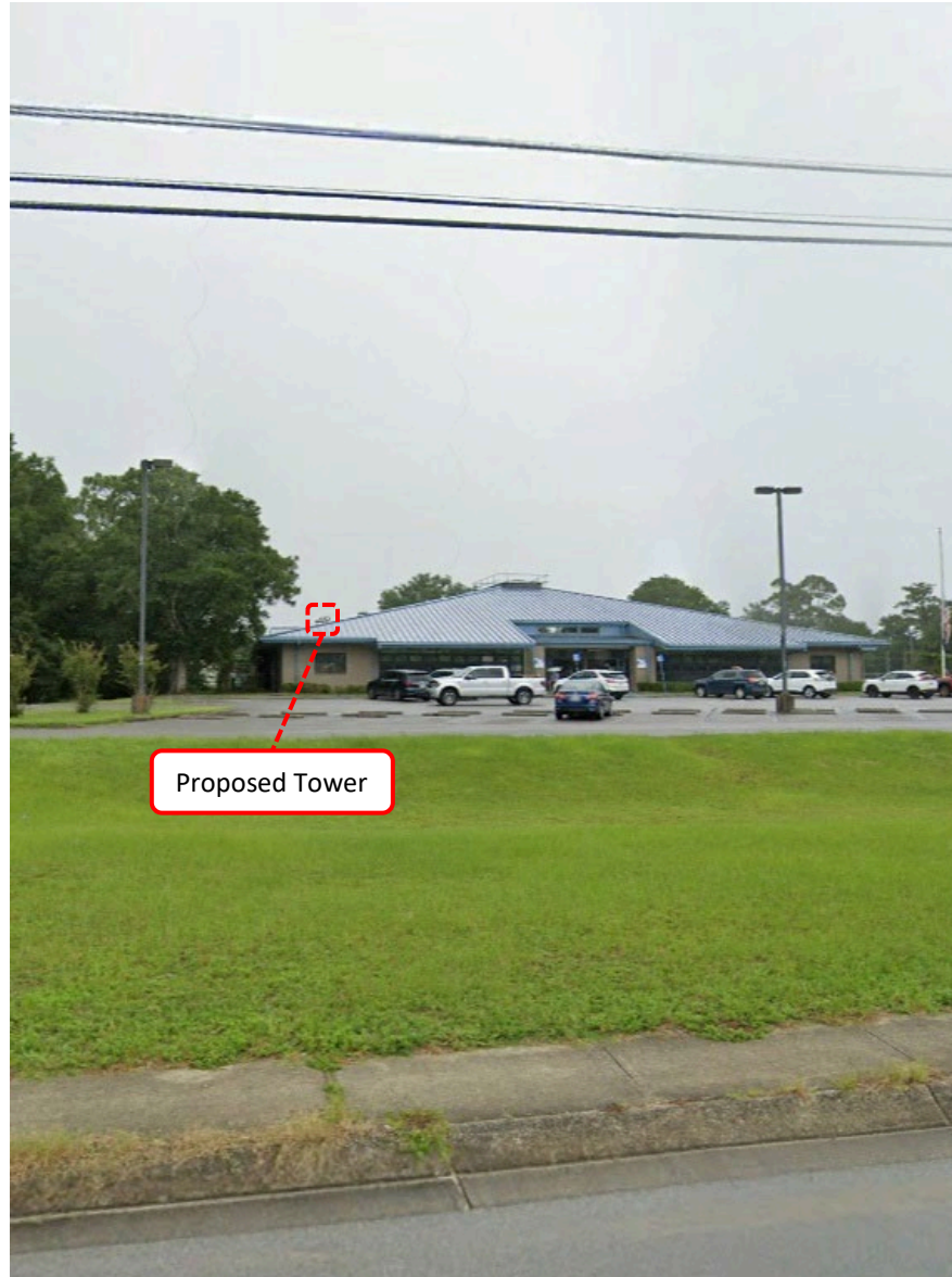
Photo facing East toward the proposed tower location from Tippin Ave
