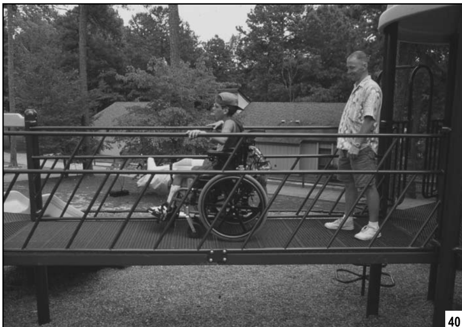
This photo illustrates an elevated accessible route:
