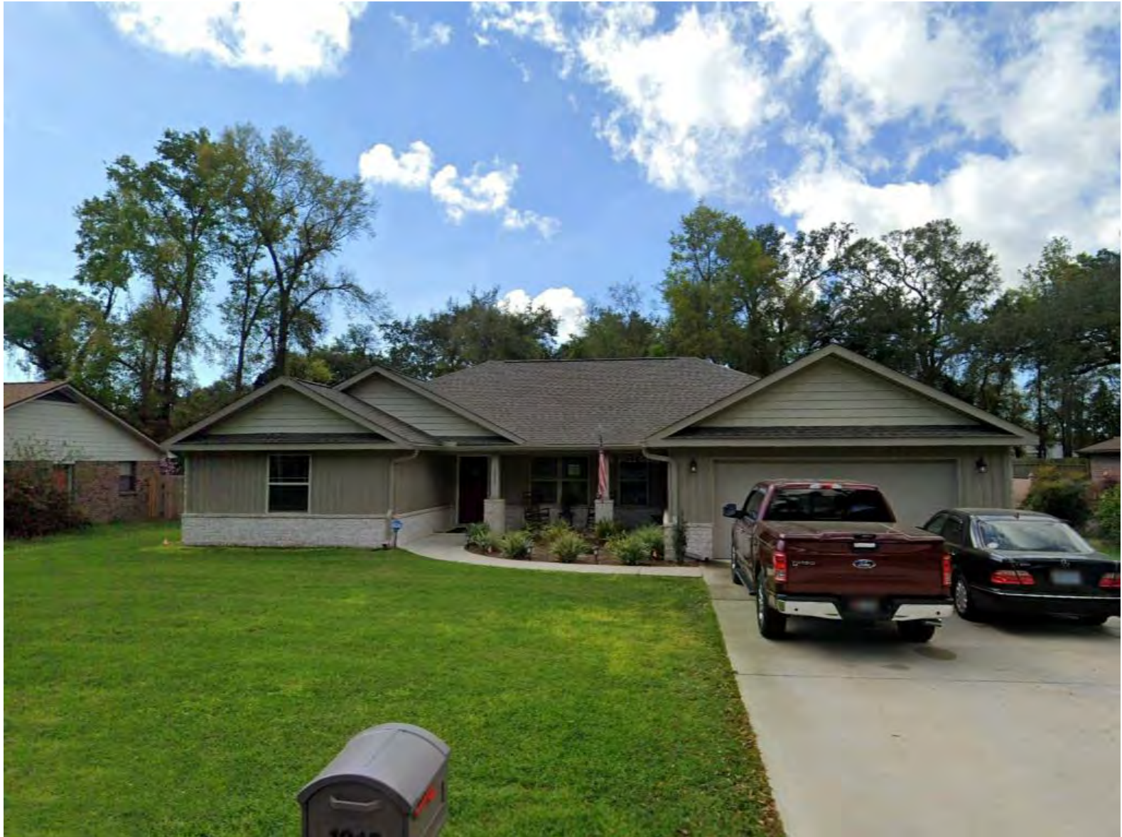
Photo facing South toward the proposed tower locations from Tamara Dr
