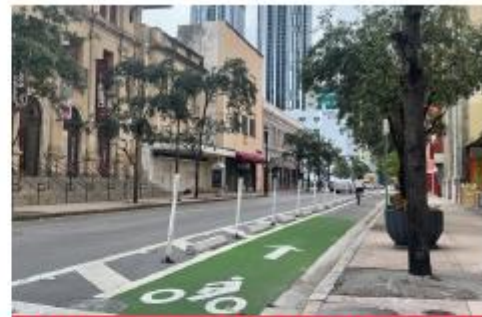
Separated Bicycle Lane with Bollards
