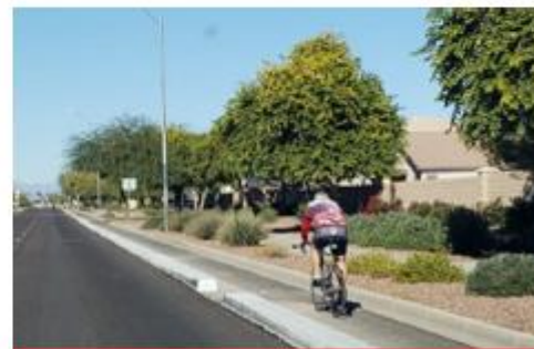
Median Bicycle Lane with Concrete Buffer
