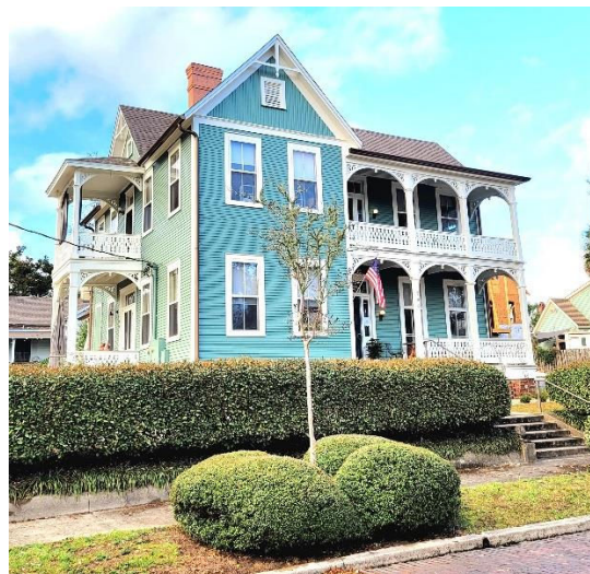
Views of Existing Front
