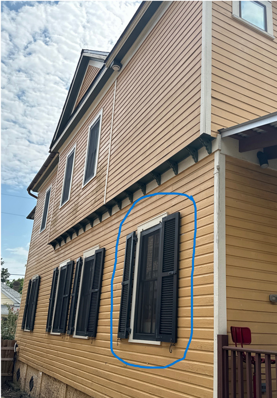
Window to be covered with shutters
