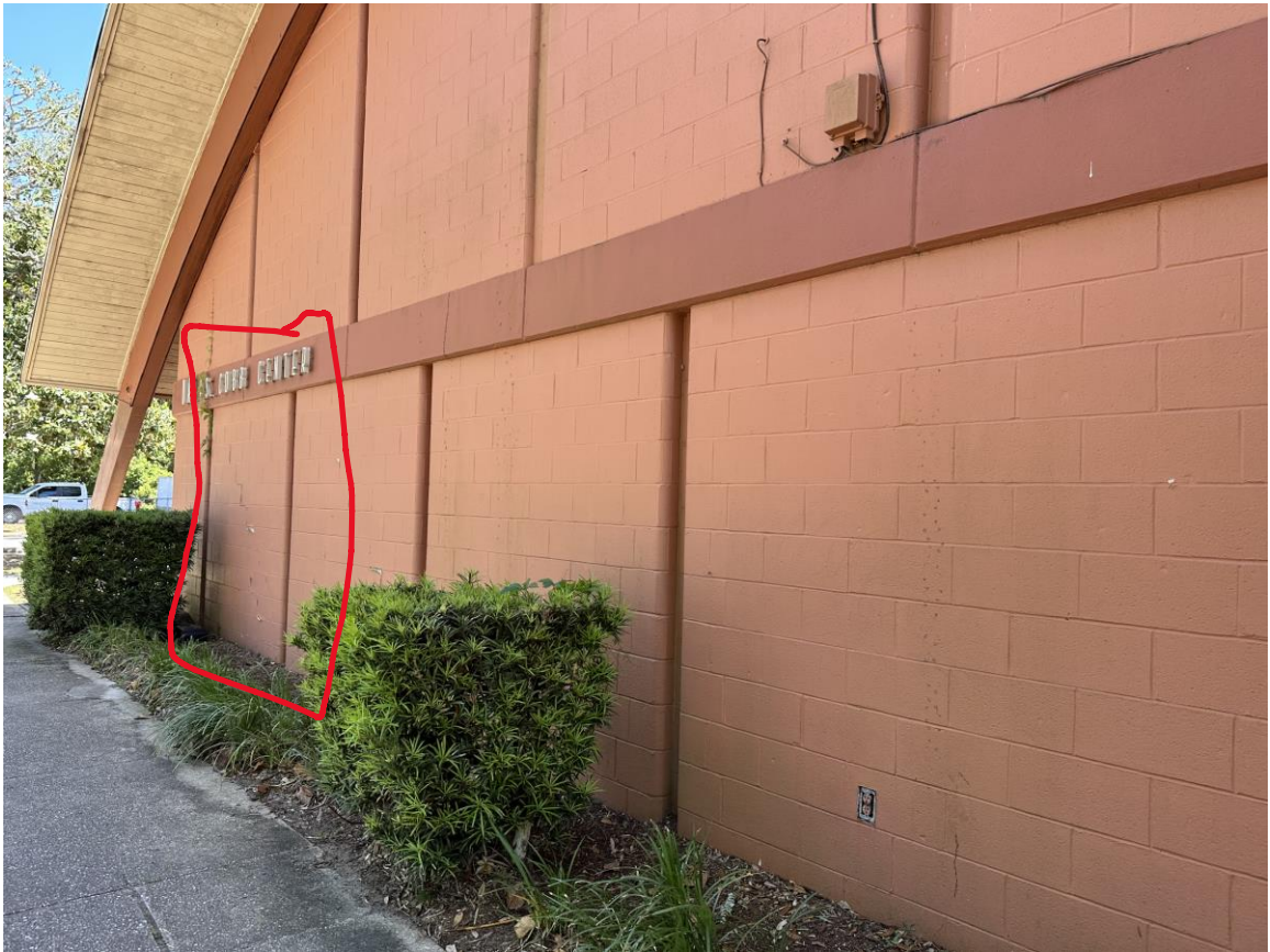
Photo 16 – North Exterior Wall (East Half)
