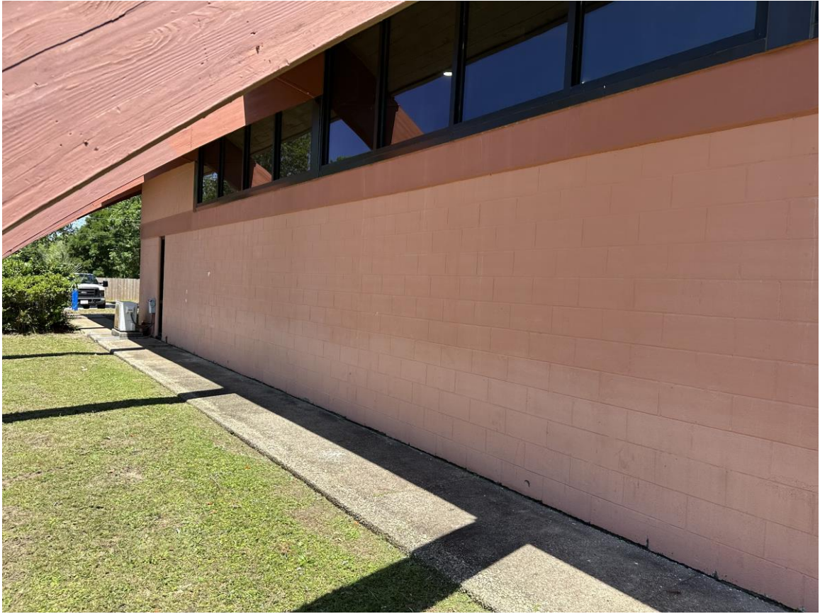
Photo 19 – West Exterior Wall (Looking NE)
