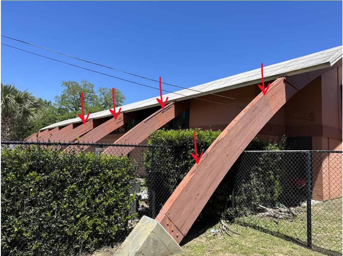
Photo 6 – West Side of Gym (Looking Northeast)
