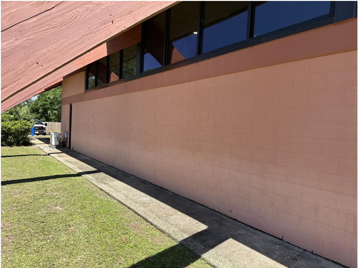
Photo 19 – West Exterior Wall (Looking NE)
