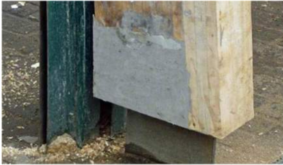
Pic 01 – Sample epoxy repair at wood Column base.
