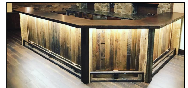
RECLAIMED PALLET BOARD BAR FACE CLADDING
