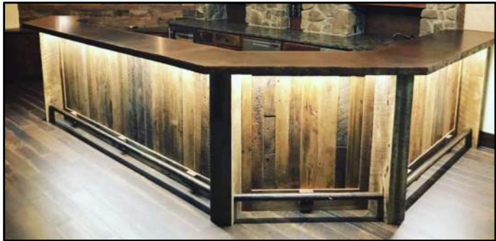
RECLAIMED PALLET BOARD BAR FACE CLADDING
