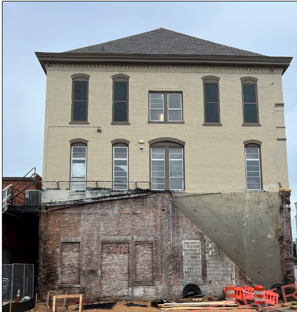
EXISTING VIEW LOOKING WEST FROM WITHIN PROPERTY
