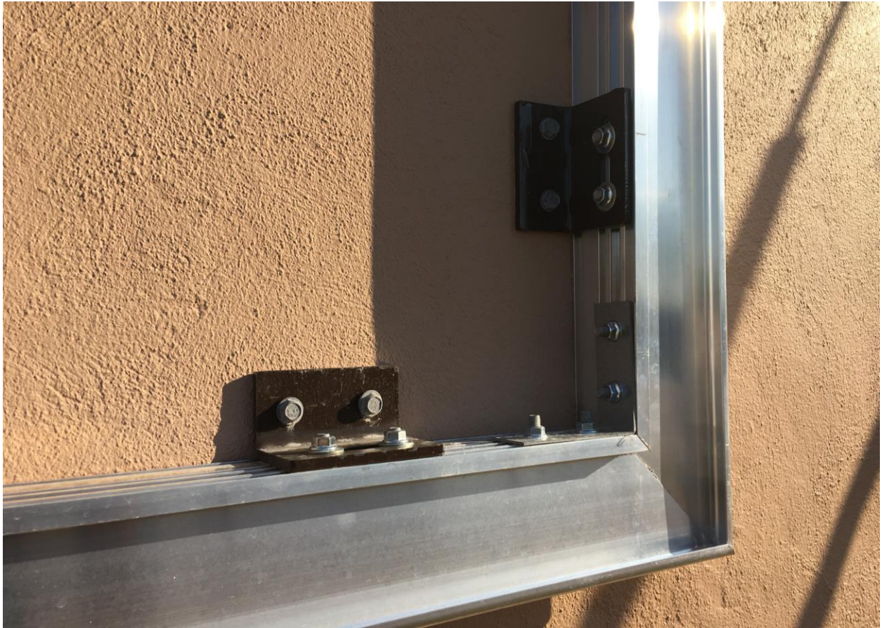
Invisible frame system bolts to the wall. Hidden hardware secures the graphic to the frame.
