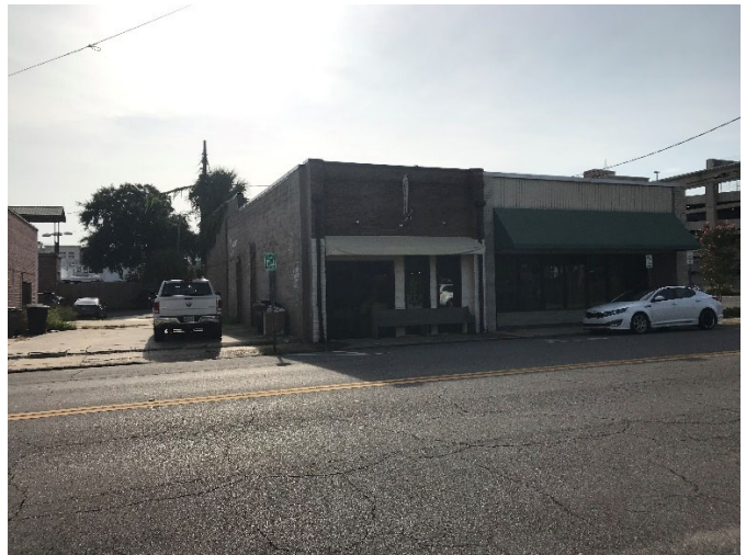
Front View of Site
