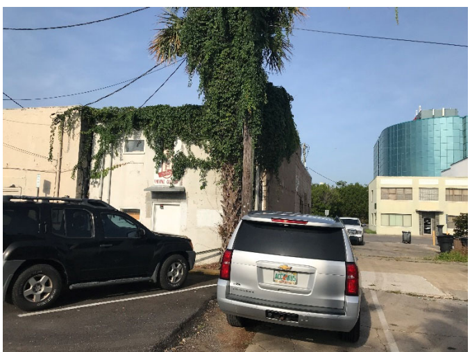
Rear View of Site
