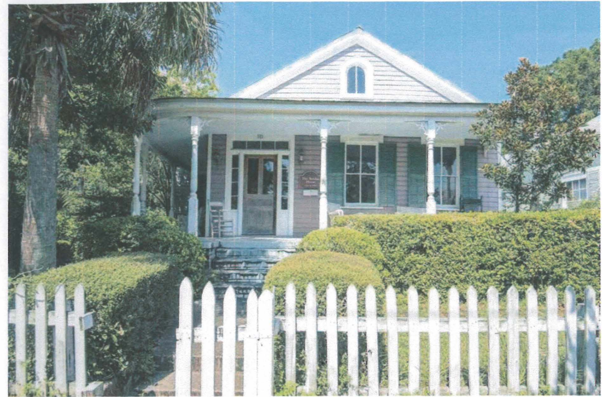
Present Condition - Main Elevation
