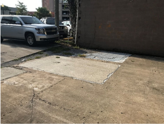
Rear View of Site
