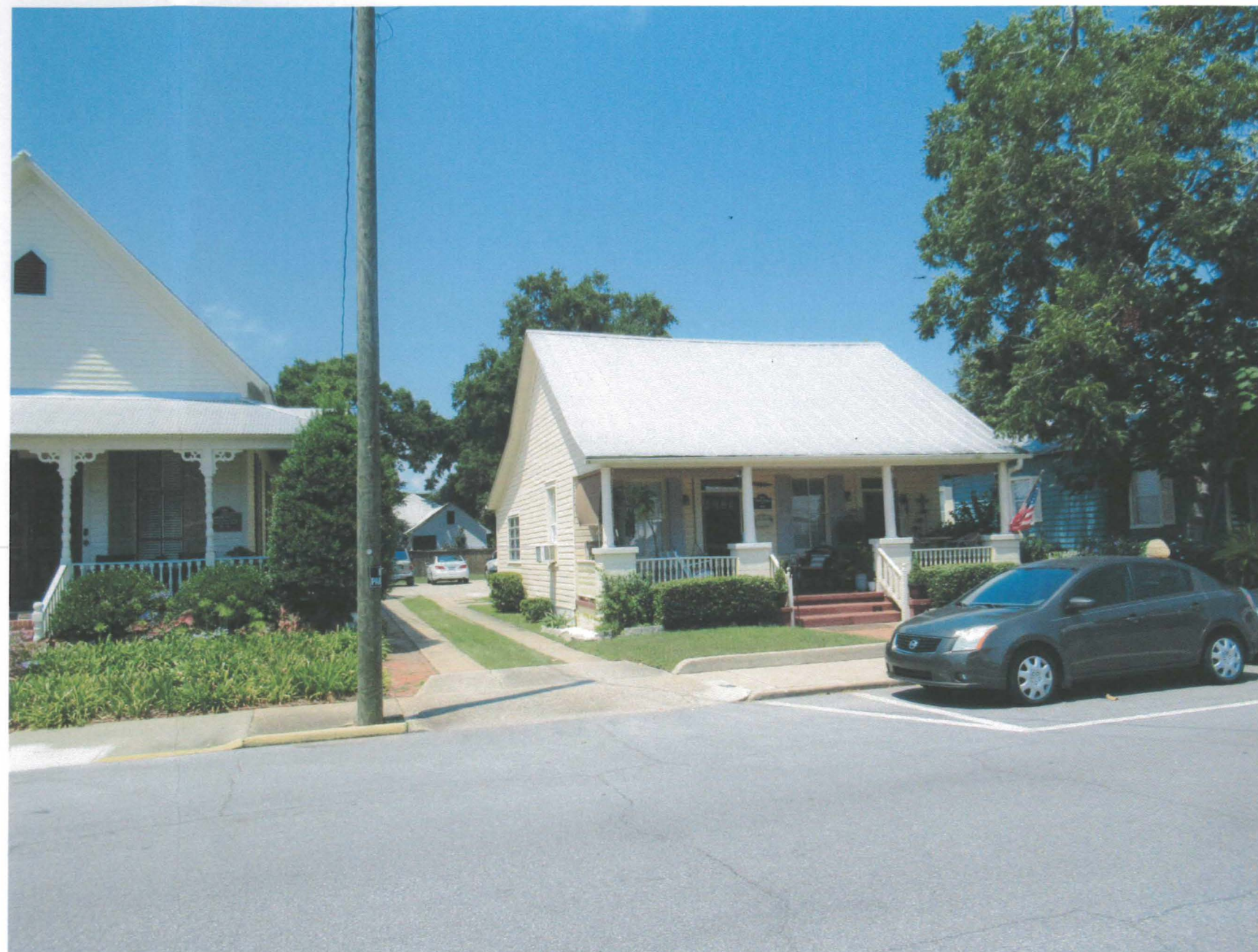
View of Existing Goverment Street Facade
