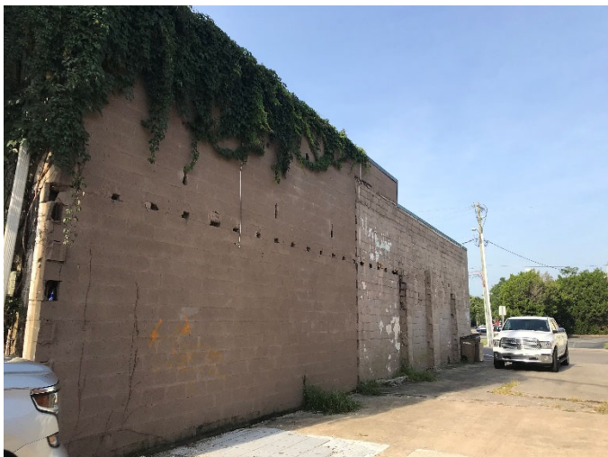
Rear View of Site
