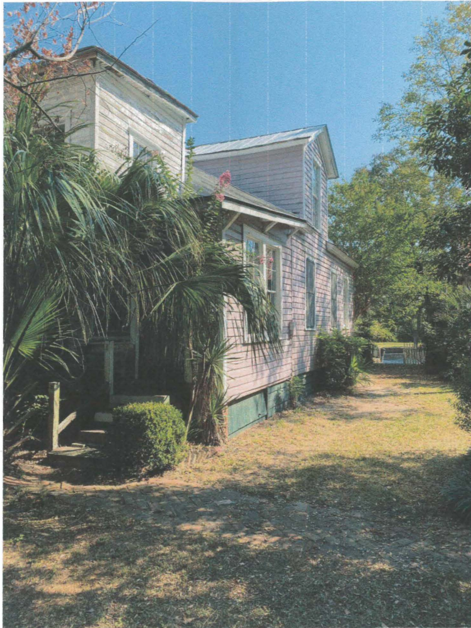
Partial South Elevation View
