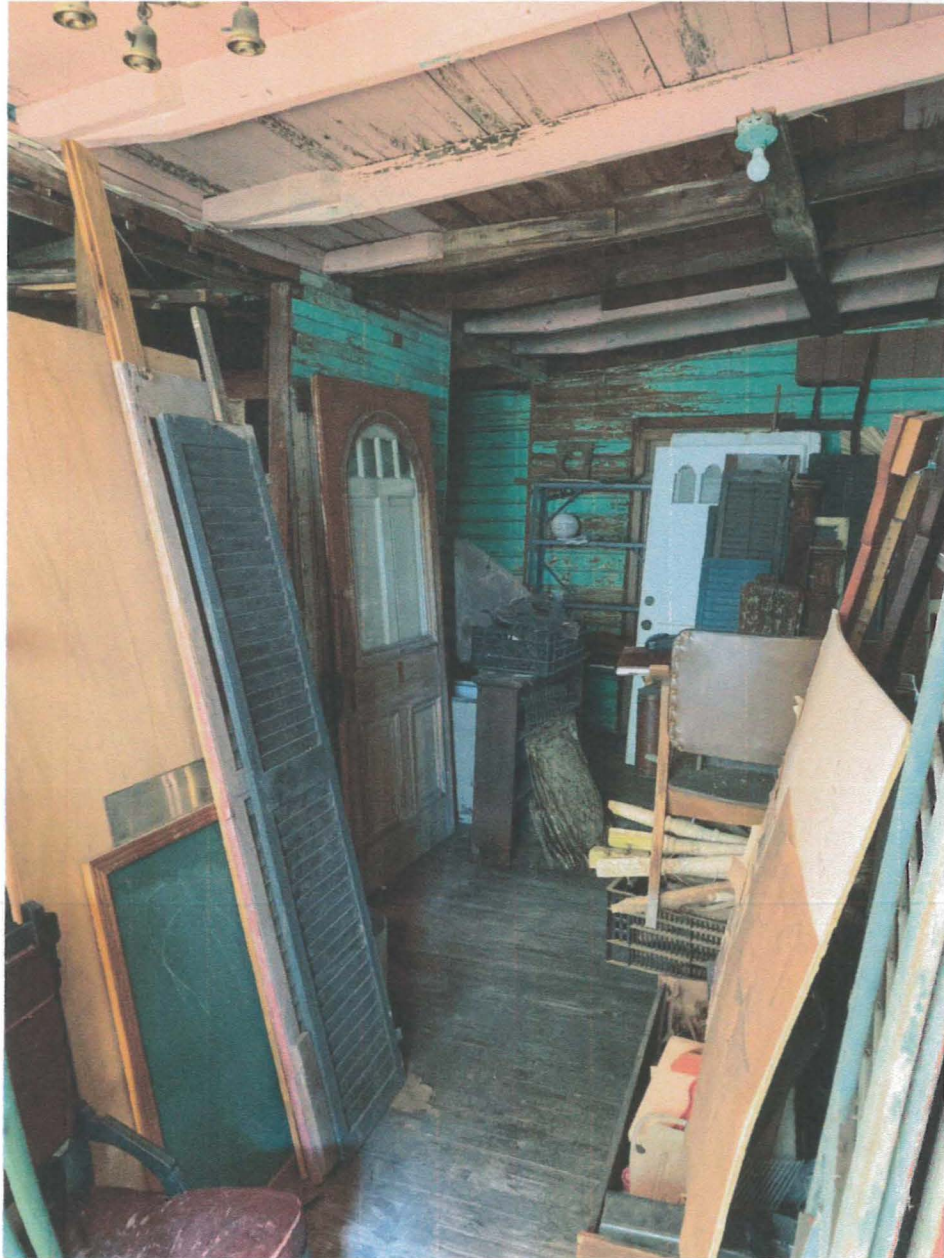
Interior View of Rear Addition to be Demolished
