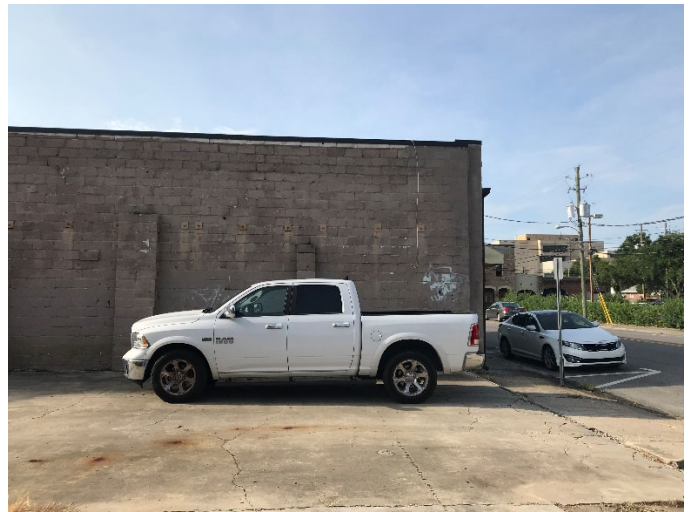
South view of Site
