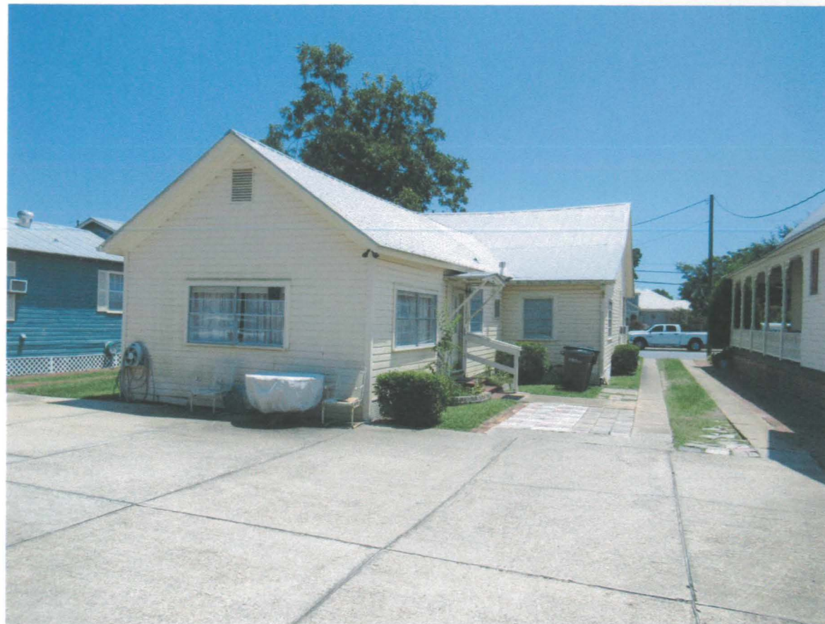
View of Back of Existing House to Receive Addition
