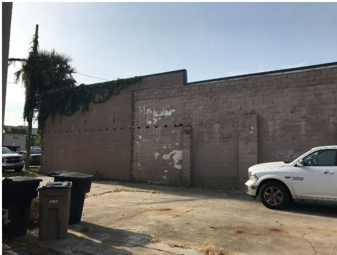
South View of Site
