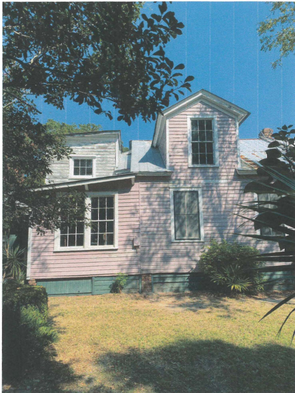
Partial South Elevation View
