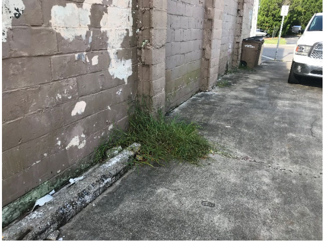
View of Existing Adjacent Building Wall
