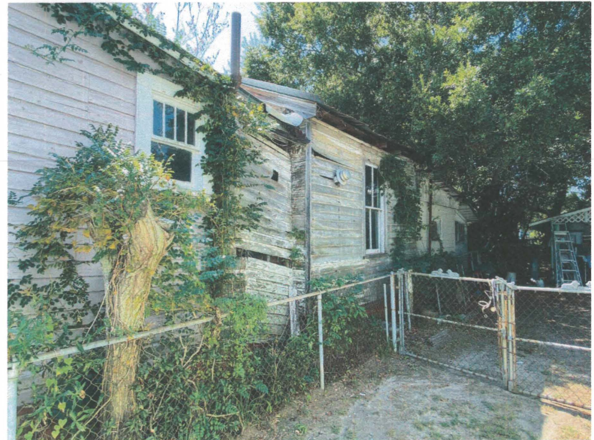
North Side Rear Addition to be Demolished
