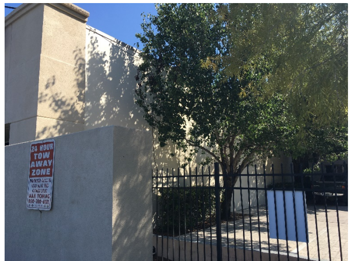
View of South Side Existing
