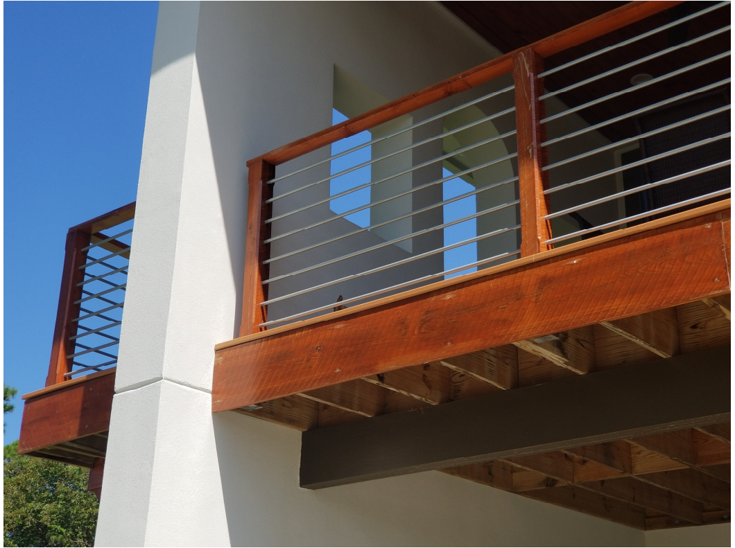
Railings - Cypress with stain, 1/2" galvanized rods, natural finish
