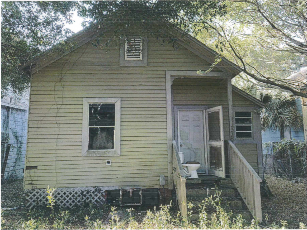
BACK ENTRY - SOUTH
