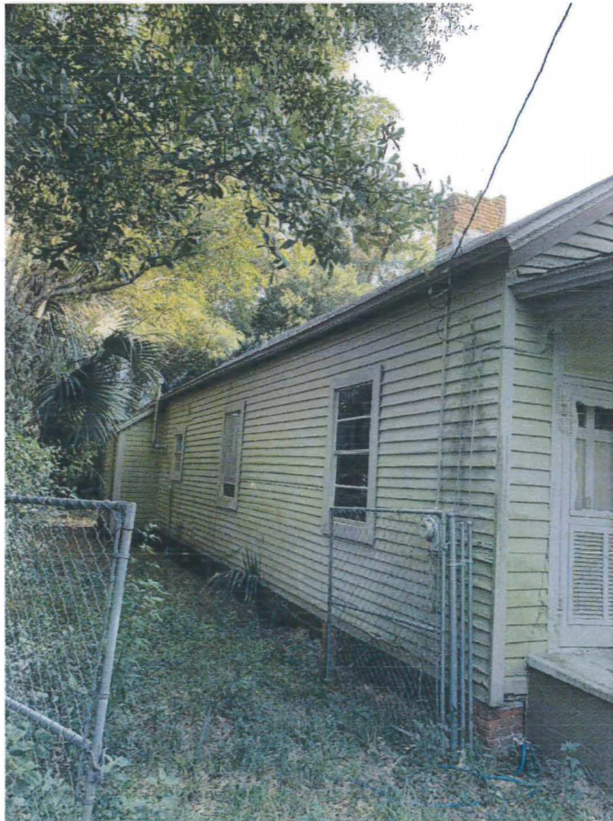
EAST SIDE OF HOUSE
