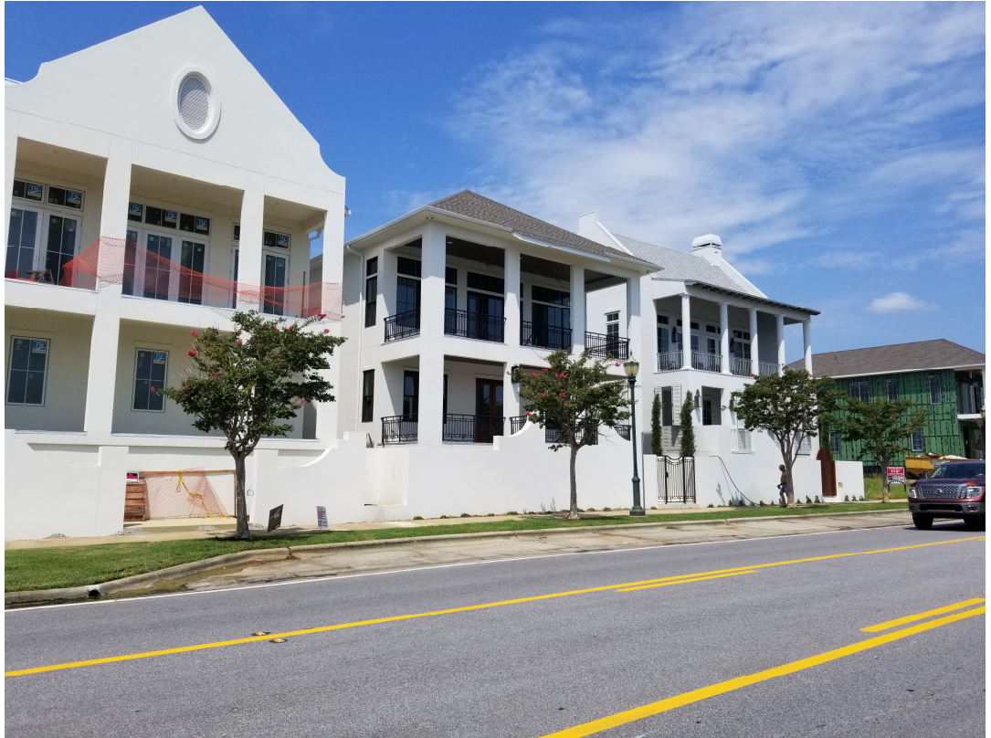
Closest Houses (divided by easment and alley), taken from Admiral Mason park looking West
