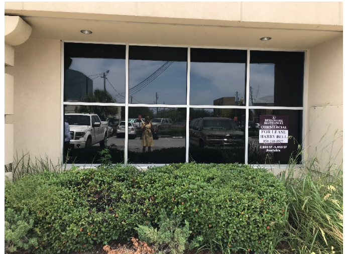
View of Existing Storefront
