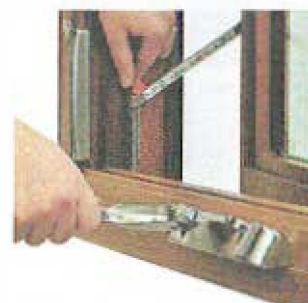
WOCD limits the sash opening to less than four inches.
