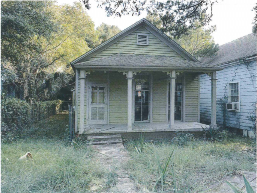
EXISTING STREET VIEW
