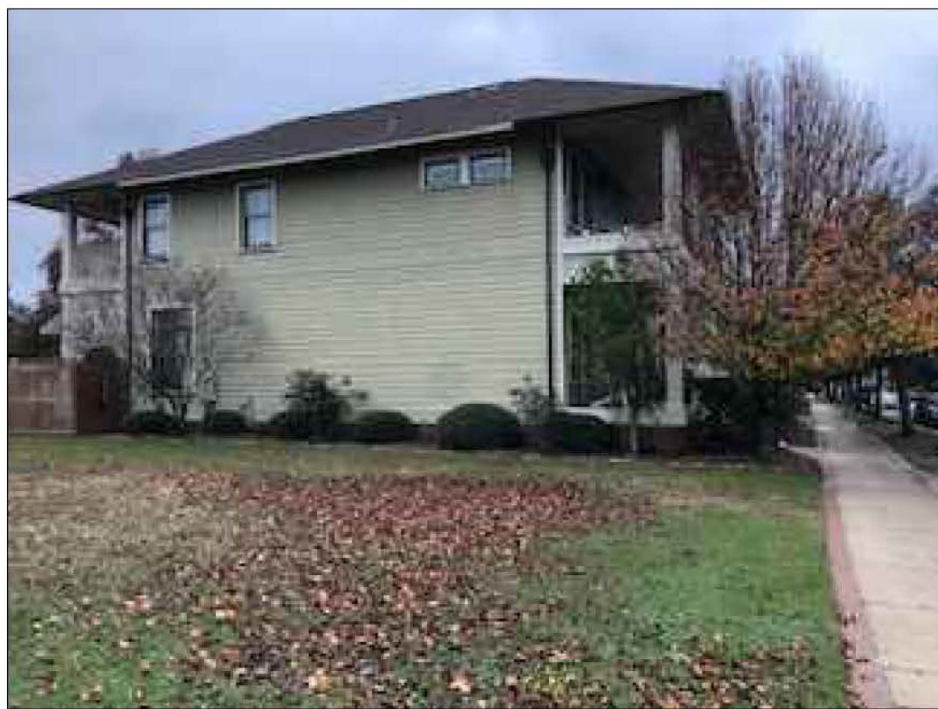
SITE PHOTO FACING WEST
