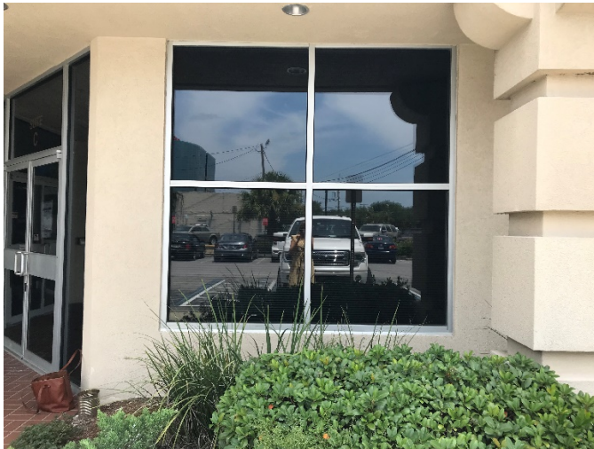
View of Existing Storefront
