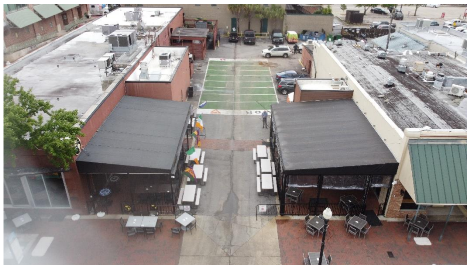
Views of Existing Front
