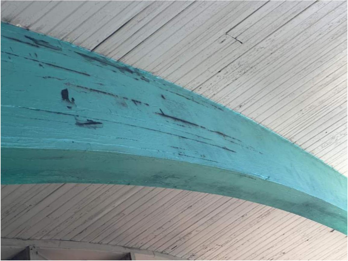
Arch #1 at South Side of Bldg (Viewing West portion of Arch between west wall at top of Arch) NOTE: Delamination
