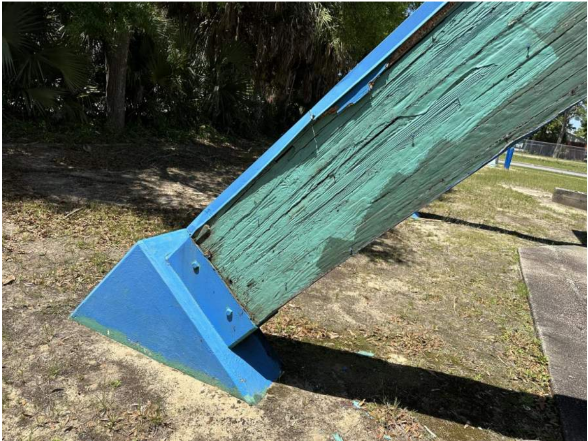
Arch #6; West End of Arch near NW corner of Bldg (Viewing West portion of Arch just above Concrete Buttress) NOTE: Severe delamination & decay
