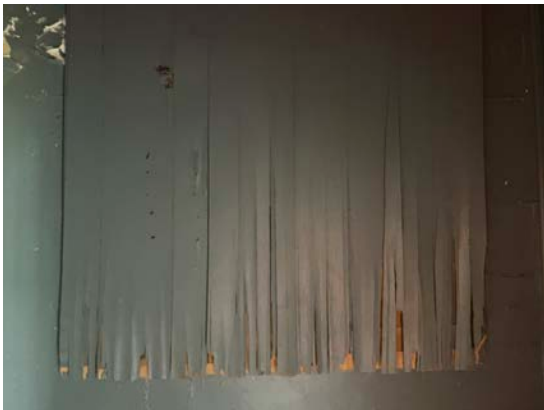
Laundry Room Interior Wall
