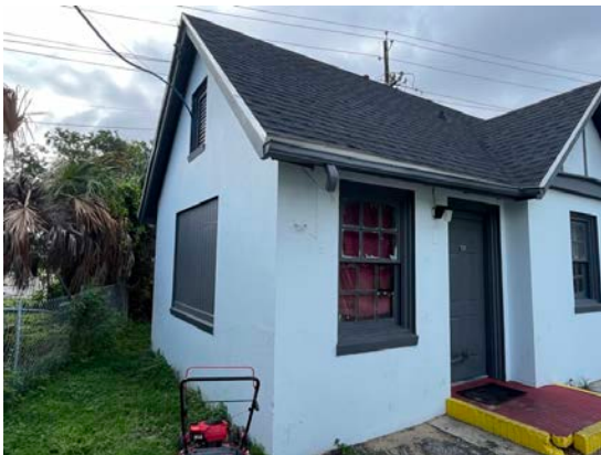
Missing Downspout
