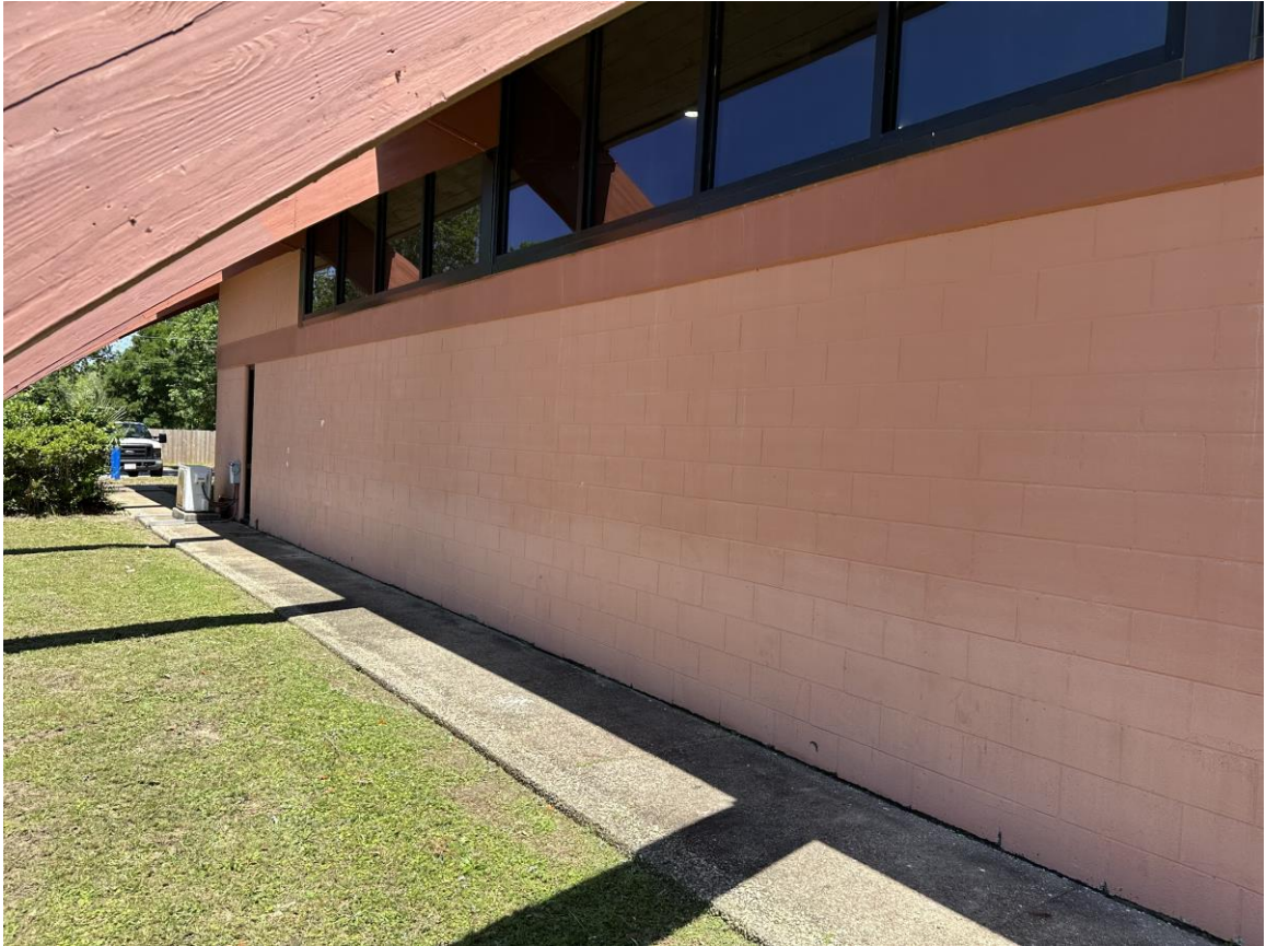
Photo 19 – West Exterior Wall (Looking NE)
