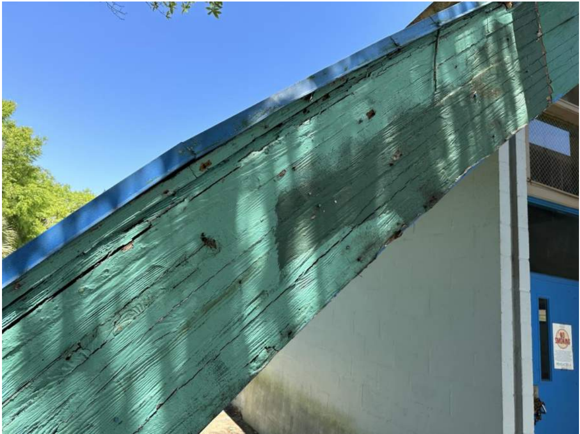
Arch #1 at South Side of Bldg (Viewing West End of Arch between Concrete Buttress and west wall) NOTE: Excessive / Severe Decay & Delamination
