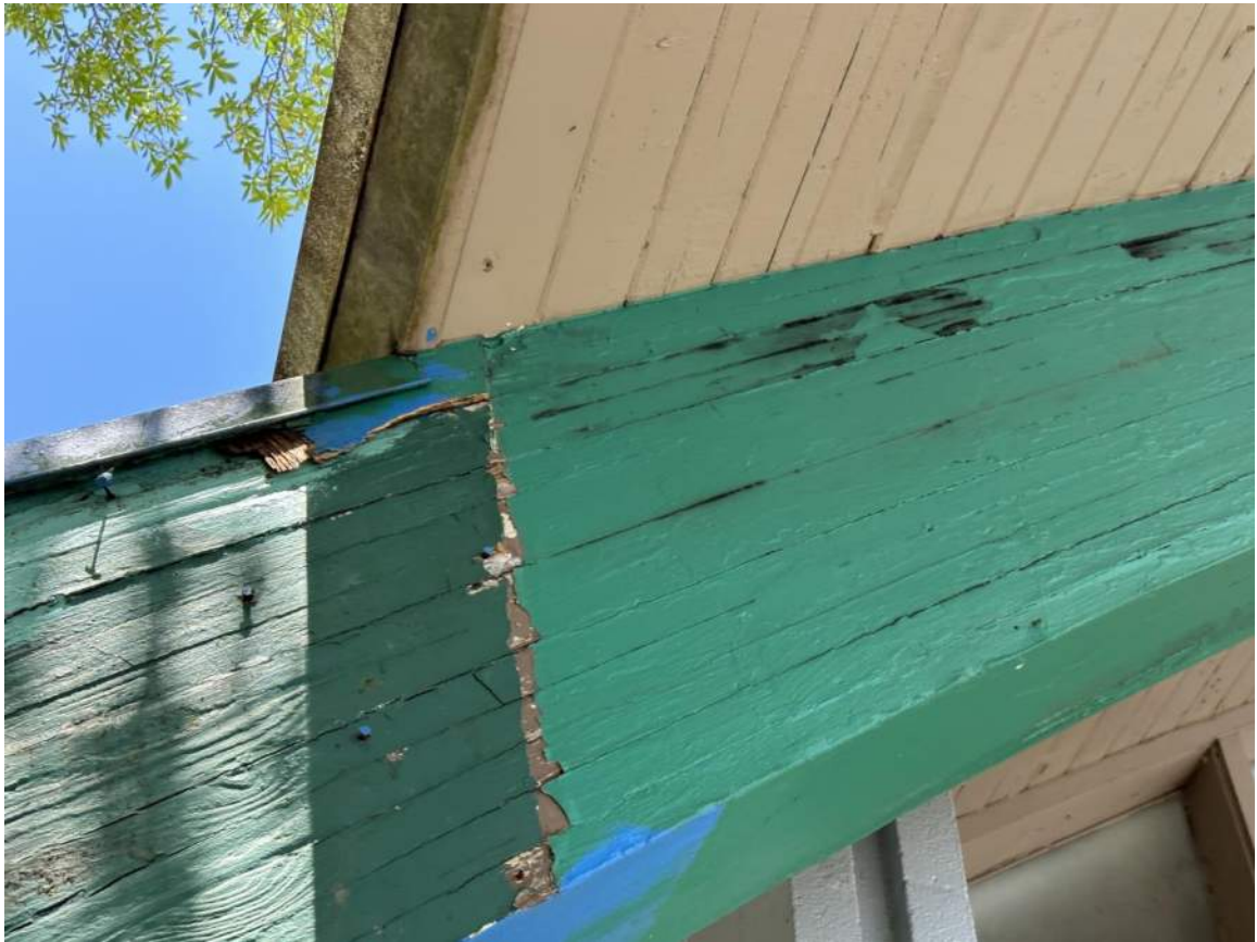
Arch #1 at South Side of Bldg (Viewing West End of Arch at west wall) NOTE: Severe Decay & Delamination
