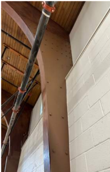
Pic 03 – Sample repair utilizing steel side plates on the existing arch.
