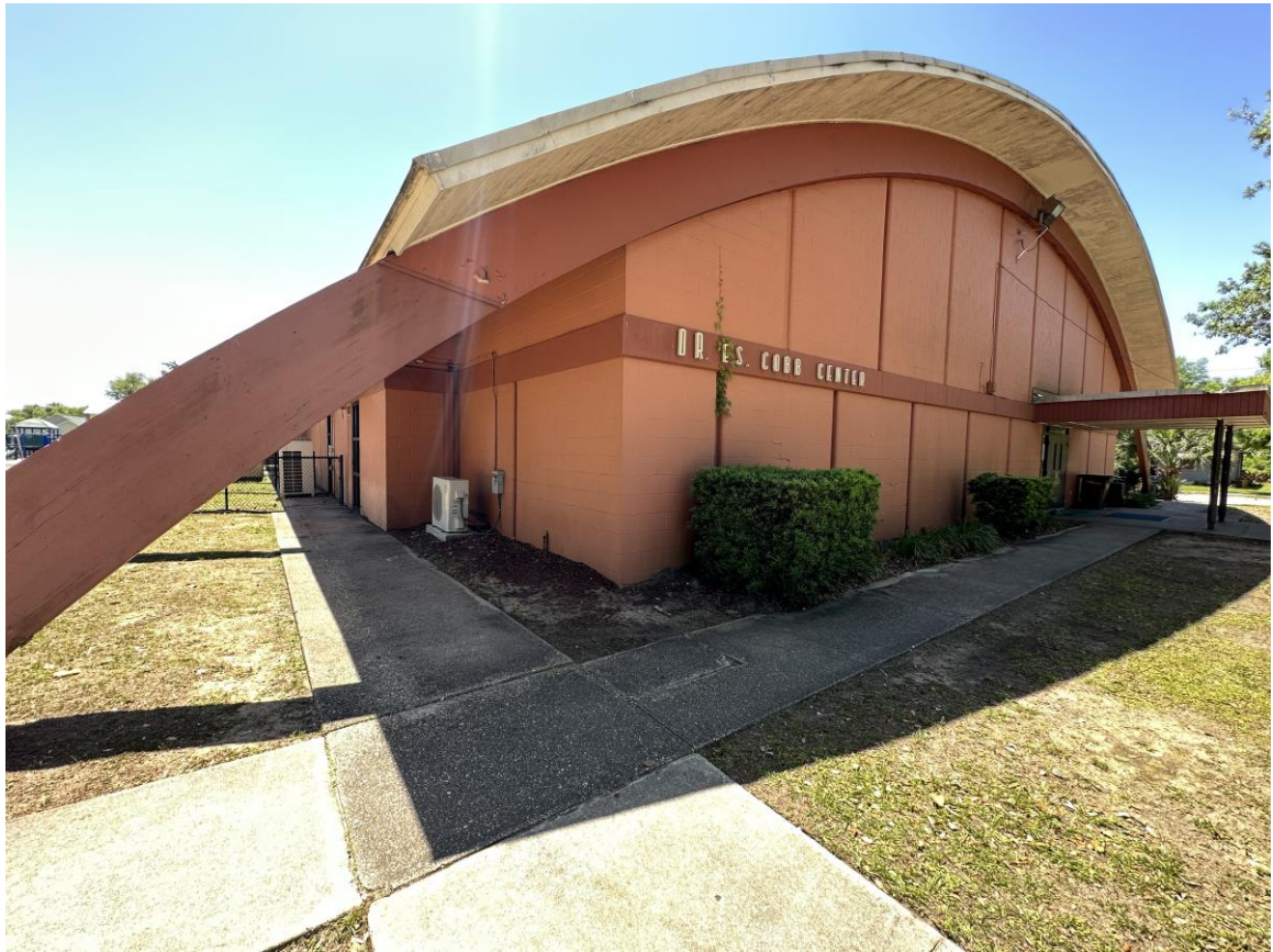
Photo 2 – Gym Exterior (Looking Southwest)
