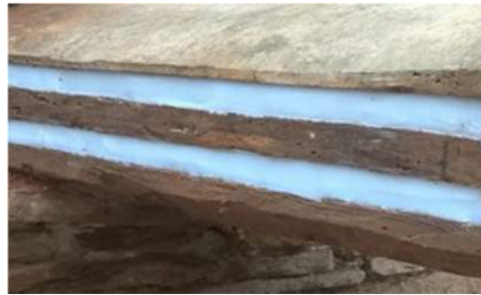
Pic 02 – Sample epoxy repair at deteriorated side trim removed and repaired with epoxy repair in lam's.
