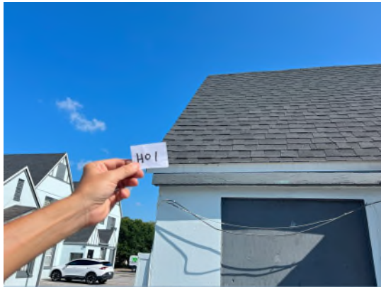
Photo 3: H01- Outside stucco/block
