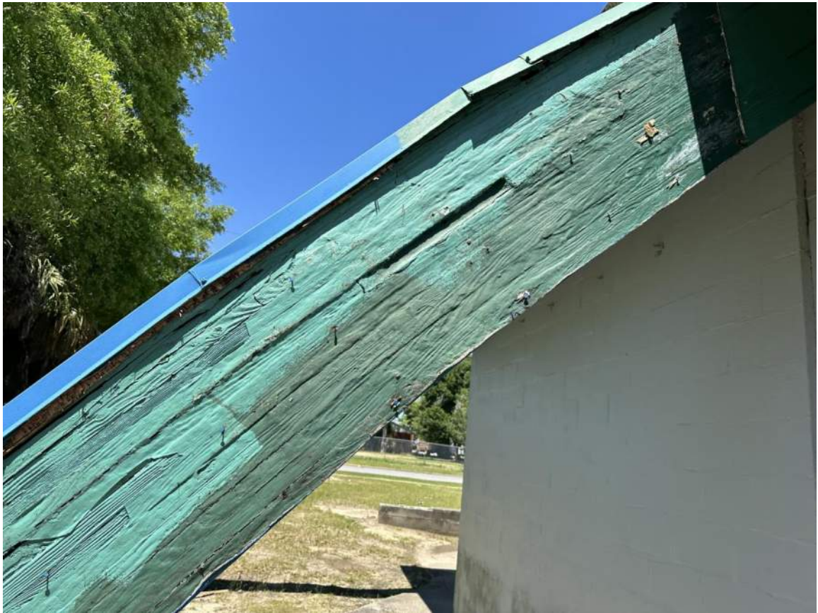
Arch #6; West End of Arch near NW corner of Bldg (Viewing West portion of Arch just above Concrete Buttress and Near West Wall) NOTE: Severe delamination & decay
