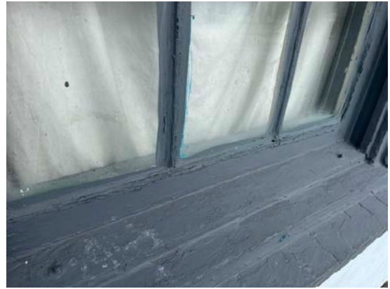
Exterior View - Windows
