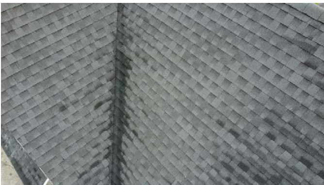
Roof Closeup Example
