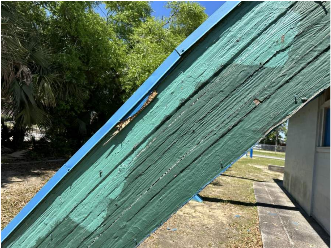
Arch #2; West End near SW corner of Bldg (Viewing West portion of Arch just above Concrete Buttress) NOTE: Severe delamination & decay
