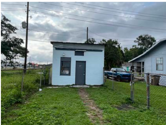
Administrative Laundry Facility
