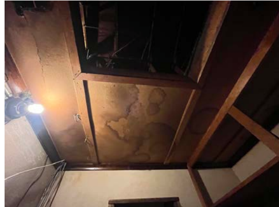
Building #11 - Second Floor
