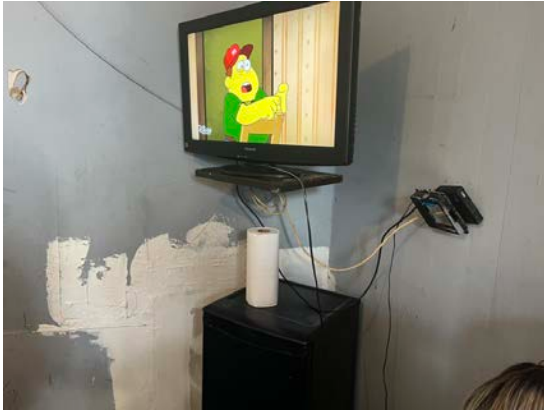
Unit #106 Interior Walls
