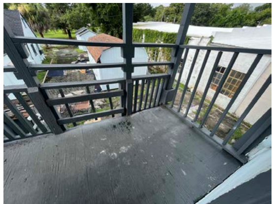
Building #11 Second Story
