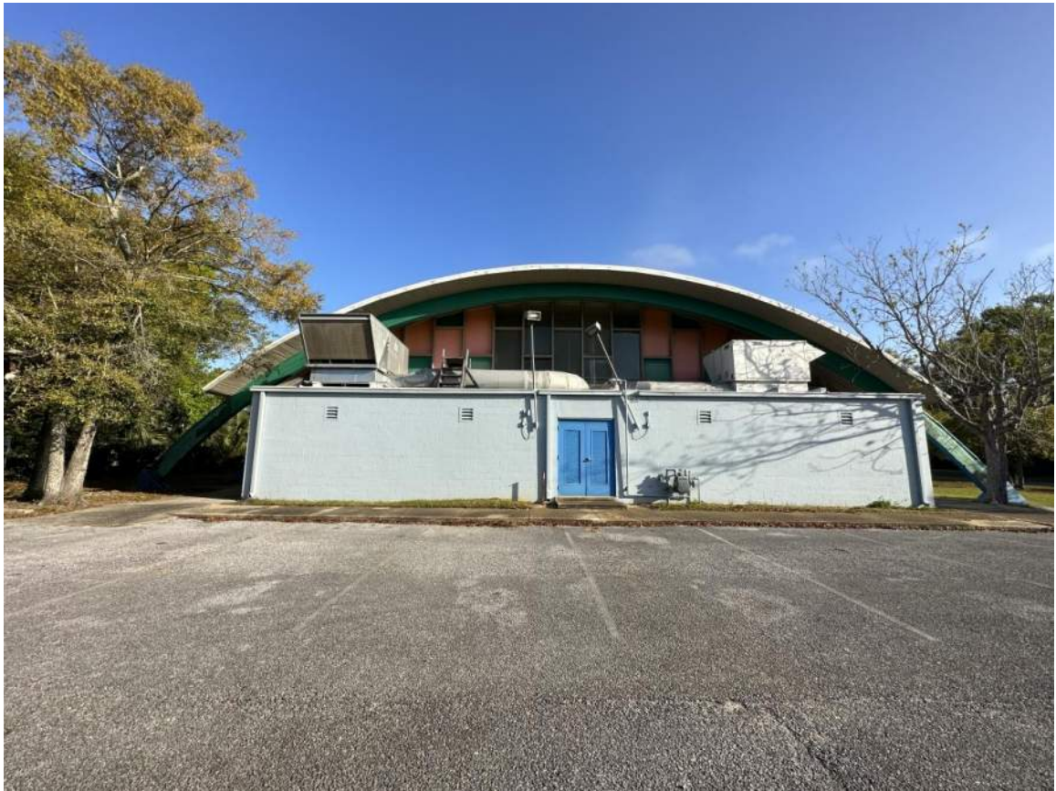
South Side of Bldg (Looking North)
