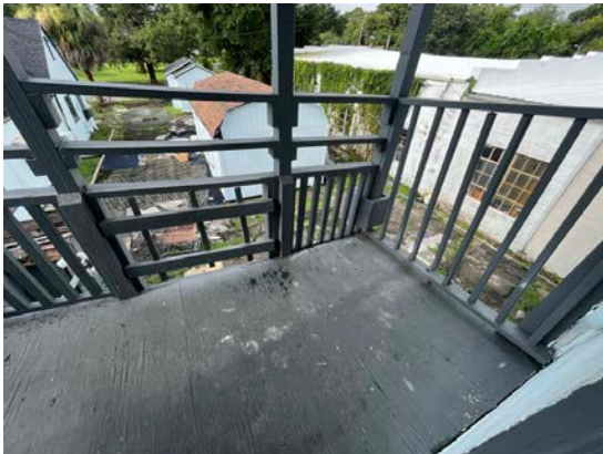
Building #11 Second Story
