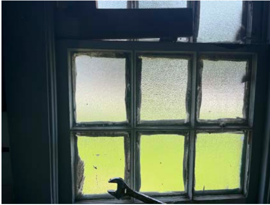
Unit Window - Screwed Closed
