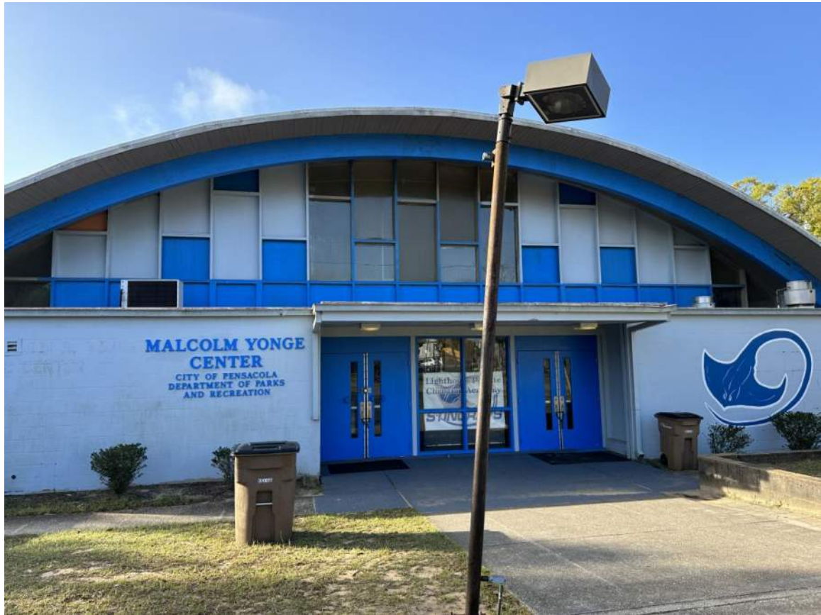
North Side of Building (Looking South)
