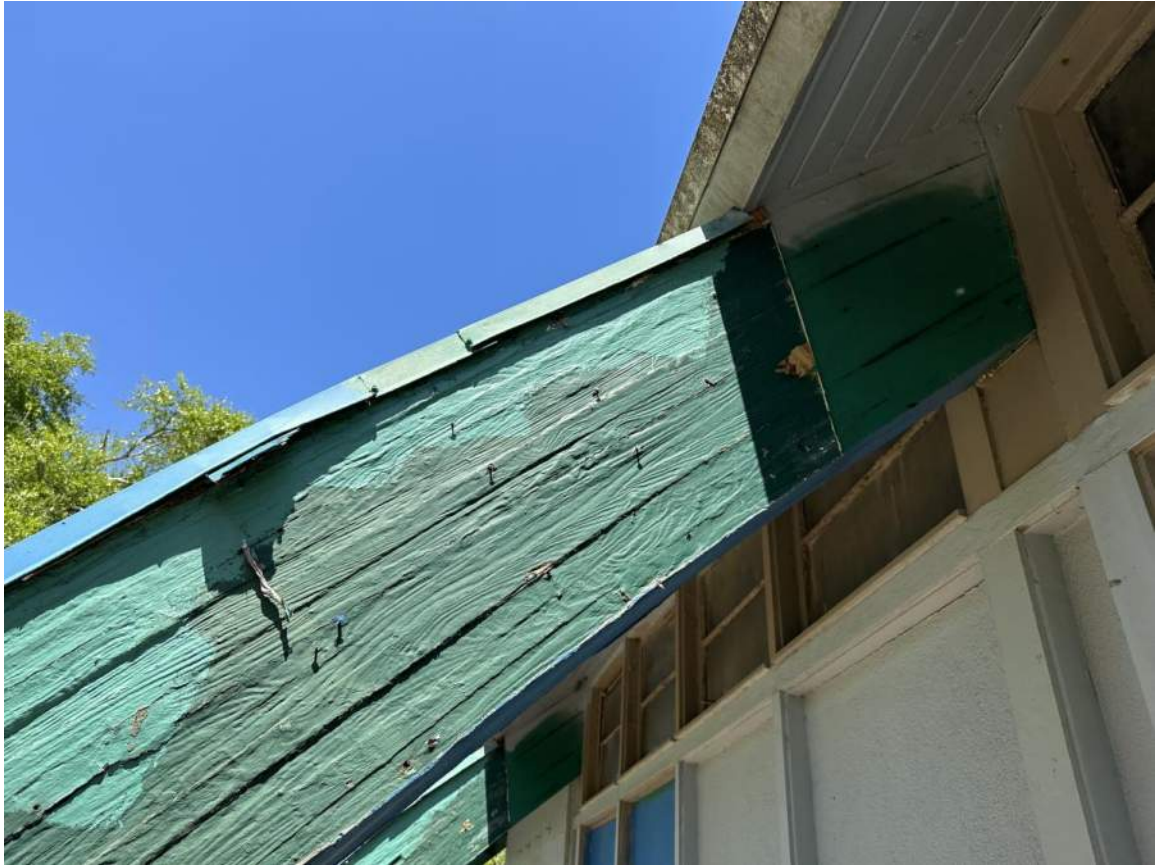
Arch #2; West End near SW corner of Bldg (Viewing West portion of Arch near west wall of building) NOTE: Severe delamination & decay
