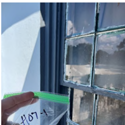
Photo 9: H07- Window Caulking
