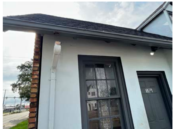
Damaged Gutter
