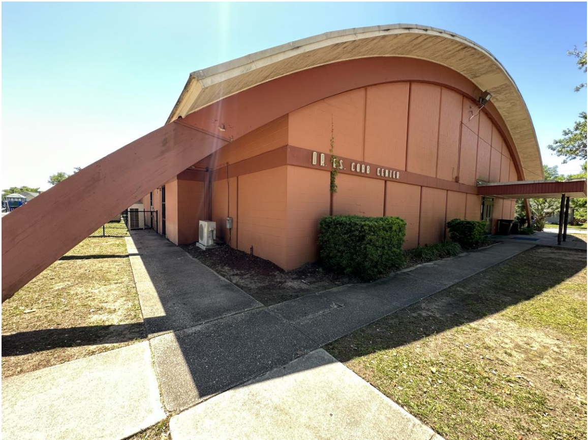
Photo 2 – Gym Exterior (Looking Southwest)
