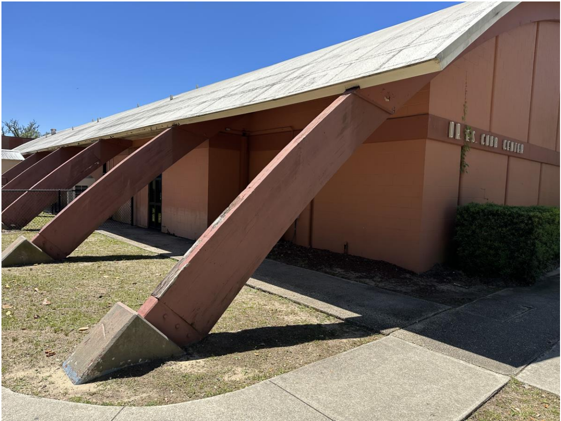
Photo 3 – Gym Exterior (East End of Arches)
