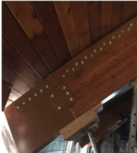
Pic 05 – Sample repair utilizing steel HSS section, existing glulam arch shown on high end of photo and HSS on low end, Glulam on high end
