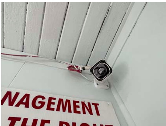
Security Camera System
