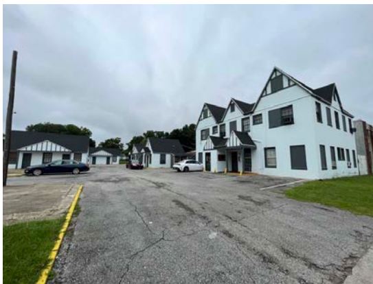
Parking Area Overview
