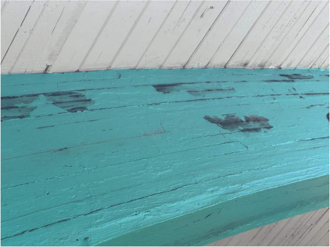
Arch #1 at South Side of Bldg (Viewing West portion of Arch at west wall) NOTE: Delamination
