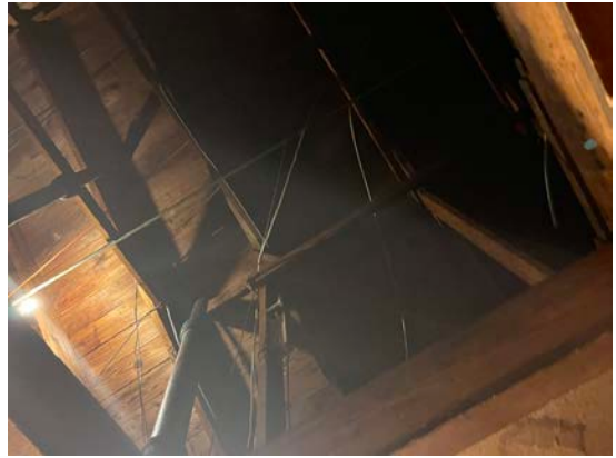
Building #11 - Second Floor
