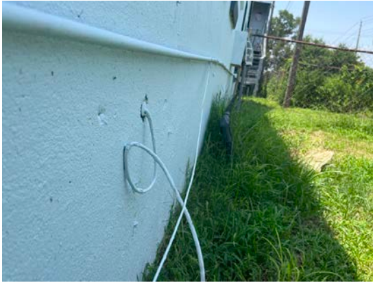
Building #2 Exterior Wall
