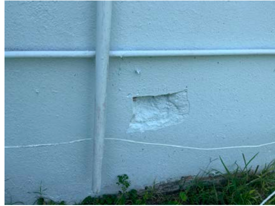
Building #2 West Elevation Wall
