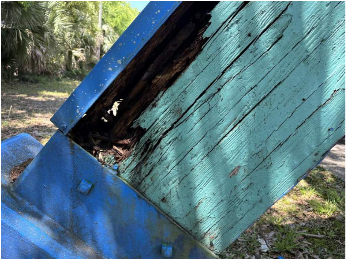
Arch #1 at South Side of Bldg (Viewing West End of Arch at Concrete Buttress) NOTE: Excessive / Severe Decay
