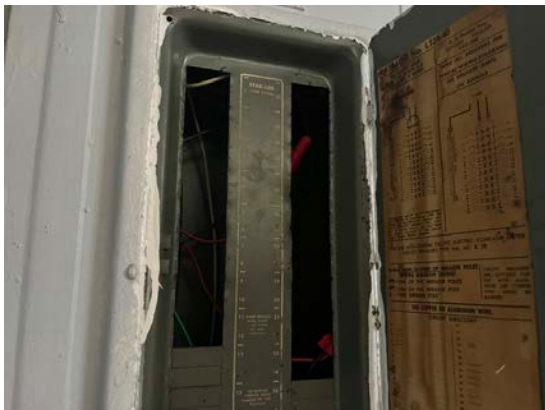
Building #11 - Interior Panel
