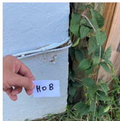
Photo 10: H08- Concrete block/office
