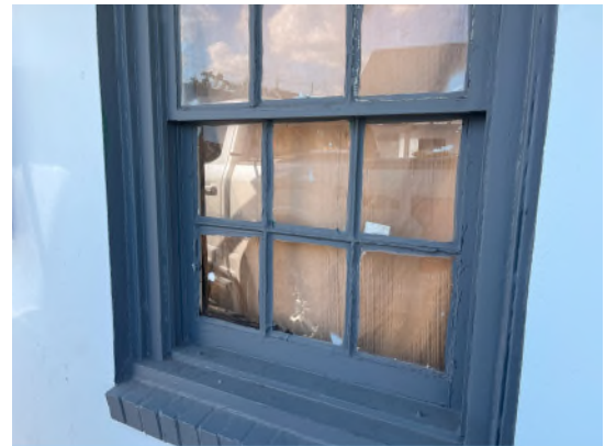
Photo 6: H04- Window Caulking
