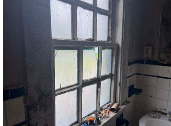
Unit Window Example - Interior View
