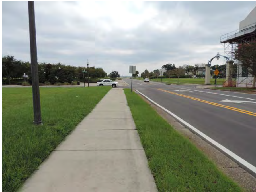
View South along South 9 th Avenue
