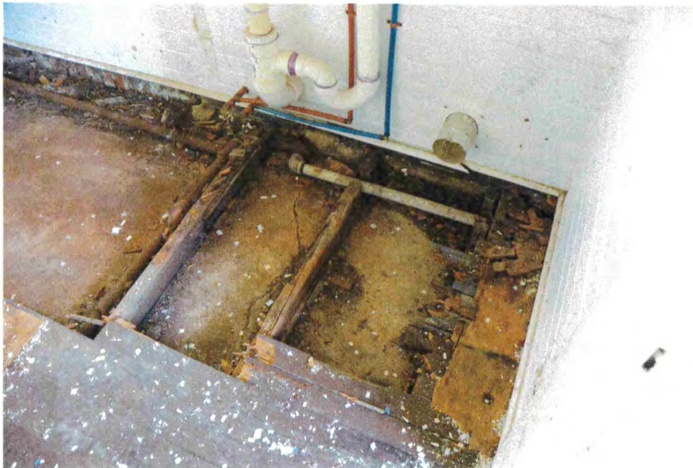
Photo 2 - 1st Floor Flooring
