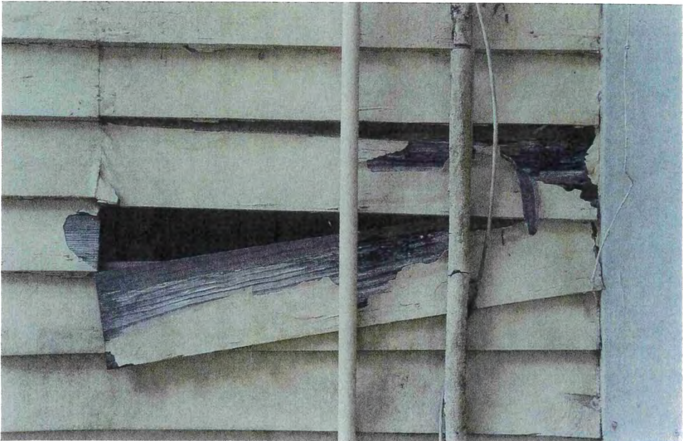
Photo 7-2 - Wood Lap Siding and Trim
