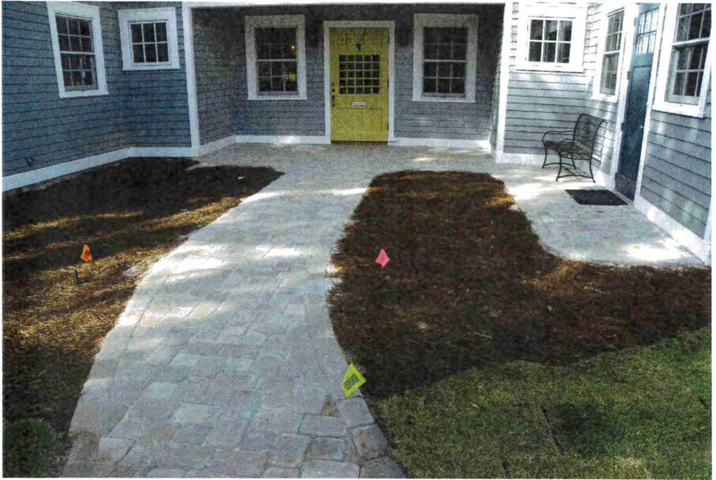
Photo 1 – Brick pavers leading to main entrance. 10/28/16
