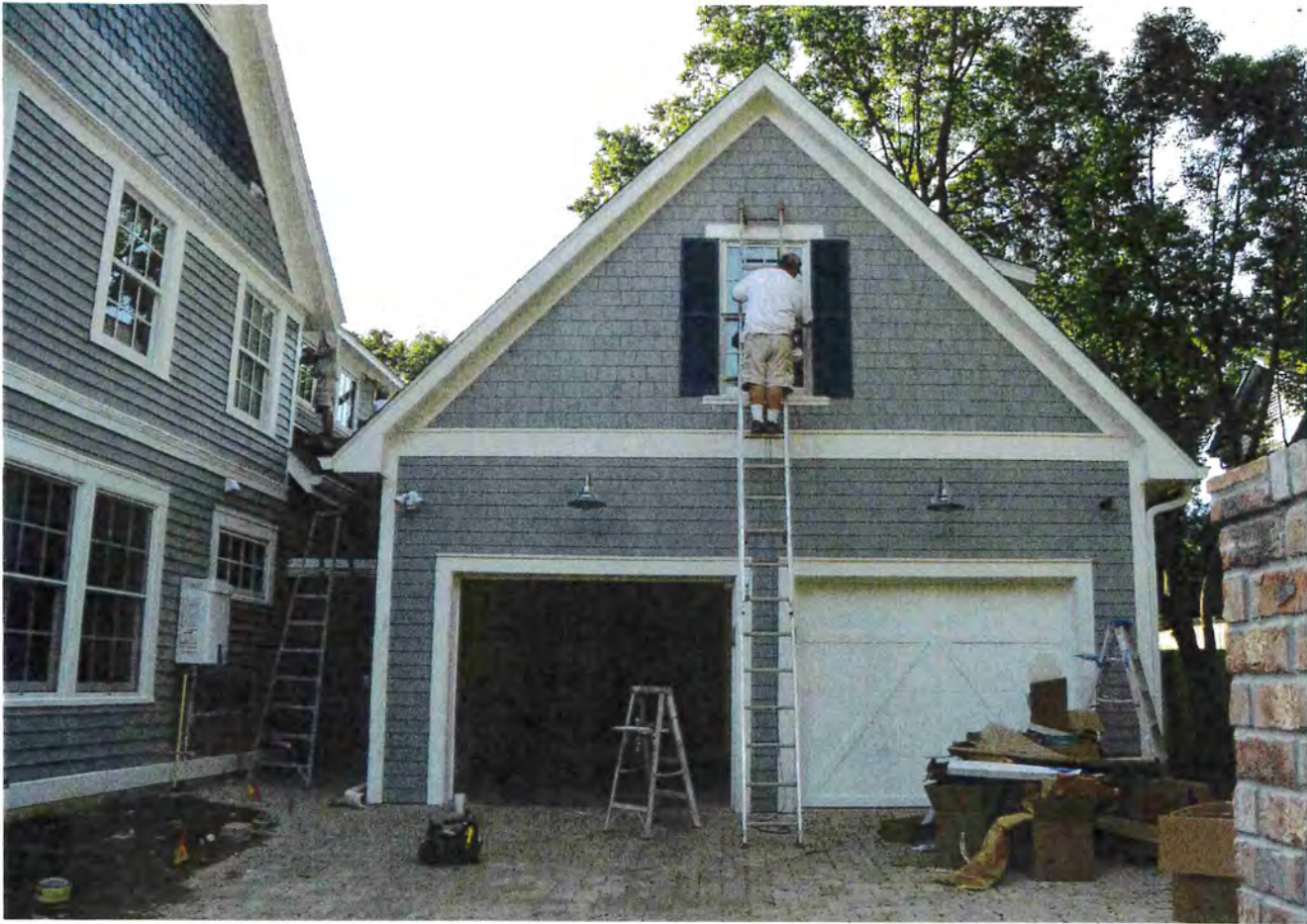
Photo 5 – New garage addition. 10/28/16
