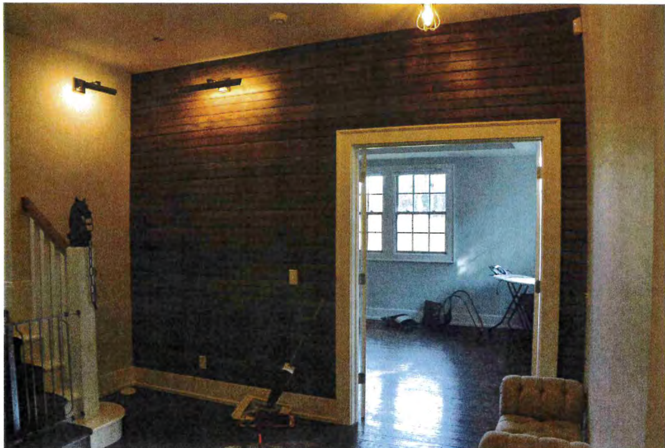
Photo 16 – Salvaged tongue and groove boards reinstalled on interior wall. 10/28/16
