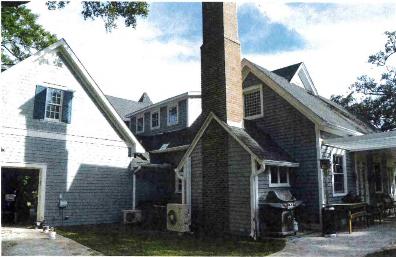
Photo 6 – Restored west façade (rear of the house). 10/28/16
