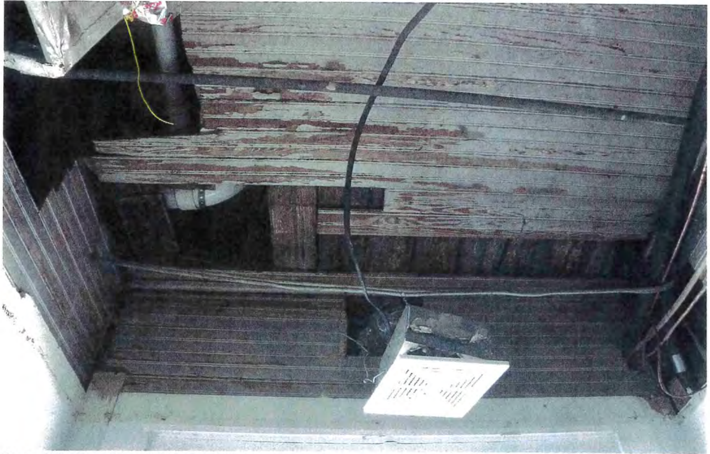
Photo 9-2 - Tongue and Groove Ceilings
