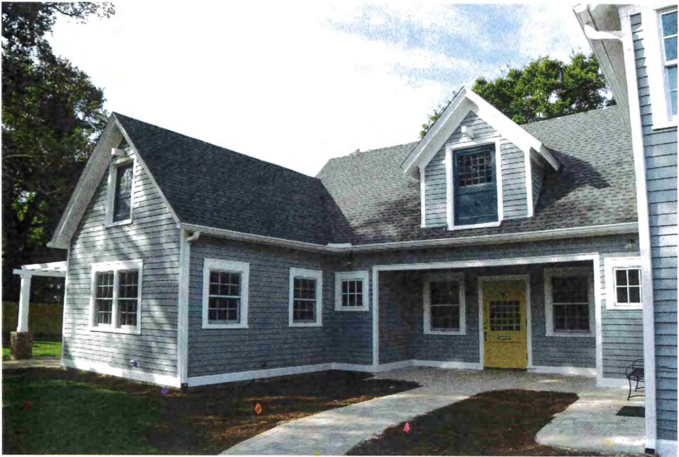
Photo 9 – Restored east façade and main entrance. 10/28/16
