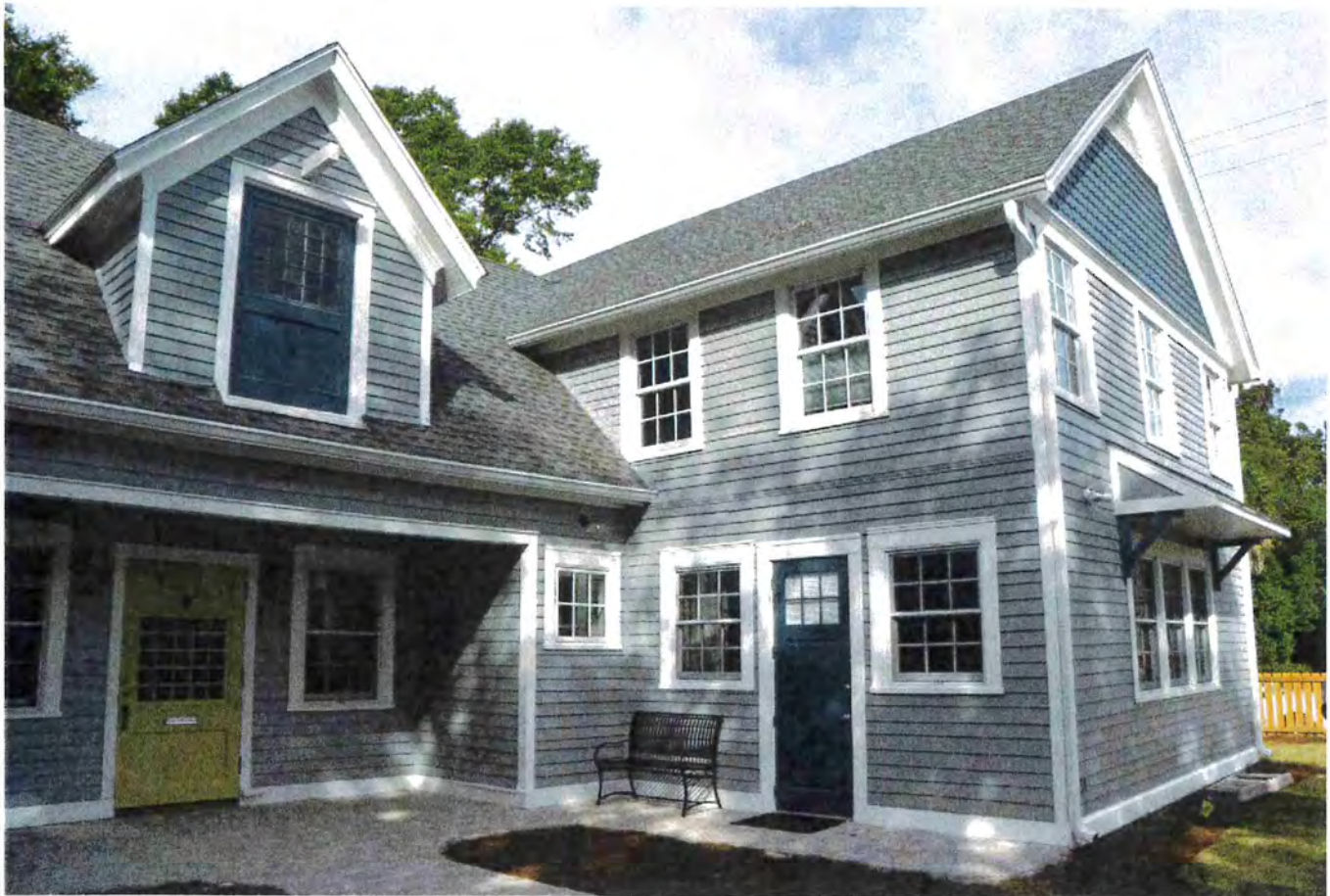
Photo 10 – Restored east façade and main entrance. 10/28/16
