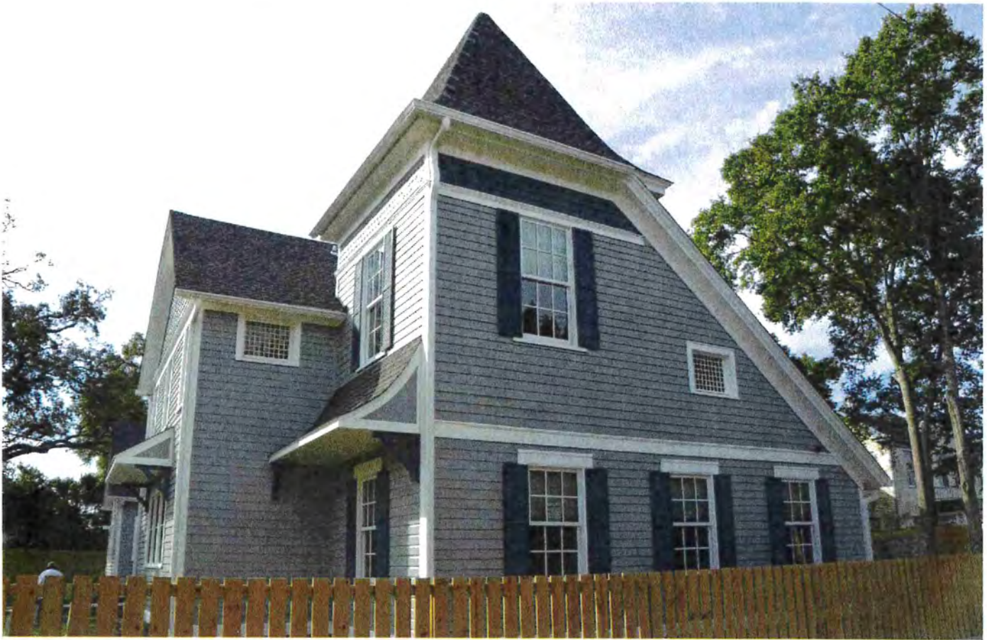
Photo 3 – Restored north façade. 10/28/16
