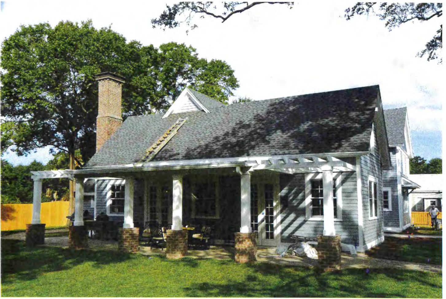
Photo 7 – Restored south façade (rear of the house). 10/28/16
