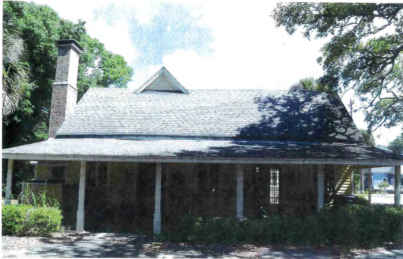
Photo 11-1 - Brick Porch and Roof
