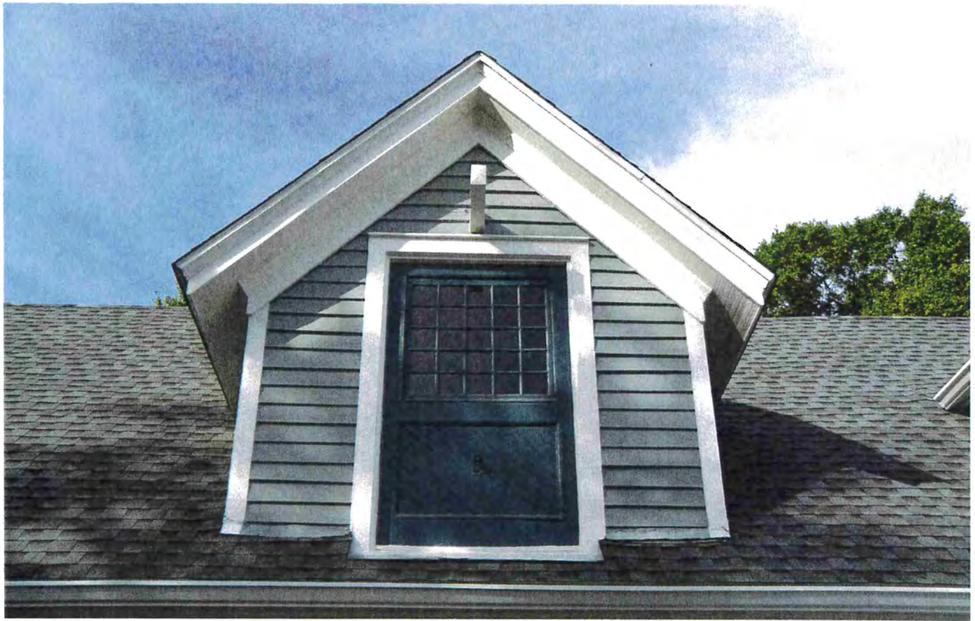
Photo 15 – Restored dormer above entry on east façade. 10/28/16
