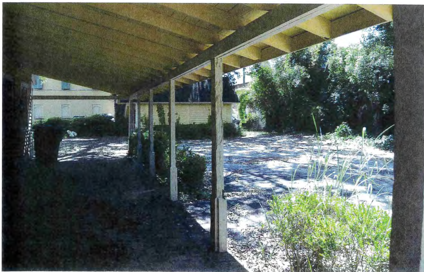
Photo 11-2 - Brick Porch and Roof
