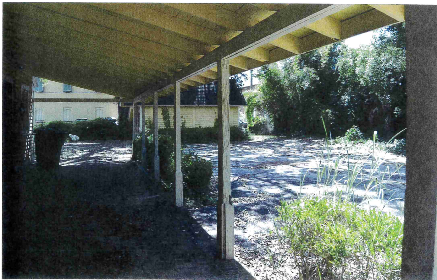
Photo 11-2 - Brick Porch and Roof
