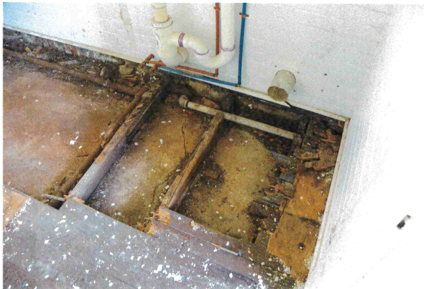
Photo 2 - 1st Floor Flooring
