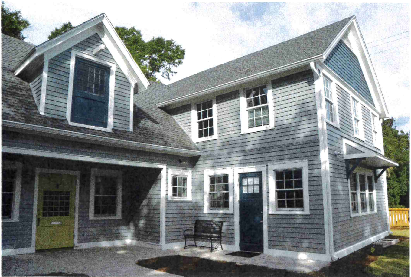
Photo 10 – Restored east façade and main entrance. 10/28/16
