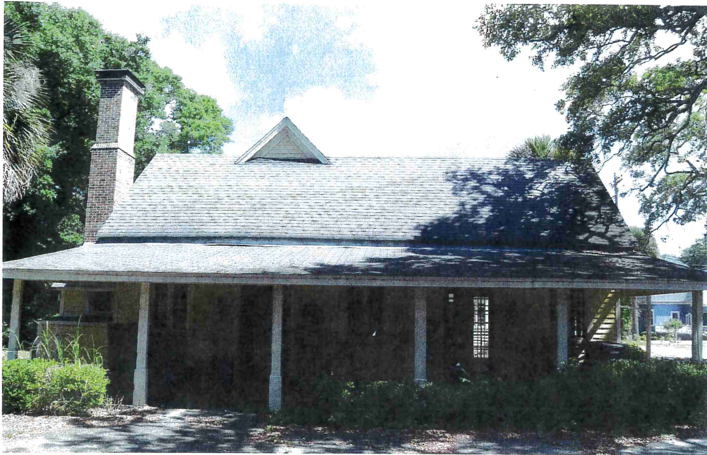
Photo 11-1 - Brick Porch and Roof
