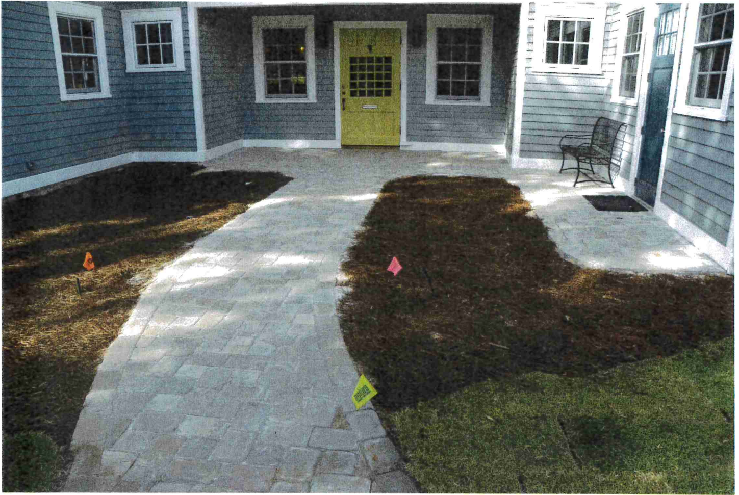
Photo 1 – Brick pavers leading to main entrance. 10/28/16
