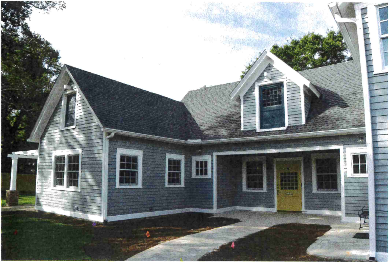
Photo 9 – Restored east façade and main entrance. 10/28/16
