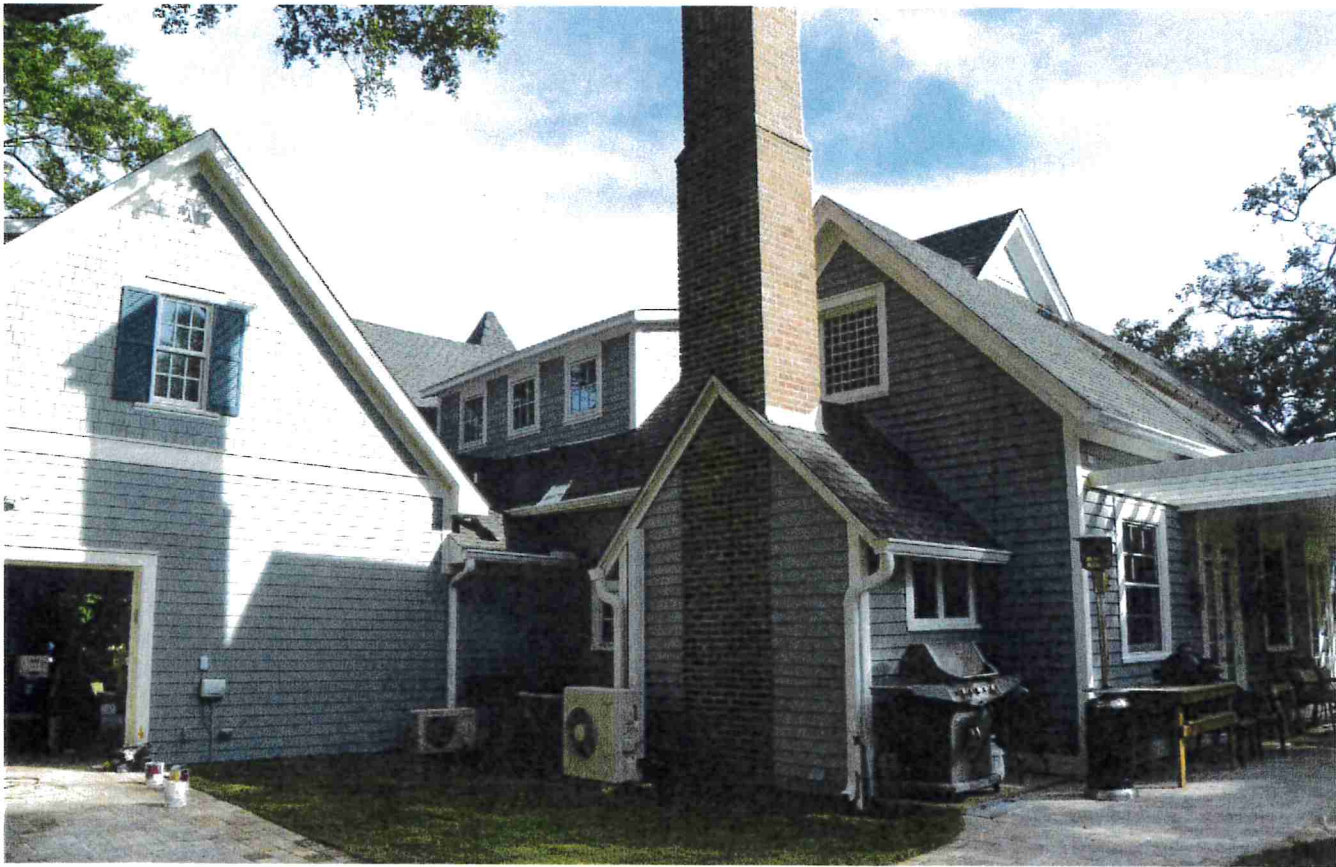
Photo 6 – Restored west façade (rear of the house). 10/28/16
