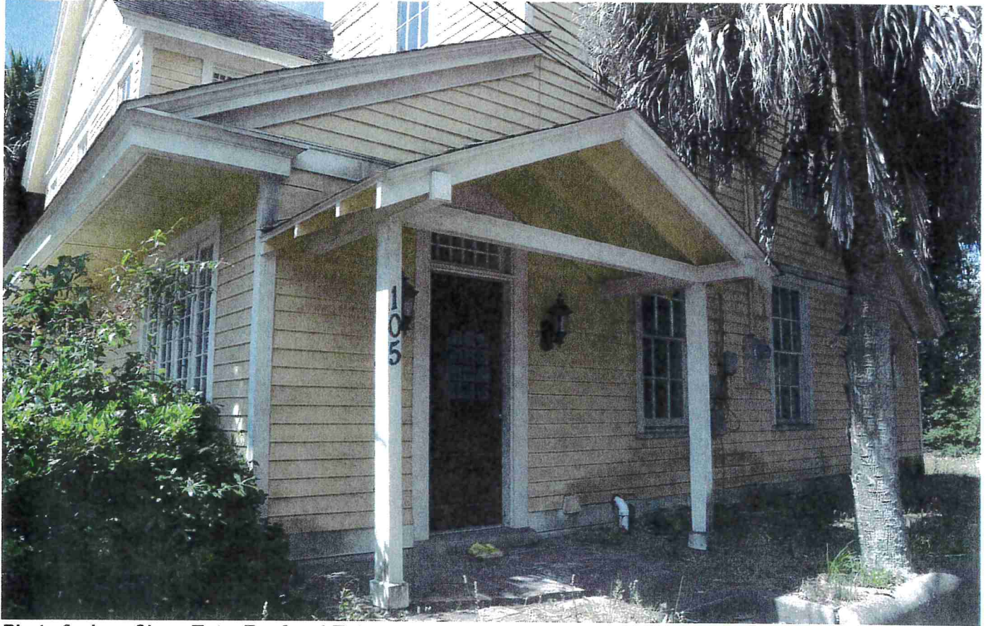
Photo 3 - Low Slope Entry Roof and Entry
