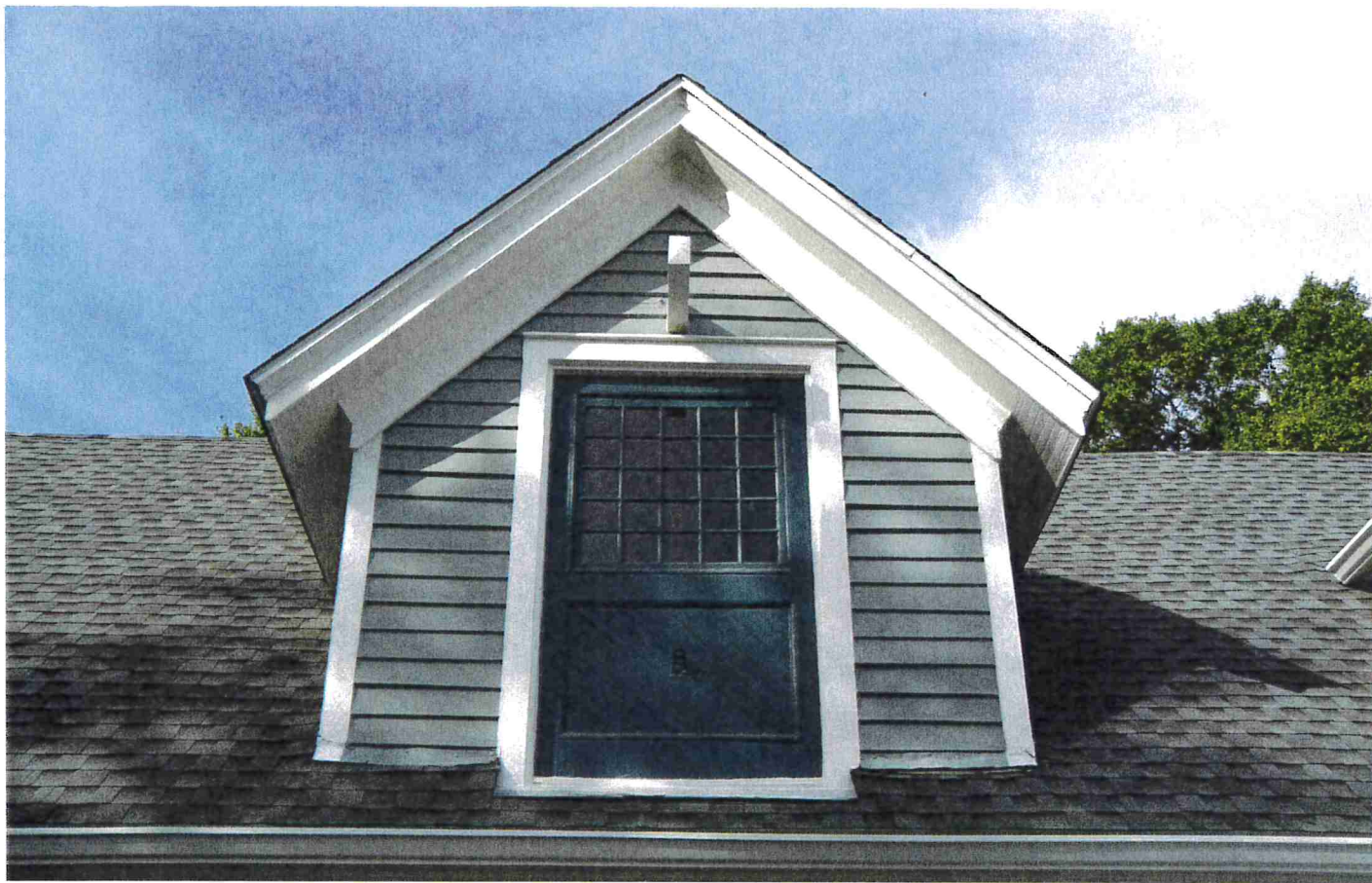
Photo 15 – Restored dormer above entry on east façade. 10/28/16
