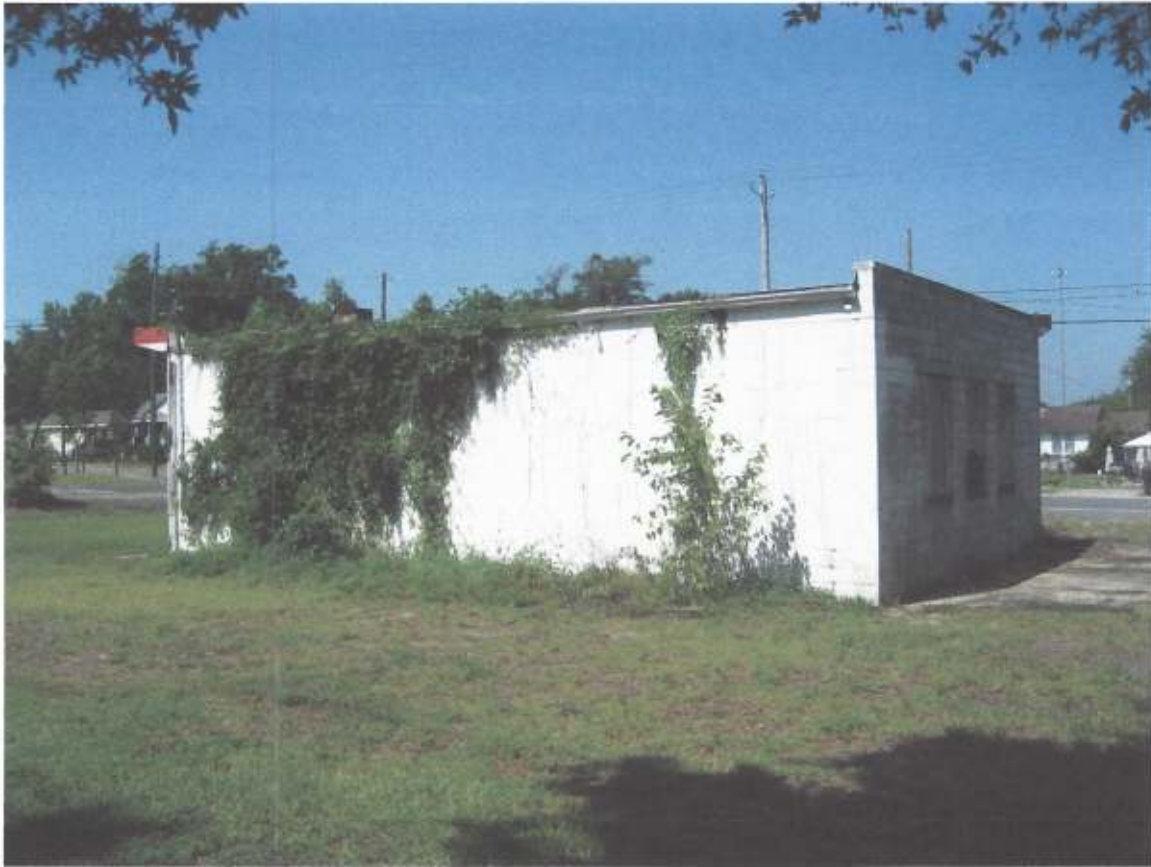
View of Rear of Subject Building
