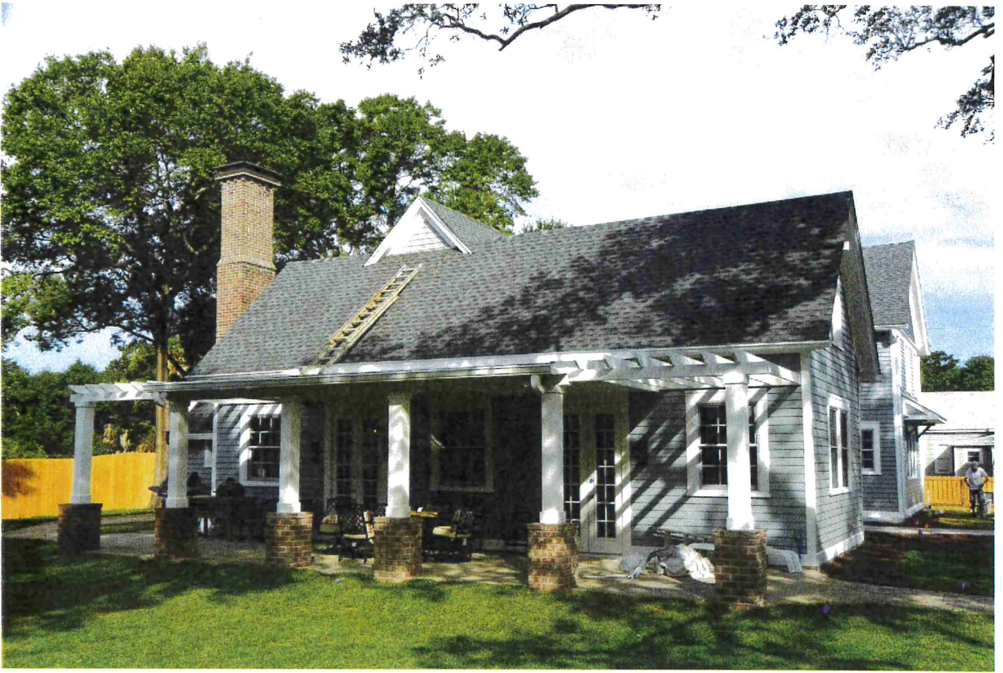
Photo 7 – Restored south façade (rear of the house). 10/28/16
