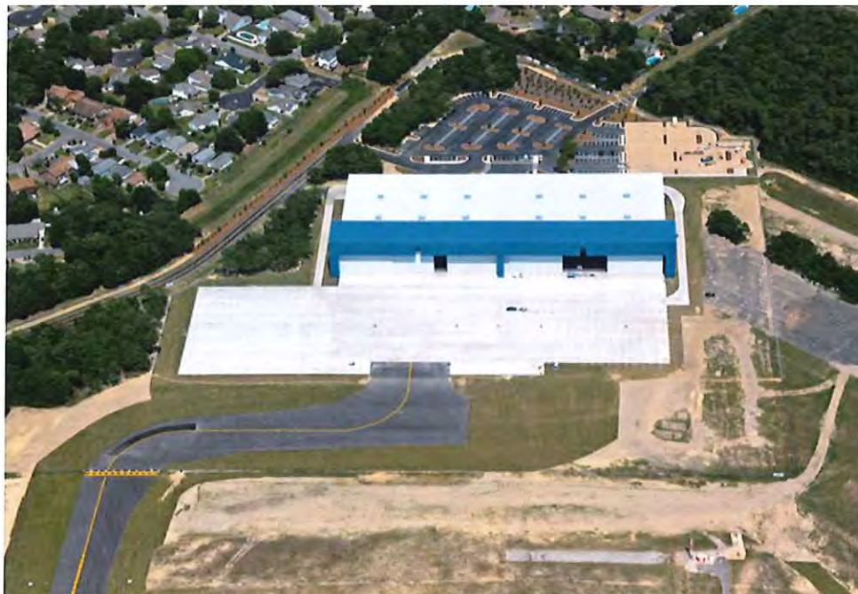
Figure 2 Hangar No. 1 on April 30, 2018
