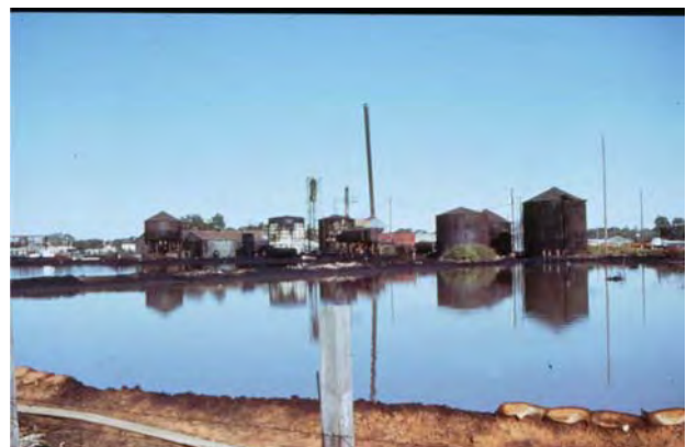
FIGURE 2-16. FORMER HOLDING PONDS AT THE ACW SITE
