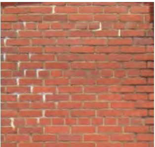
Existing Brick Facade
