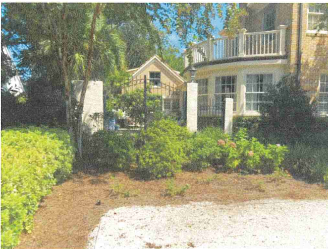
View of Front Left Side showing where existing parking Is for the property (gravel area) - Looking to where Proposed new Garage will be. The Circular Glass Sitting Room will be removed to allow for the New garage.
