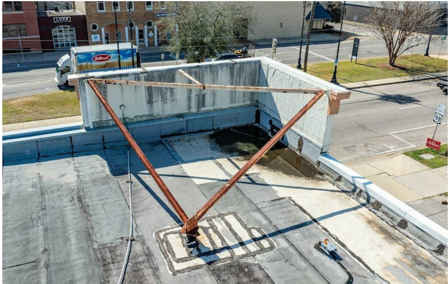
REAR OF EXISTING FACADE
