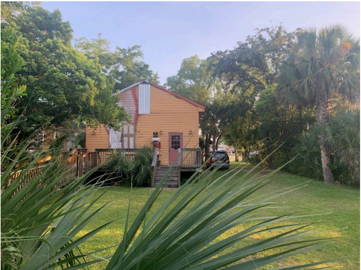
3 MID BACKYARD VIEW LOOKING NORTH
