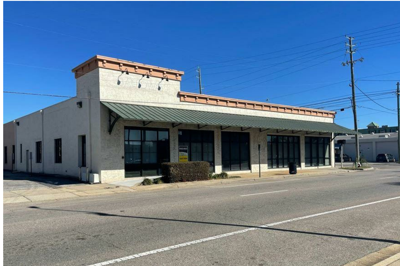
EXISTING FRONT FACING GARDEN
