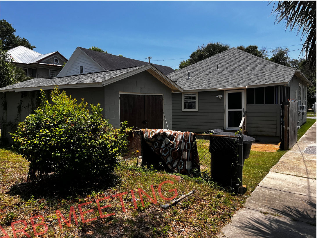
Rear Elevation of Property to the Right
