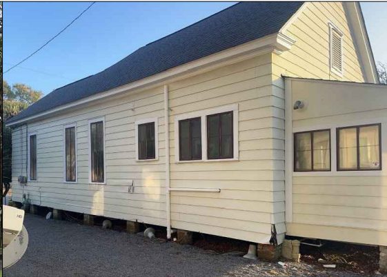
EXISTING BUILDING - SOUTHWEST VIEW
