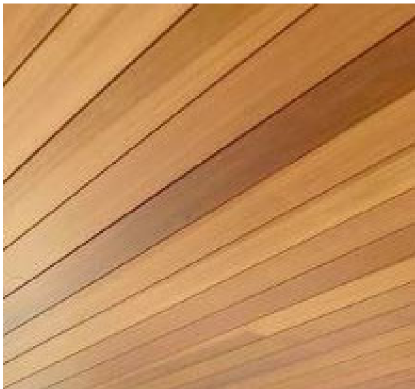
ENTRANCE AND TOWER SOFFITS
