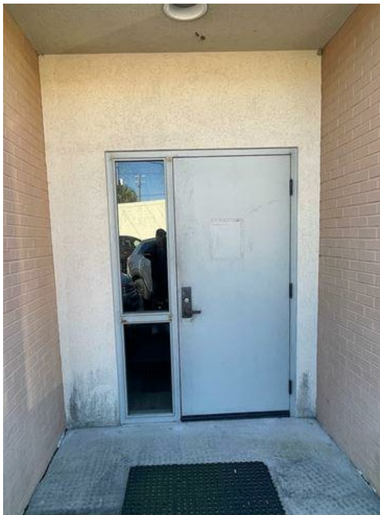
EXISTING REAR DOOR
