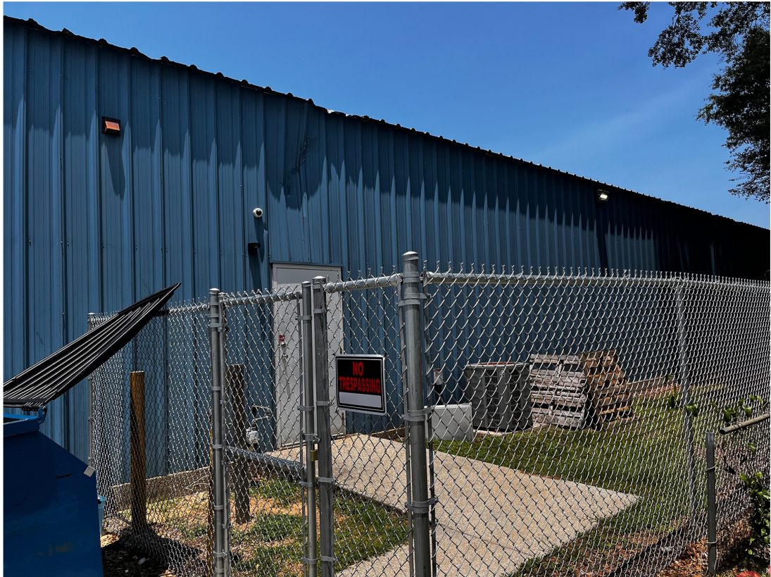
Rear Elevation of Property to the Left
