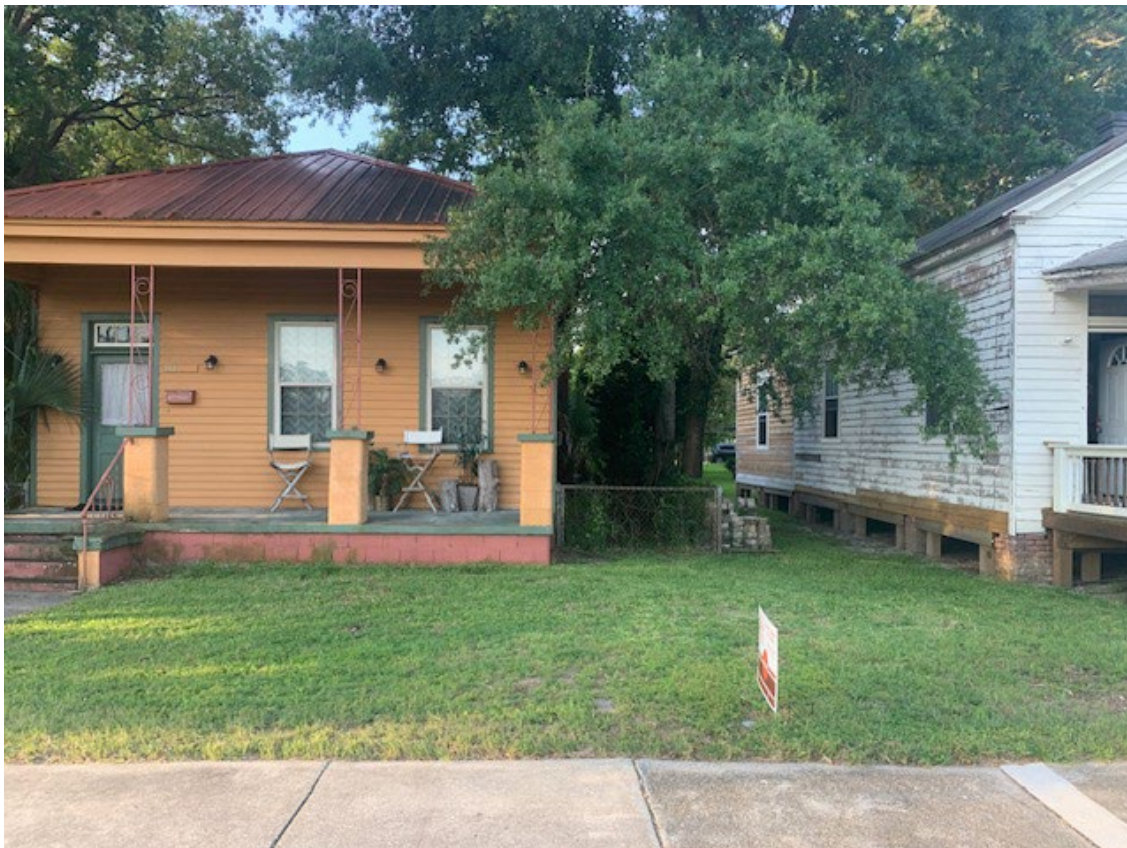
FRONT VIEW WITH WEST NEIGHBOR LOOKING SOUTH
