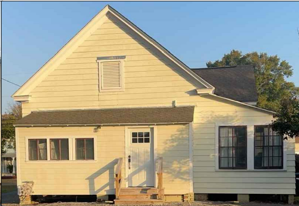
EXISTING BUILDING - SOUTH VIEW
