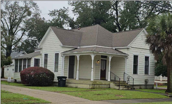
EXISTING BUILDING - NORTHEAST VIEW
