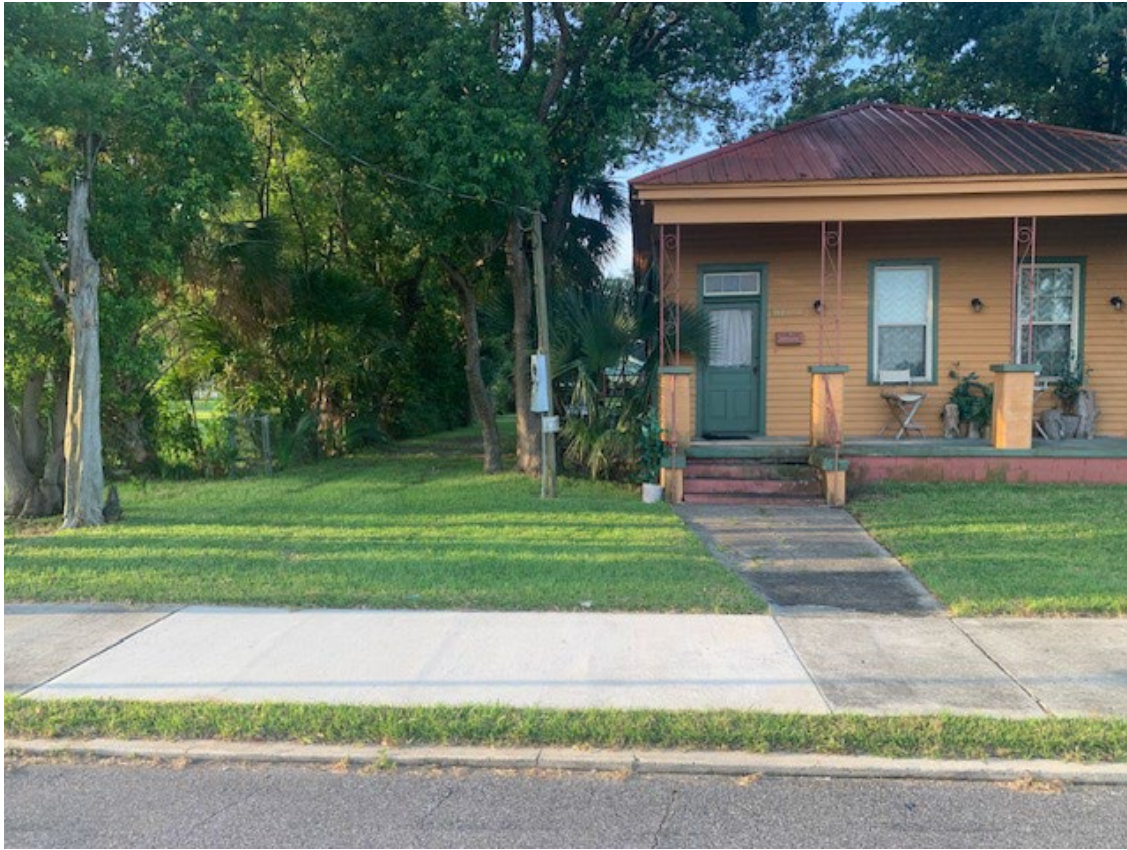
① FRONT VIEW LOOKING SOUTH
