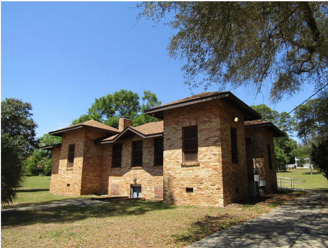
Figure 5-10. Southern elevation of the Boy Scout Building (8ES03838).
