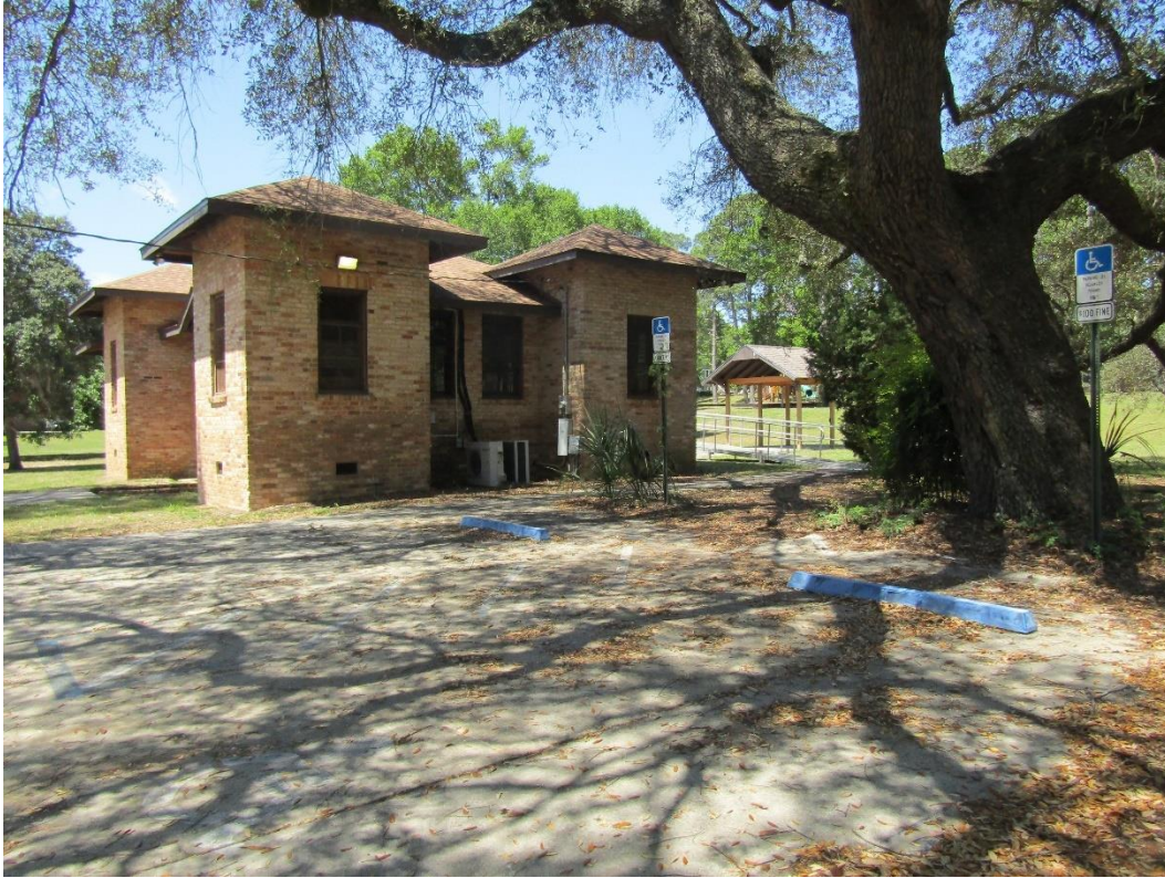
Figure 5-12. Miraflores Park parking lot with Boy Scout Building in background.
