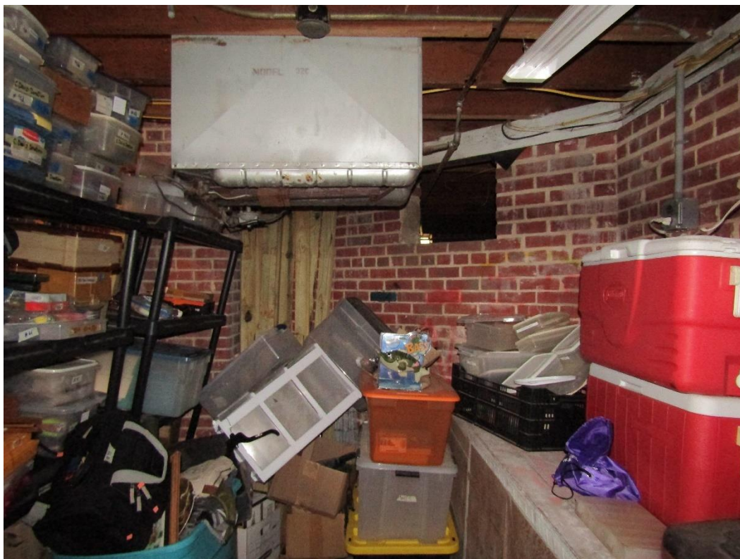
Figure 6-2. Interior of Boy Scout Building (8ES03838) raised basement.
