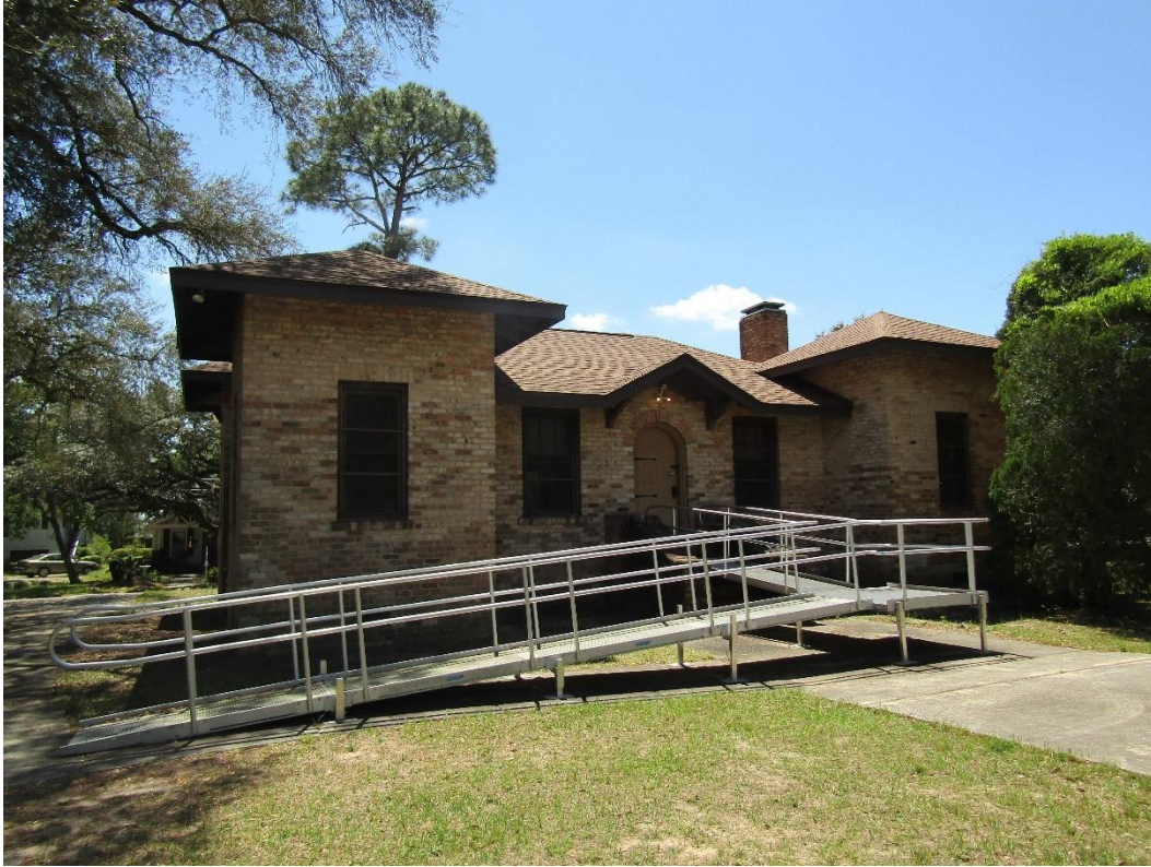
Figure 5-7. Primary (northern) elevation of the Boy Scout Building (8ES03838).
