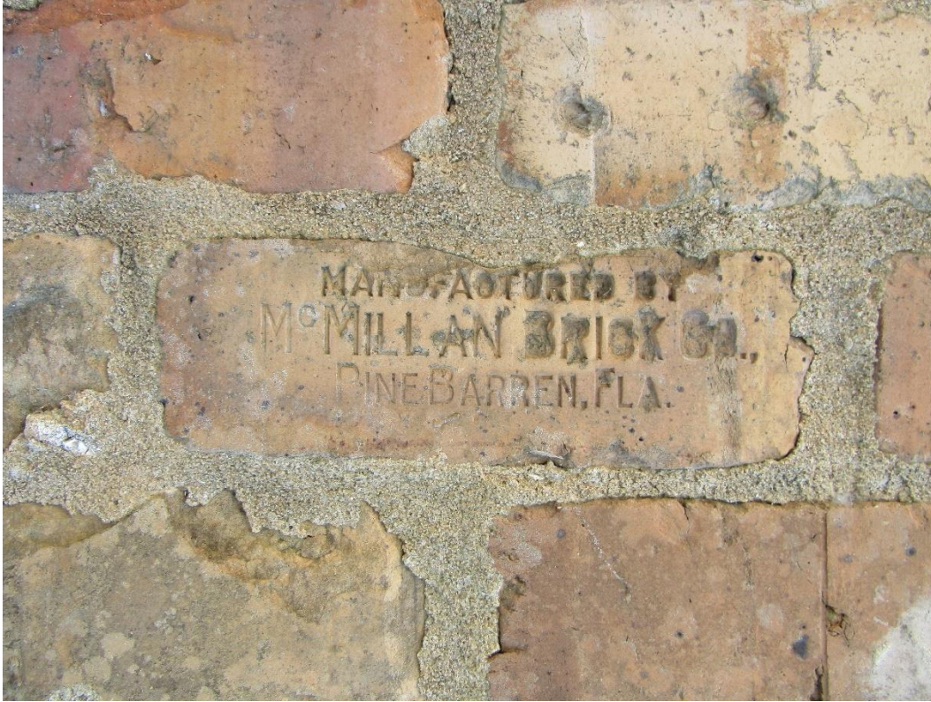
Figure 5-9. McMillan Brick Co. stamp found on Boy Scout Building exterior wall.
