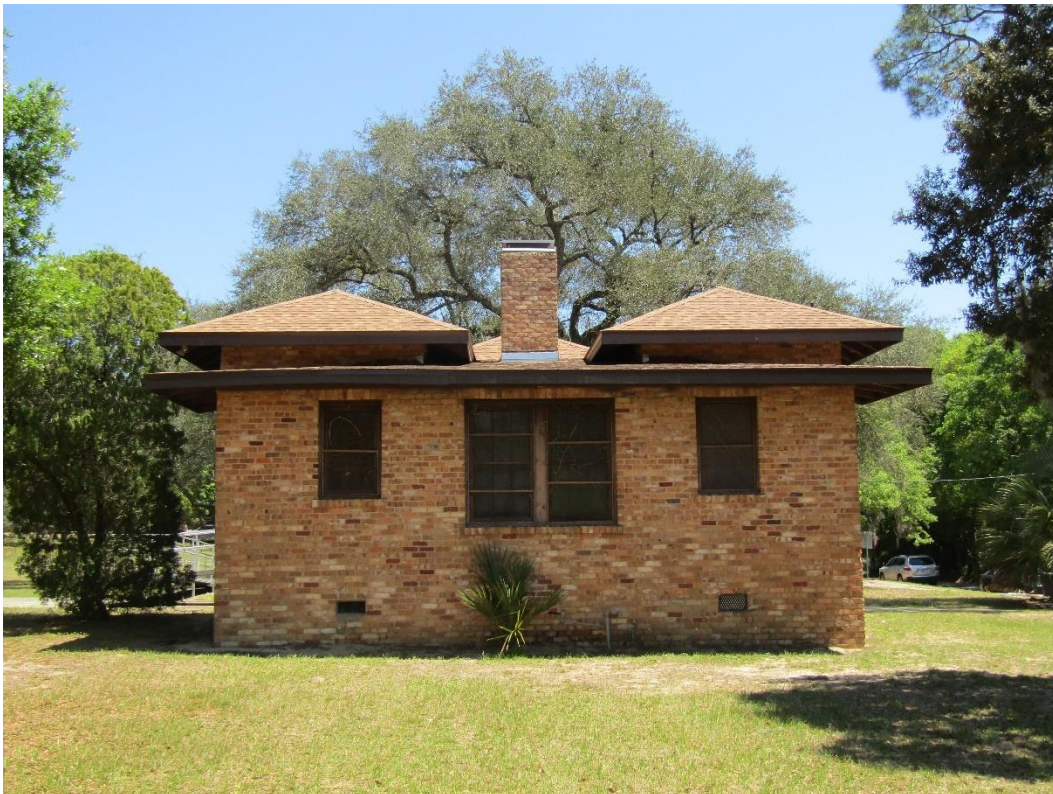
Figure 5-8. Western elevation of the Boy Scout Building (8ES03838).
