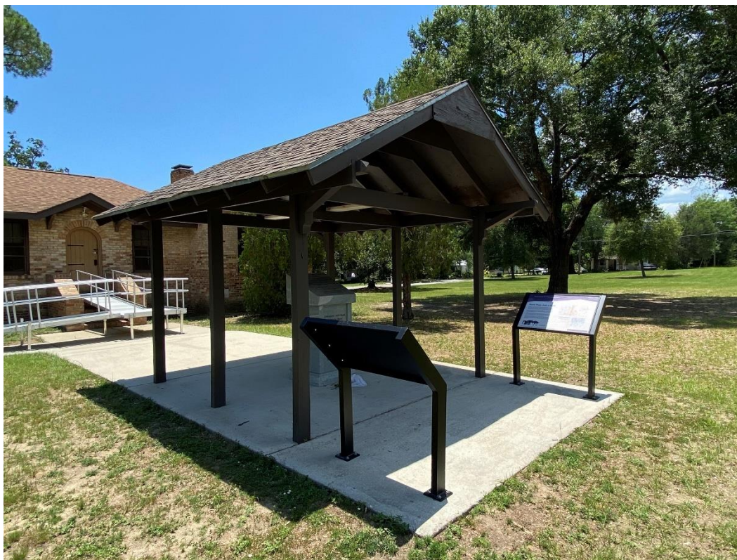
Figure 5-13. Miraflores Park pavilion, facing southwest.
