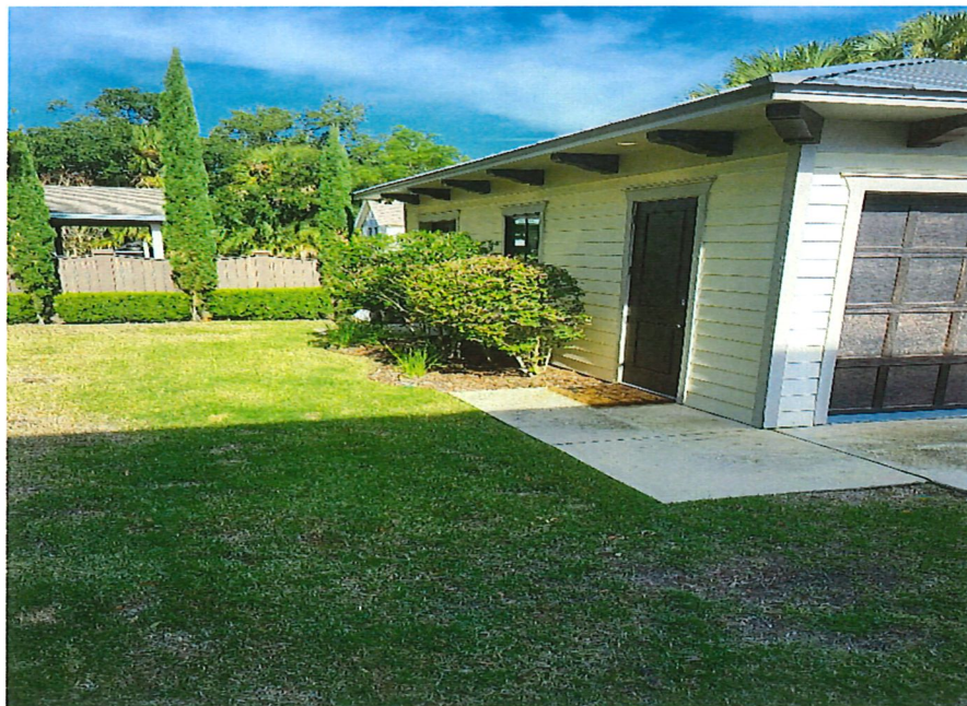
House looking towards back fence
