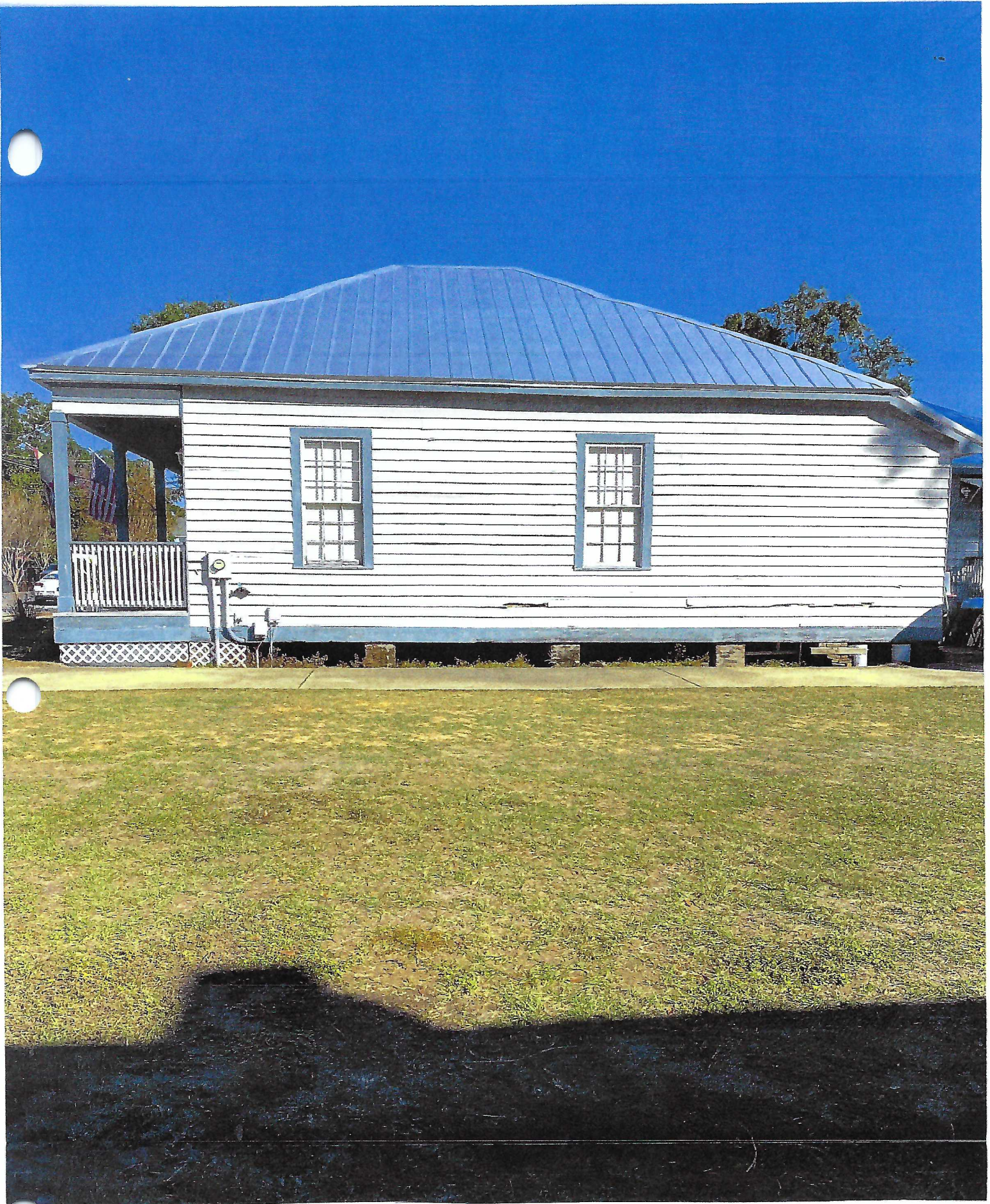
VIEW FROM EAST SIDE OF BUILDING
