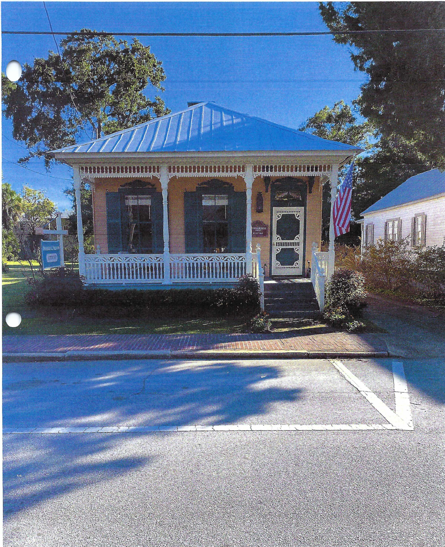
NORTH SIDE (FRONT) OF BUILDING
