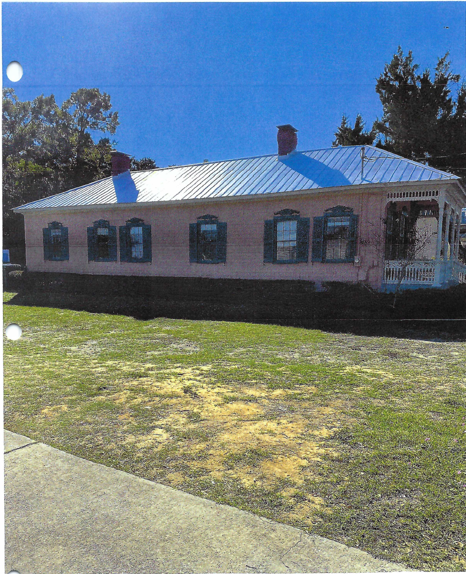
EAST SIDE OF BUILDING
