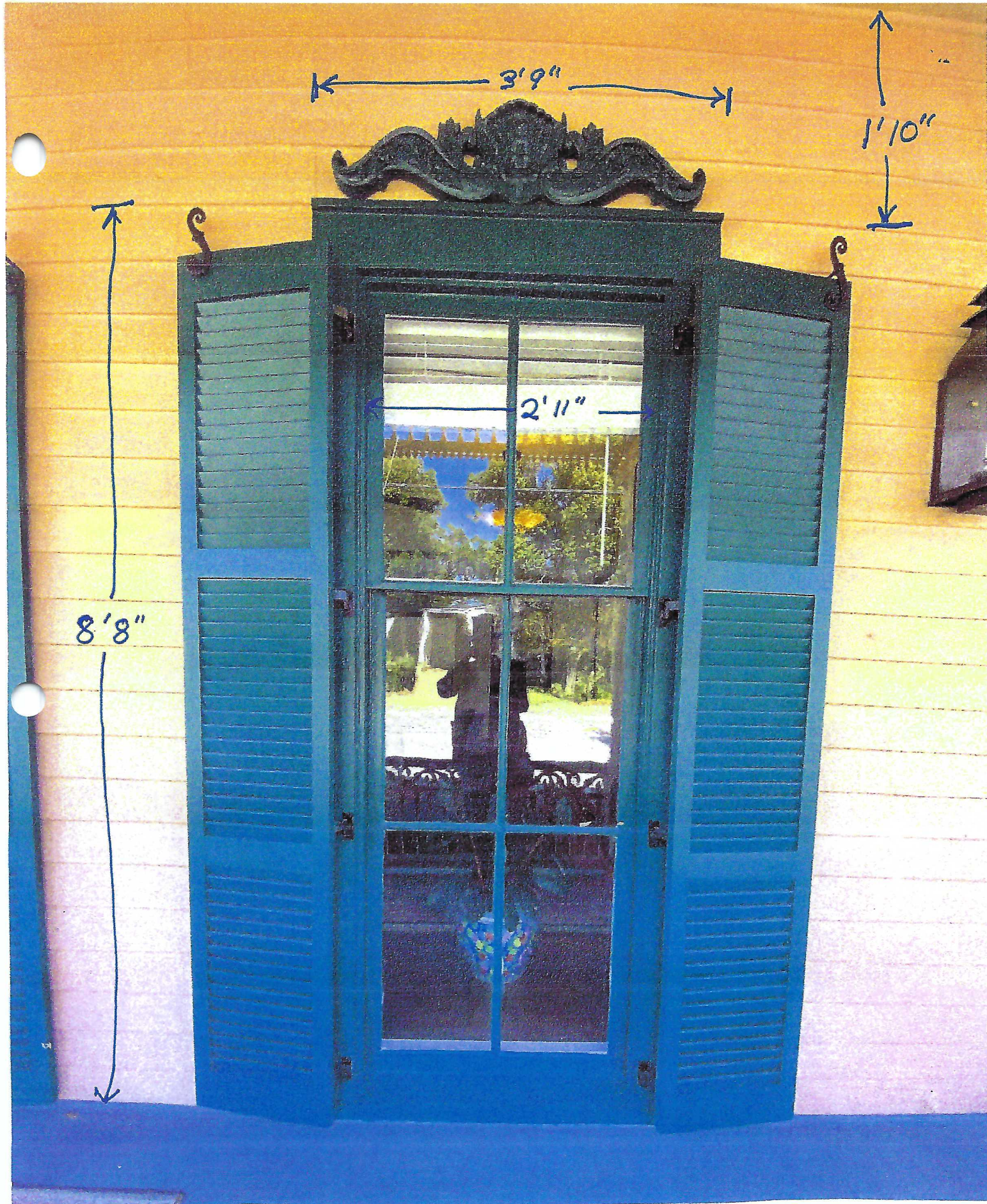
THERE ARE TWO OF THESE WINDOWS ON THE NORTH SIDE (FRONT) OF THE BUILDING
