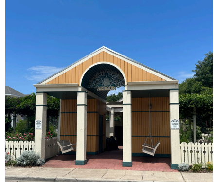
Shaded bus shelter in Aragon neighborhood
