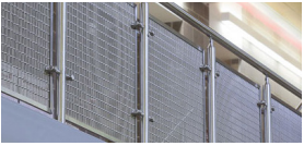
9. Metal Mesh Guardrail
