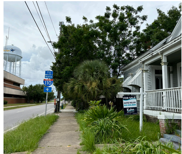
Sidewalk conditions along major Eastside corridors
