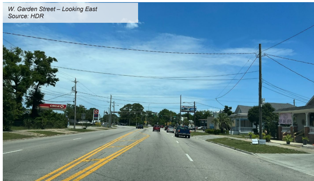
Figure 4 Westside – Arterial Road
