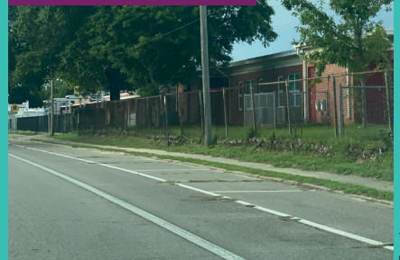
N Davis Highway
