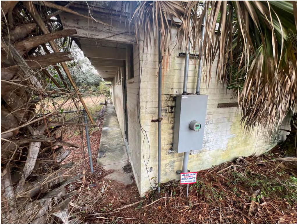
(5) View of northwest corner of the subject structure
