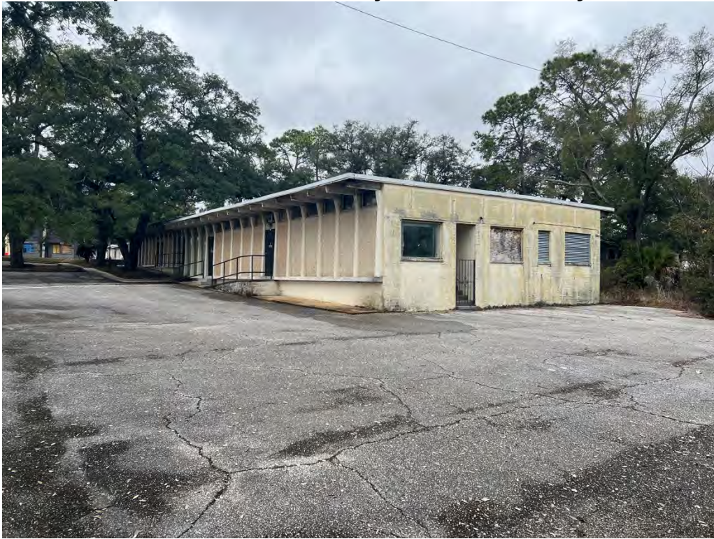
(1) View of southeast corner of the subject structure
