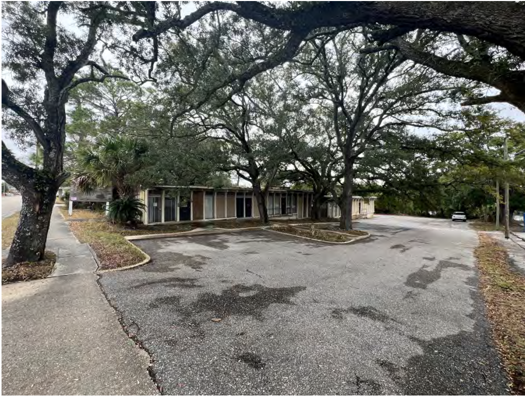
(3) View of southwest corner of the subject structure
