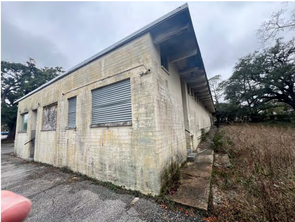
(2) View of northeast corner of the subject structure.
