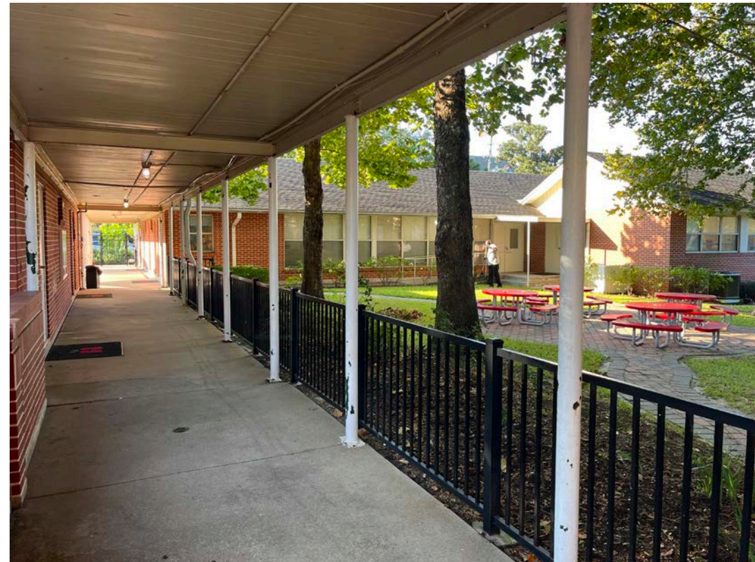
Photo of existing ceiling looking south. Various conduit to be consolidated into the new cornice, along with new paint on the ceiling and new lights.
