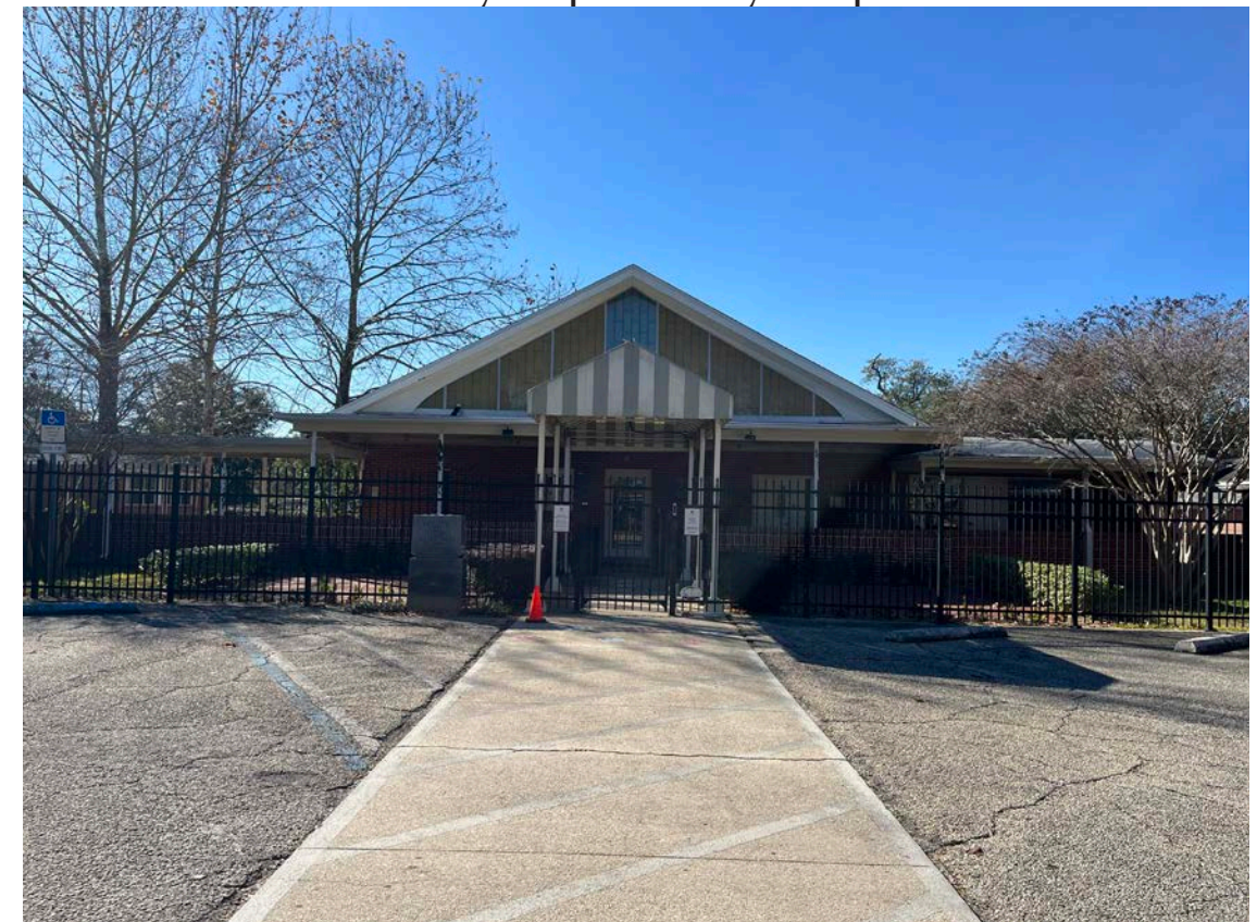
Photo of front entry. The asphalt and concrete will be replaced with pavers. The aluminum fence is to remain.
