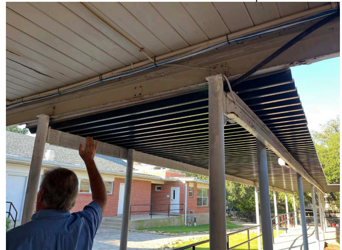
Photo showing underside of existing cross-corridor, as well as the various conduit to be cleaned up.
