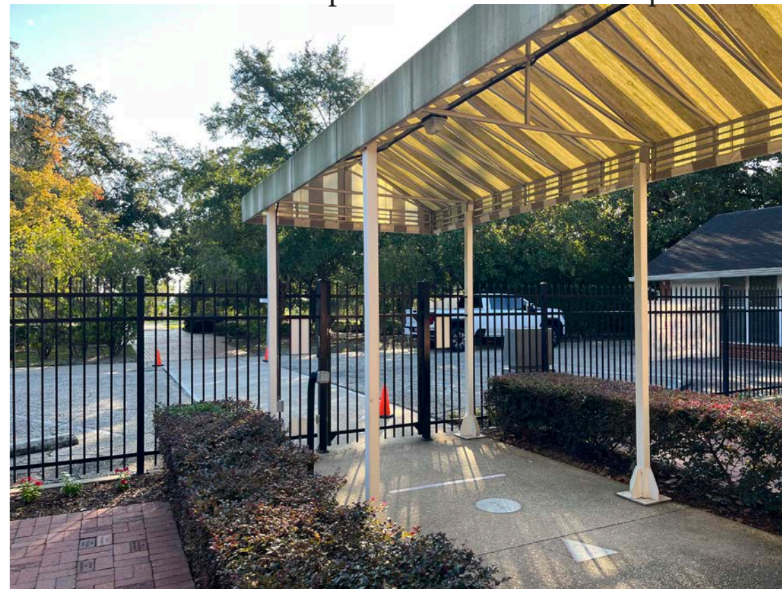
Photo of entry from inside. This area will be replaced with new pavers. The canopy will be removed and replaced with the new drop-off.
