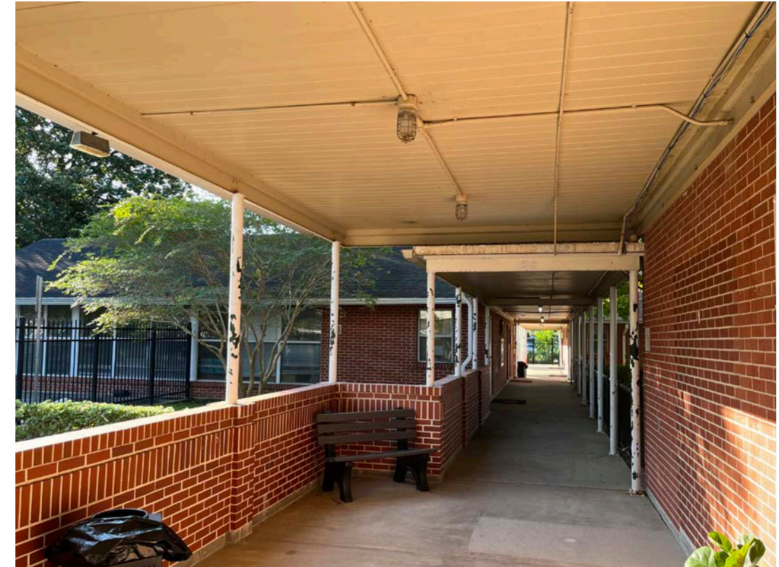
Photo of existing ceiling condition near check-in. New paint, light fixtures, and ceiling fans are proposed. New white square column covers will be installed on the existing pipe columns
