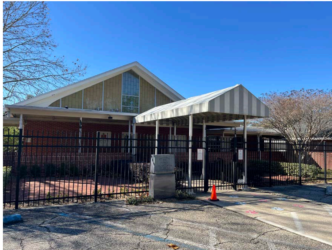
Photo of existing entry and canopy. This canopy will be removed and replaced with the new drop-off.
