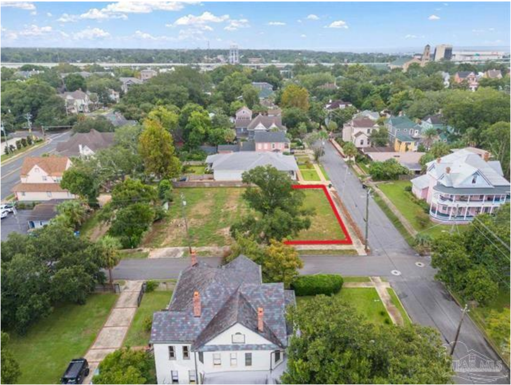
FROM WEST, LOOKING EAST – AERIAL
