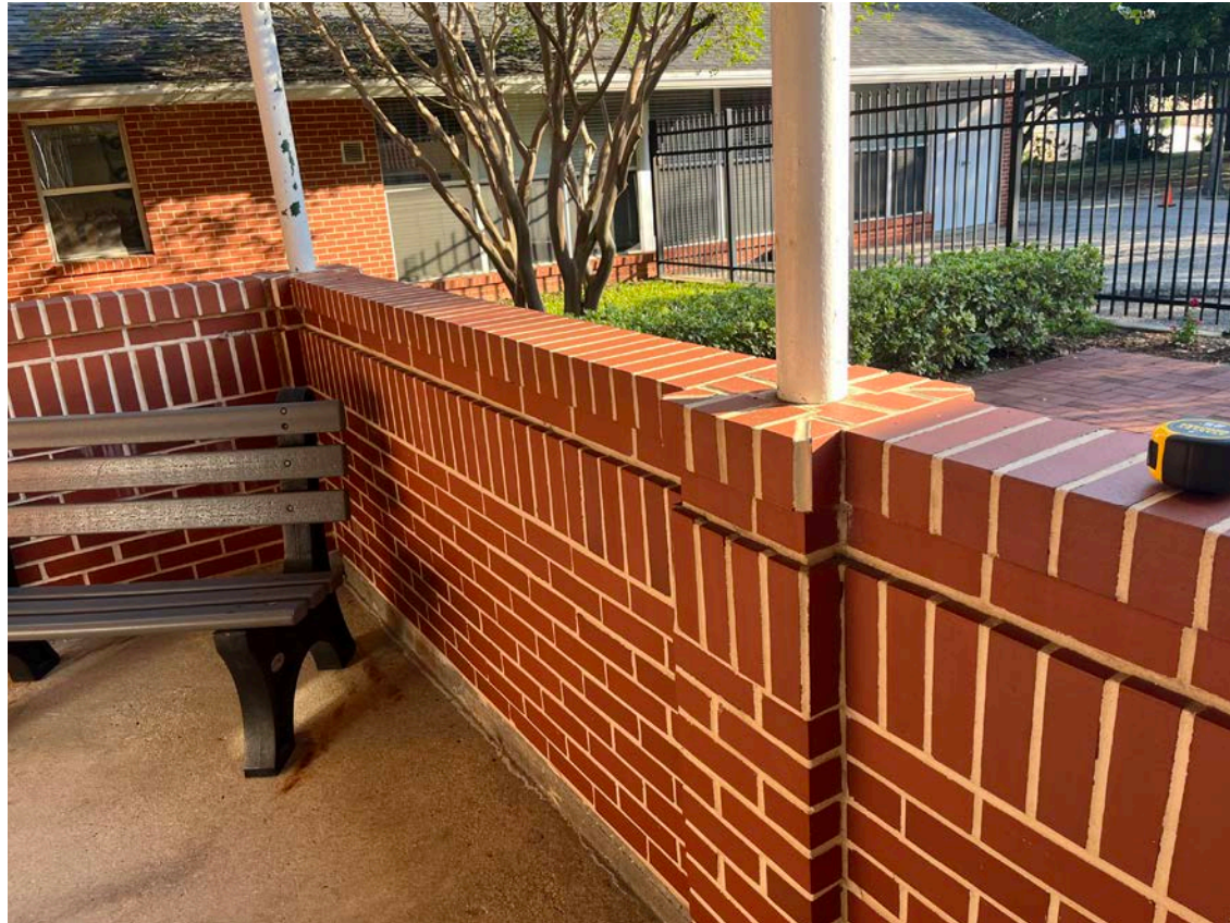
Photo of brick detailing at the existing low walls. The new columns on the south end are to match. Pipe columns to receive square column wrap.
