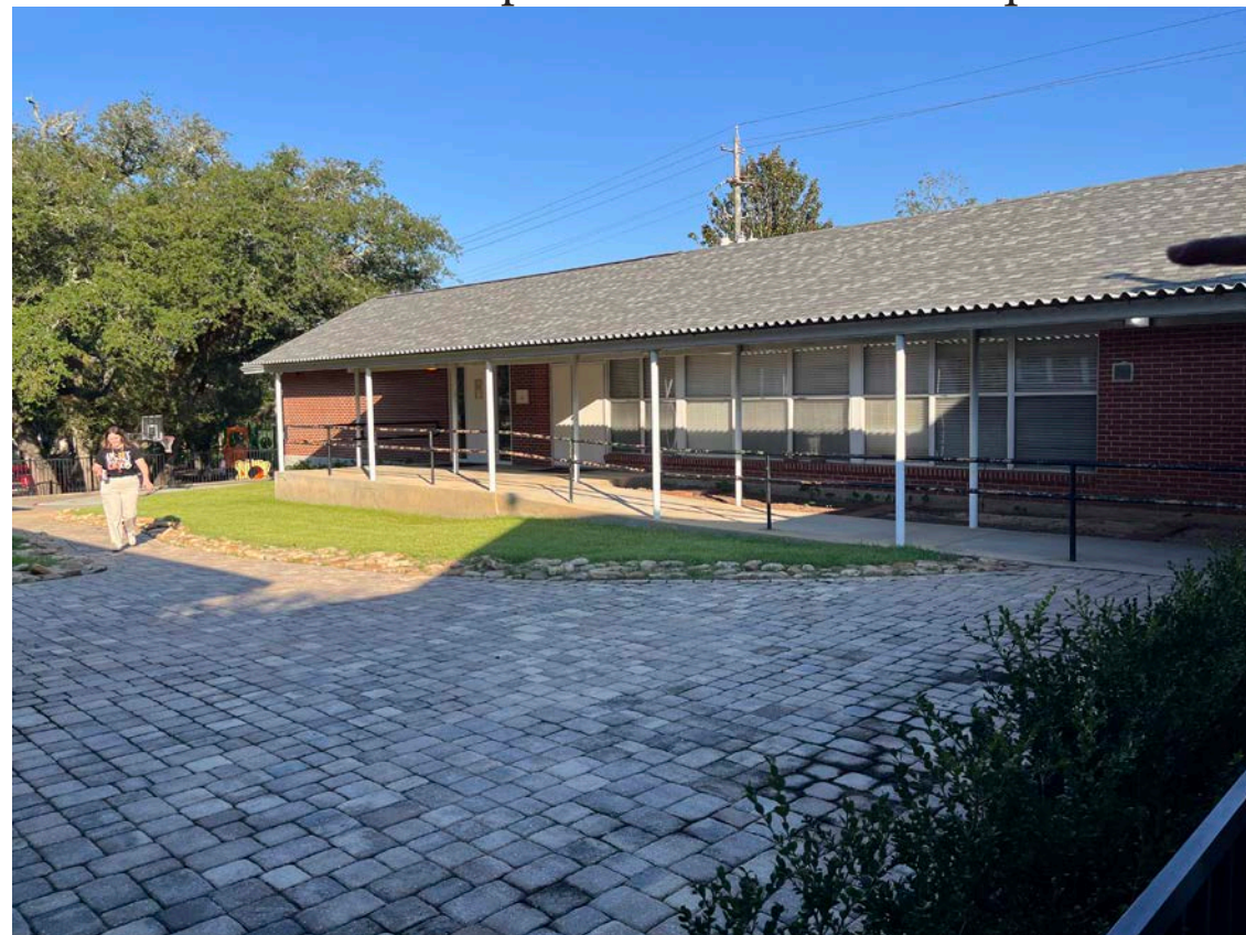
Photo showing existing cross-corridor. New T&G ceiling and TPO roof will be installed to match the existing corridor.
