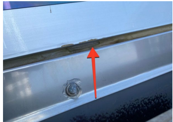
Failing sealant
